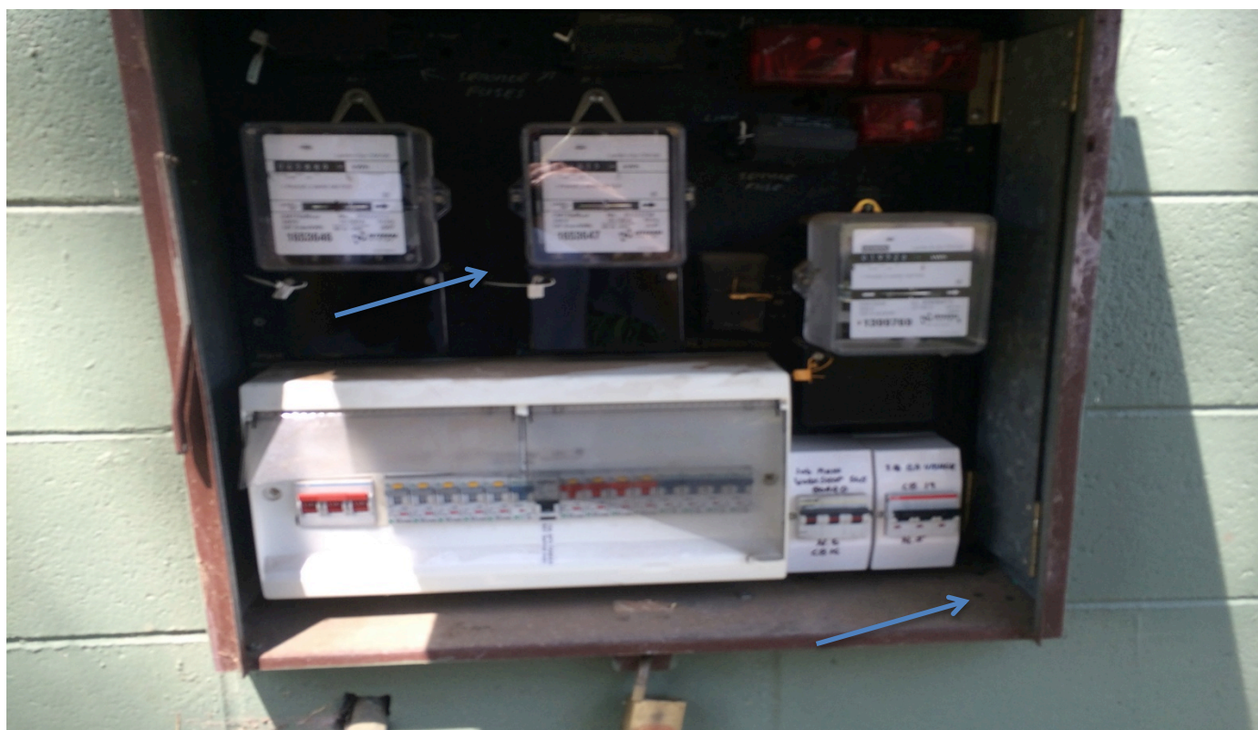
Photo 131: Electrical backing board and debris containing asbestos on the north-eastern perimeter of the Winmalee Rural Fire Service Bushfire Brigade.
