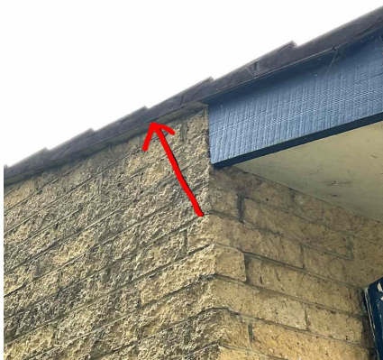
External, GF, Exterior, Throughout roof perimeter, Below Roof Tiles on Edge Soffit - Fibre Cement, Chrysotile, B17372-S03
