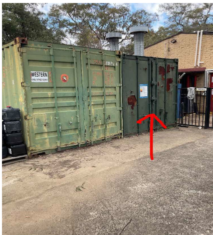
External, GF, Shipping Container, All surfaces - Green (Dark) - Topcoat, Lead Detected (%0.54 w/w), 17372S03
