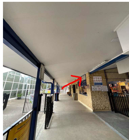
Internal, GF, Kiosk, Infill Panel Roller Door - Fibre Cement, Assumed Positive, Similar to B17372-S08 - Assumed Chrysotile
