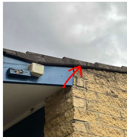
External, GF, Exterior, Throughout roof perimeter, Below Roof Tiles on Edge Soffit - Fibre Cement, Chrysotile, B17372-S03
