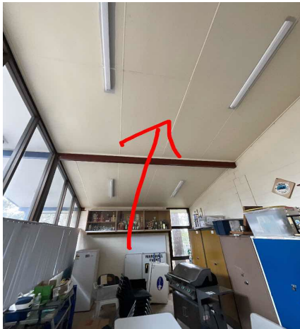
Internal, GF, Clubroom, Fibre Cement Ceiling - Fibre Cement, Assumed Positive, Similar to B17372- S10 - Assumed Chrysotile
