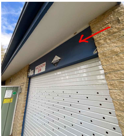
External, GF, Exterior, South East, South East elevation, Infill Above Roller Door - Fibre Cement, Chrysotile, B17372-S01
