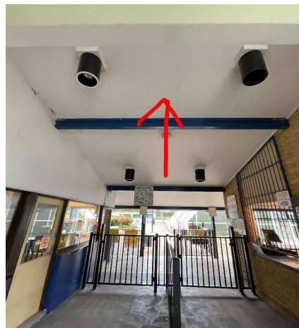
External, GF, Exterior, South East, Entrance ceiling lining - Fibre Cement, Assumed Positive, Same to B17372-S02 - Assumed Chrysotile
