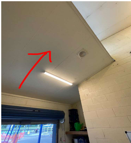
Internal, GF, Store Room 3, Ceiling - Fibre Cement, Chrysotile, B17372-S10
