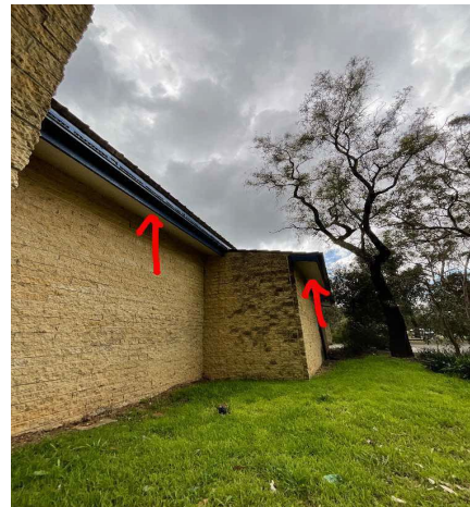
External, GF, Exterior, South East, South East elevation, Eaves - Fibre Cement, Chrysotile, B17372-S02
