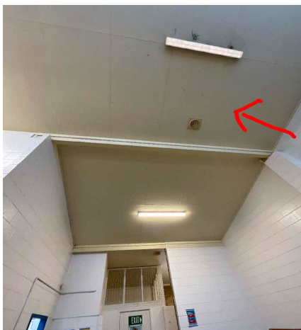
Internal, GF, Female Amenities, Ceiling - Fibre Cement, Assumed Positive, Similar to B17372-S10 - Assumed Chrysotile
