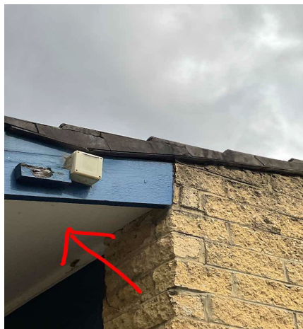
External, GF, Exterior, South East, Eave lining above infill over roller door - Fibre Cement, Assumed Positive, Same to B17372-S02 - Assumed Chrysotile
