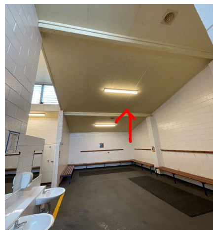
Internal, GF, Male Amenities, Ceiling - Fibre Cement, Assumed Positive, Similar to B17372-S10 - Assumed Chrysotile
