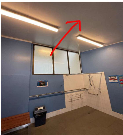
Internal, GF, Wheelchair Accessible Toilet, Ceiling - Fibre Cement, Assumed Positive, Similar to B17372 - S10 - Assumed Chrysotile
