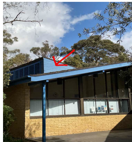
External, Roof, Gable, South East, Fascia - Blue - Topcoat, Lead Detected (%0.1 w/w), 17372S01
