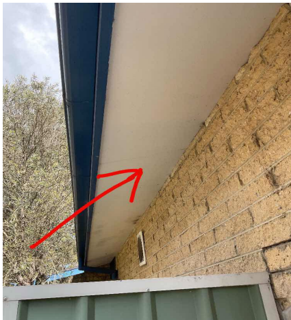
External, GF, Exterior, South East, South East elevation, Eaves - Fibre Cement, Chrysotile, B17372-S02
