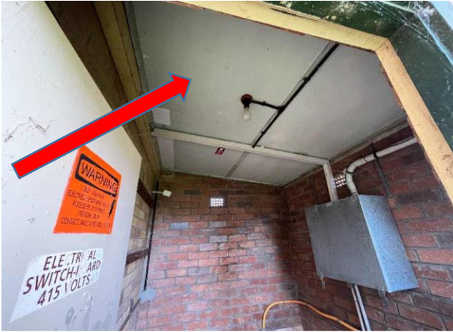
Internal, GF, Electrical board room (western side), Ceiling - Fibre Cement Sheet, Chrysotile & Amosite Asbestos detected, Previously sampled, similar to B17399S02
