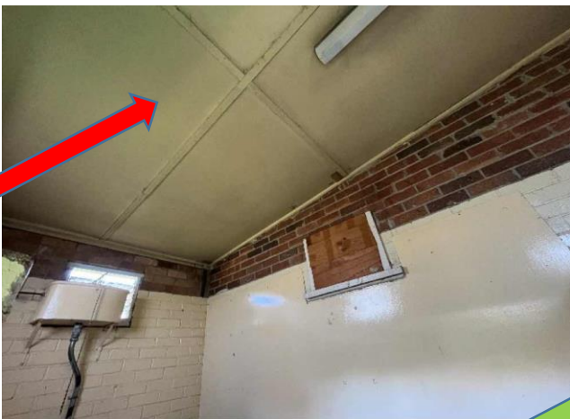
Internal, GF, Men's toilet, Ceiling - Fibre Cement Sheet, Chrysotile & Amosite Asbestos detected, Previously sampled, similar to B17399S02
