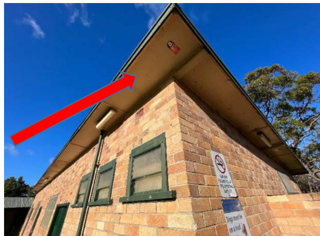
External, GF, Exterior, Eaves, Perimeter of main amenities - Fibre Cement Sheet, Chrysotile & Amosite Asbestos detected, Previously sampled B17399S01
