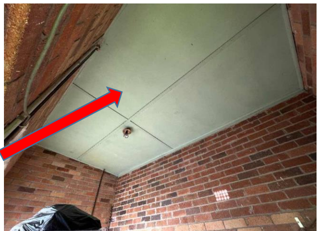
Internal, GF, South West Room (kitchen), Ceiling - Fibre Cement Sheet, Chrysotile & Amosite Asbestos Detected, Previously sampled B17399S02
