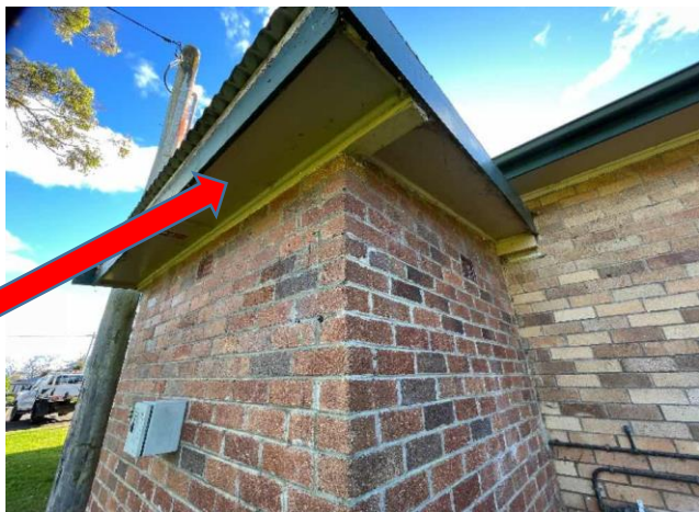
External, GF, Exterior, West, Eaves, Perimeter of electrical room - Fibre Cement Sheet, Chrysotile & Amosite Asbestos detected, Previously sampled, same as B17399S01
