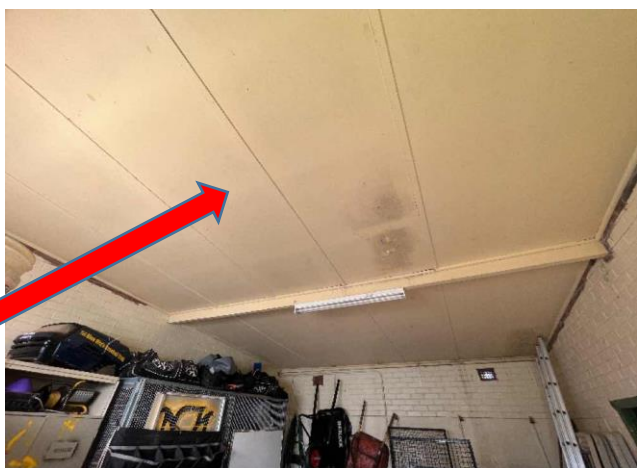
Internal, GF, Central (north) storeroom (Cricket storeroom), Ceiling -
