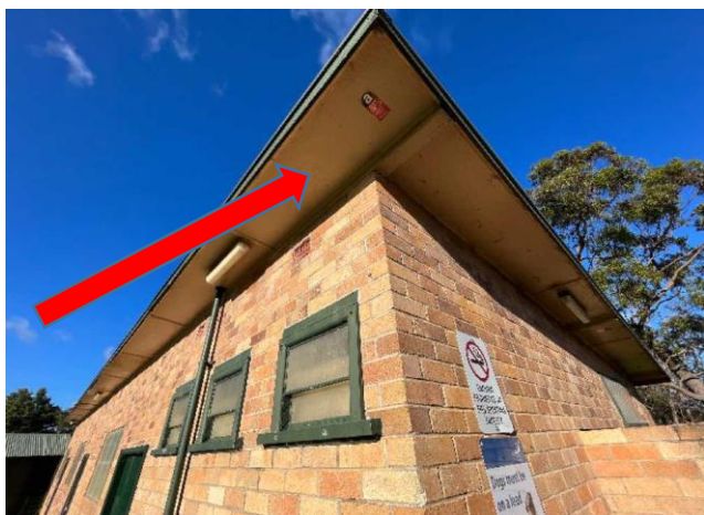
External, GF, Exterior, External cream paint system - Cream - Topcoat, Lead Detected (1.0%w/w), Previously sampled 17399-S05
