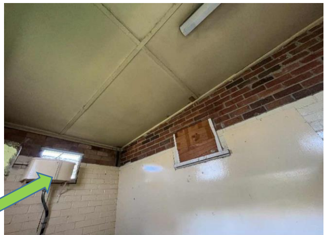
Internal, GF, Men's toilet, Mens urinal cistern - Moulded Fibre Cement, No Asbestos Detected, Previously sampled B17399S03
