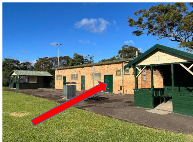
External, GF, Exterior, External green paint system - Green - Topcoat, Lead detected, 437871-LP01
