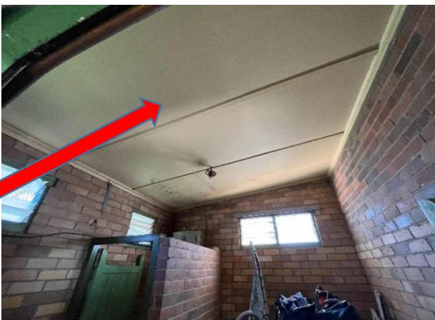
Internal, GF, North west corner storeroom/toilet, Ceiling - Fibre Cement Sheet, Chrysotile & Amosite Asbestos detected, Previously sampled, similar to B17399S02
