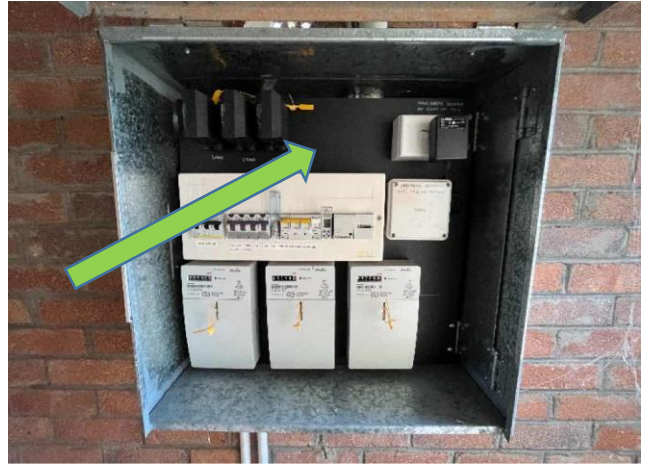
Internal, GF, Electrical board room (western side), West, Wall - Electrical backing board, No Asbestos Detected, Visually identified
