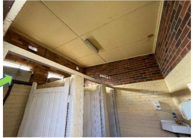
Internal, GF, Women's toilet, Women's toilet cistern - Moulded Fibre Cement, No Asbestos Detected, Previously sampled B17399-S7
