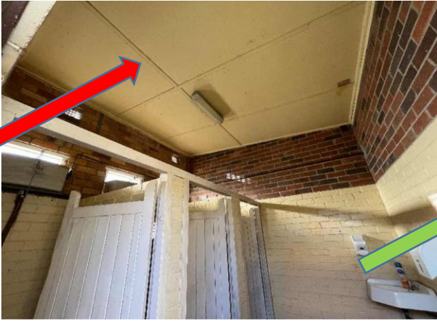
Internal, GF, Women's toilet, Ceiling - Fibre Cement Sheet, Chrysotile & Amosite Asbestos detected, Previously sampled, similar to B17399S02
