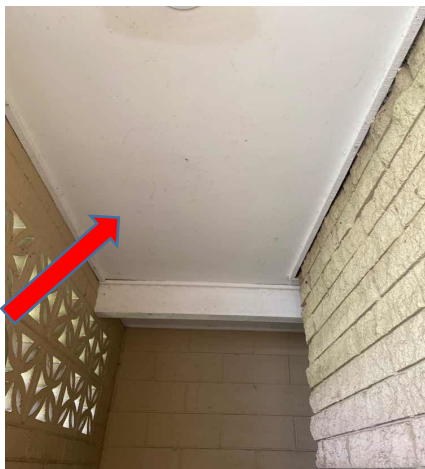
Internal, GF, Female Toilet, Ceiling - Fibre Cement, Chrysotile and AMOSITE, B17397-S05
