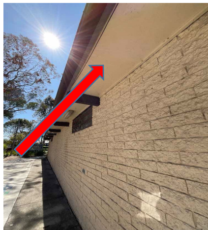
External, GF, Exterior (west) Clubhouse, Eaves - Fibre Cement Sheeting, Chrysotile Asbestos, B17397S01
