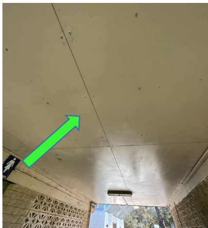
External, GF, Exterior central walkway, Ceiling - Fibre cement, No Asbestos identified, B17397-S02
