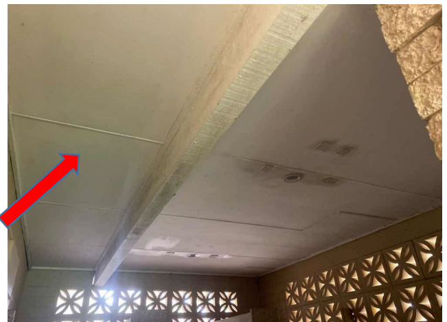
Internal, GF, Female Toilet, Ceiling - Fibre Cement, Chrysotile and AMOSITE, B17397-S05
