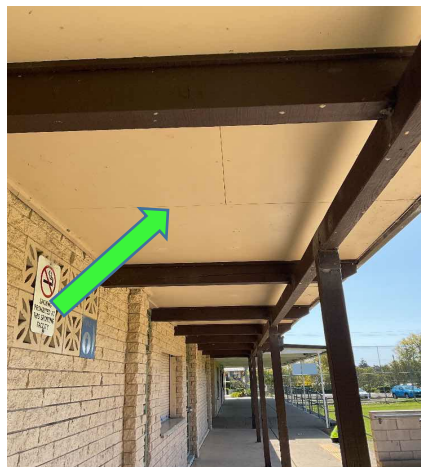
External, GF, Exterior (east) Amenities, Ceiling - Fibre cement, No Asbestos identified, B1737-S03
