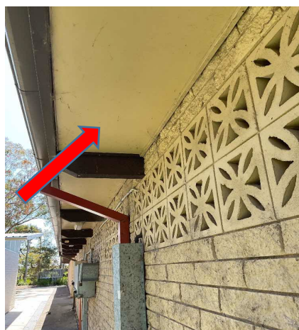
External, GF, Exterior (west) Amenities, Eave Linings to West Amenities End - Fibre cement, Chrysotile, B17397-S01
