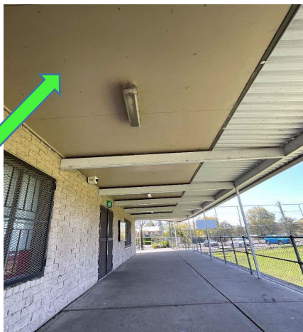
External, GF, Exterior (east) Clubhouse, Ceiling lining - Fibre Cement Sheeting, No Asbestos Detected, Similar to B17397-S03
