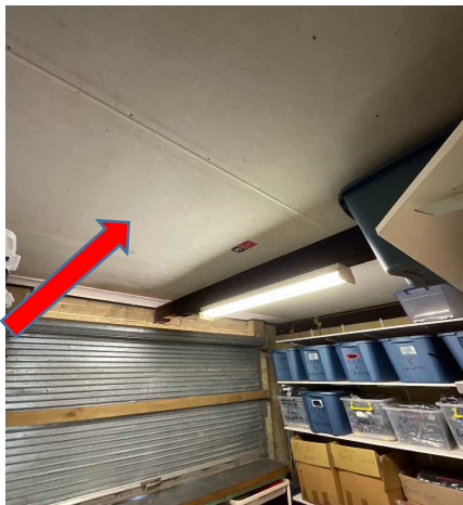
Internal, GF, Storeroom, Ceiling - Fibre Cement, Chrysotile and AMOSITE, B17397-S05.4
