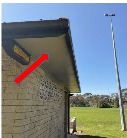
External, GF, Exterior (south) Amenities, South, Eave linings to south amenities end - Fibre Cement, Chrysotile, B17397-S04
