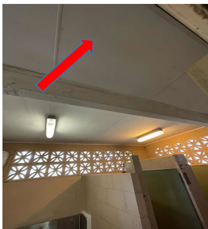
Internal, GF, Male Toilet & Changeroom, Ceiling - Fibre Cement, Chrysotile and AMOSITE, B17397-S05.1
