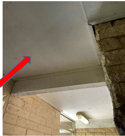
Internal, GF, Female Changeroom, Ceiling - Fibre Cement, Chrysotile and AMOSITE, B17397-S05.3
