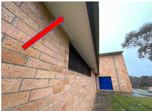
External, GF, Adjacent Kids Kingdom, Eave Linings - Fibre Board, Chrysotile, B17382-S28
