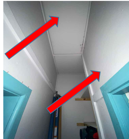
Internal, GF, Kids Kingdom Kitchen Foyer/Storage Room, Walls and Ceiling - Fibre Board, Chrysotile, B17382-S23
