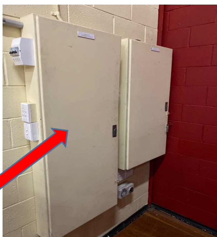
Internal, GF, Kids Kingdom Electrical Switchboard, Electrical Meter Board - Note: Electrical Cabinets were locked Therefore Could Not Be Accessed - Fibre Board, Assumed Positive, Assumed positive
