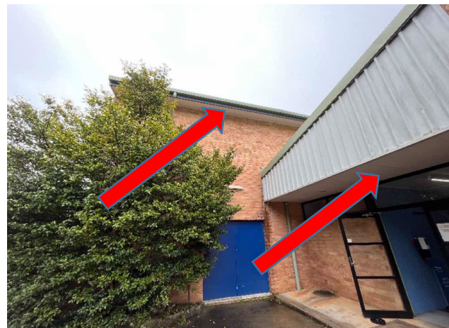
External, GF, Exterior, External Eaves Adjacent Band Hall - Fibreboard, Assumed Positive, Similar to B17382-S28 - Assumed Chrysotile
