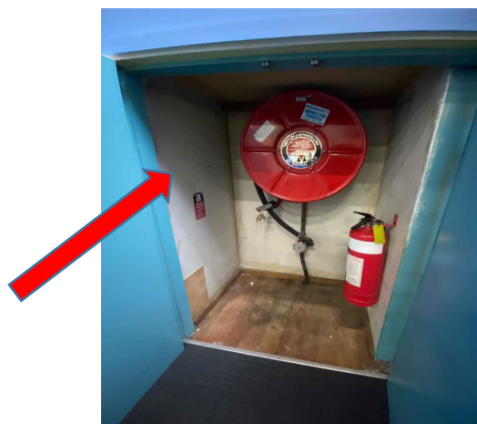
Internal, GF, Kids Kingdom Fire Hydrant Cupboard, Fire Hydrant Cupboard Lining Fibre Board - Fibre Board, Chrysotile, B17382-S20
