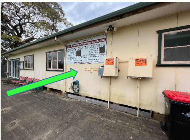
External, GF, Exterior, South, Wall cladding - Fibre Cement Sheet, No Asbestos Detected, B17380S28
