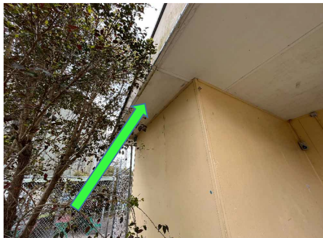
External, GF, Exterior, East, Eave - Fibre Cement Sheet, No Asbestos Detected, B17380S24
