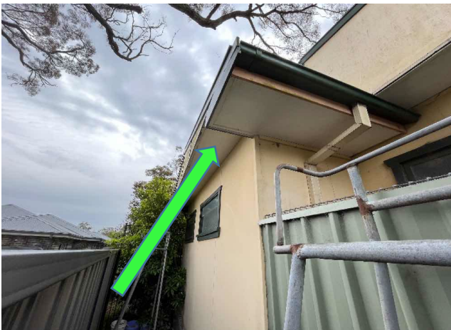
External, GF, Exterior, South West, Eaves adjacent tennis club amenities - Fibre Cement Sheet, No Asbestos Detected, B17380S31
