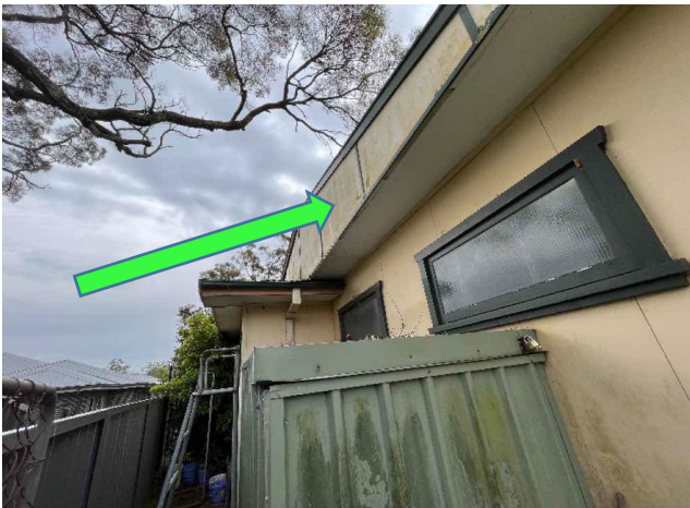
External, GF, Exterior, West, Gable end - Fibre Cement Sheet, No Asbestos Detected, B17380S23
