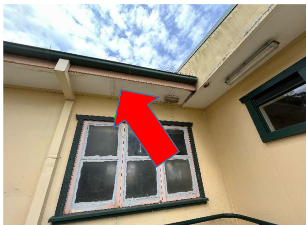
External, GF, Exterior, North, Eave lining to Approx 1.2m, Above Wheelchair Ramp - Fibre Cement Sheet, Chrysotile Asbestos, B17380S02 & B17380S32
