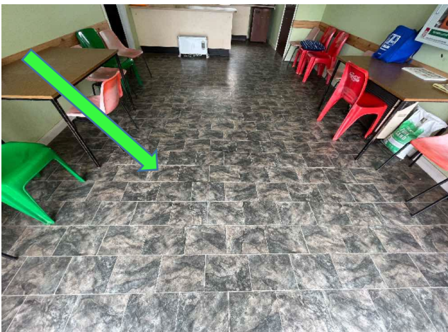
Internal, GF, Tennis Club Room, Kitchen Kickboard - Vinyl Sheet Adjacent Cupboards - Vinyl Sheet, No Asbestos identified, B17380S13
