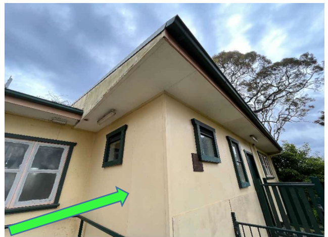
External, GF, Exterior, North, Walls and eaves adjacent wheelchair access - Fibre Cement Sheet, No Asbestos Detected, B17380S25 & B17380S31
