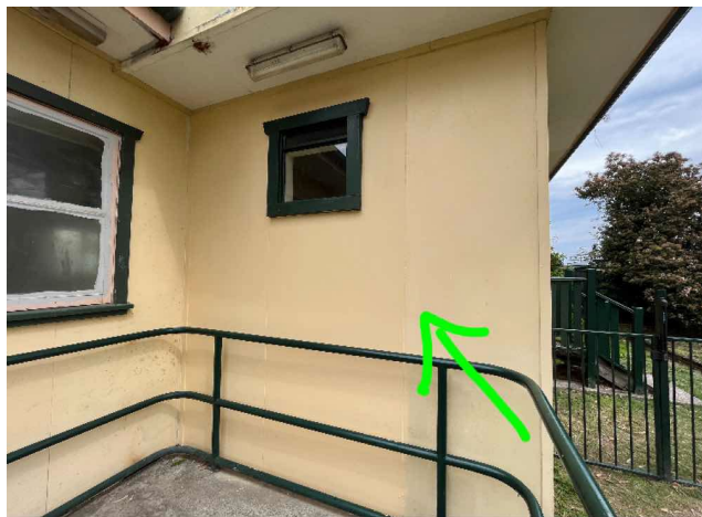
External, GF, Exterior, East, External wall - Fibre Cement Sheet, No Asbestos Detected, B17380S04
