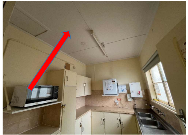
Internal, GF, Kitchen, Ceiling Lining - Fibre Cement, Assumed Positive, Similar to B17380S15 - Assumed Chrysotile
