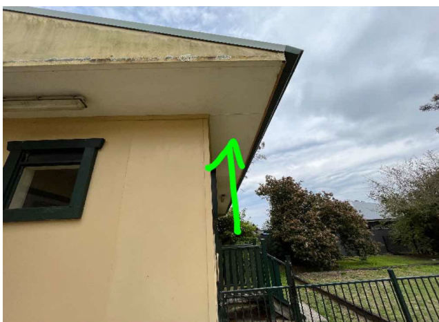
External, GF, Exterior, North, Eaves - Fibre Cement Sheet, No
