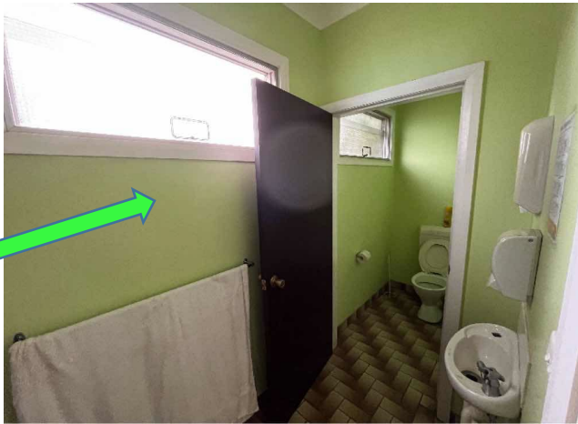
Internal, GF, Amenities, Ceilings and Walls - Fibre Cement, No Asbestos identified, B17380S14
