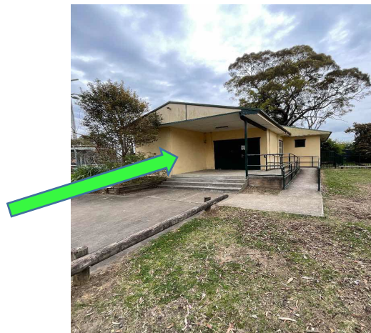
External, GF, Exterior, North East, Wall cladding - Fibre Cement Sheet, No Asbestos Detected, B17380S24 & B17380S28
