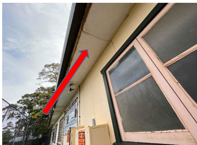
External, GF, Exterior, South, Eaves adjacent original hall - Fibre Cement
