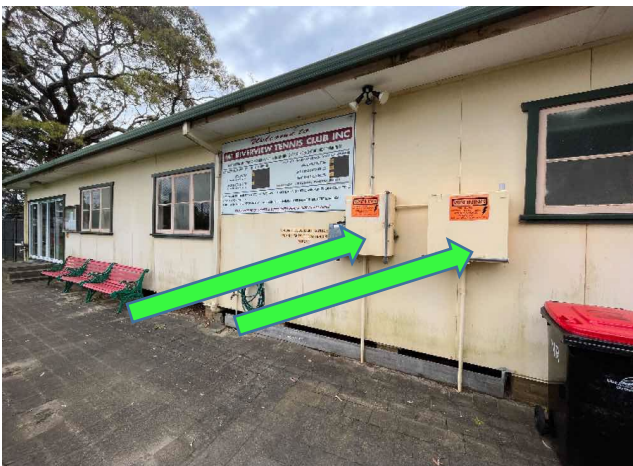
External, GF, Exterior, Wall - Electrical backing board, No Asbestos Detected, -
