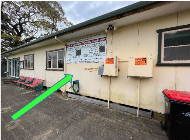
External, GF, Exterior, External walls - Cream - Topcoat, Lead Not Detected (<0.05%w/w), 17380-2
