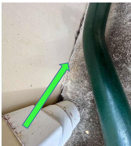
External, GF, Exterior, North, External wall - Fibre Cement Sheeting, No Asbestos Detected, B17380S08
