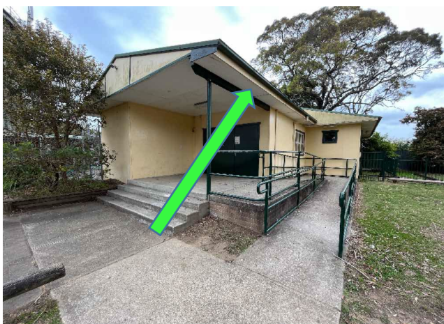
External, GF, Exterior, North East, Eave - Fibre Cement Sheet, No Asbestos Detected, Similar to B17380S24
