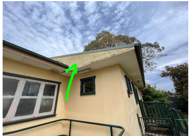
External, GF, Exterior, East, Gable infill - Fibre Cement Sheet, No Asbestos Detected, B17380S01 & B17380S26
