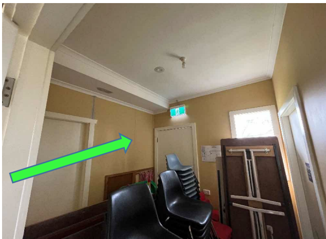
Internal, GF, Gutory Room, West And South, Wall Cladding - Fibre Cement, No Asbestos identified, B17380-S19 & B17380-S20
