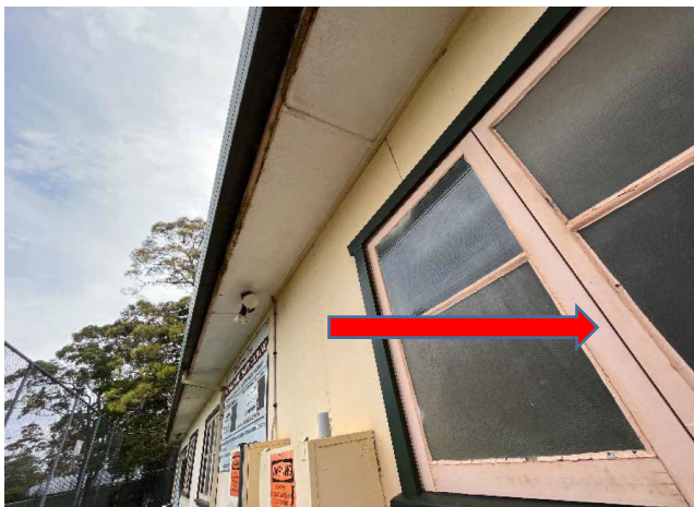
External, GF, All Windows, Frames - Pink - Topcoat, Lead Detected (%0.82 w/w), 17380-1
