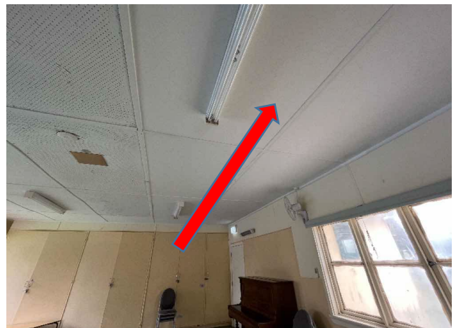
Internal, GF, Hall, Ceiling Lining - Fibre Cement, Chrysotile, B17380S15
