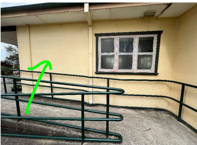
External, GF, Exterior, North, External wall - Fibre Cement Sheet, No Asbestos Detected, B17380S06
