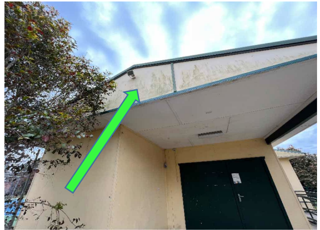
External, GF, Exterior, East, Gable end - Fibre Cement Sheet, No Asbestos Detected, B17380 S24
