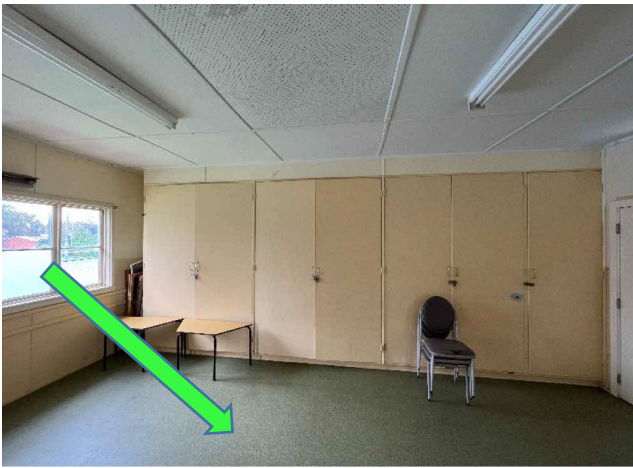
Internal, GF, Hall, Floor Linoleum - Linoleum, No Asbestos identified, B17380S16
