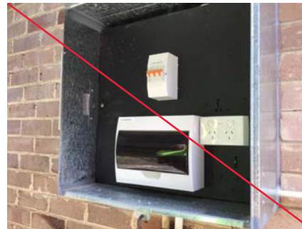
PHOTO NO.: J154900-001-PHOTO088 RESULT: ASBESTOS - PRESUMED POSITIVE BUILDING/LEVEL: STORAGE SHED - GROUND LEVEL ROOM/LOCATION: EXTERIOR - NORTH FEATURE/MATERIAL: ELECTRICAL - SWITCH BOARD - COMPRESSED BITUMINOUS ELECTRICAL PANEL SAMPLE NO.: SIMILAR TO:
