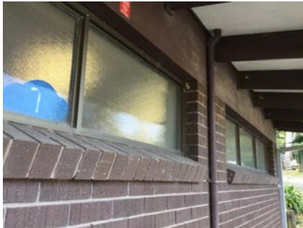
PHOTO NO.: J154900-001-PHOTO125 RESULT: ASBESTOS - POSITIVE BUILDING/LEVEL: AMENITIES BUILDING - ALL LEVELS ROOM/LOCATION: EXTERIOR - EAST & WEST FEATURE/MATERIAL: INFILL PANELS - FIBRE CEMENT SHEETING SAMPLE NO.: J154900-001-049
