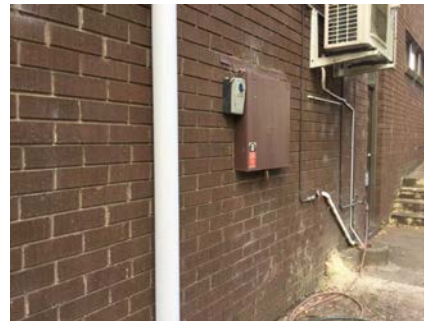
PHOTO NO.: J154900-001-PHOTO112 RESULT: ASBESTOS - PRESUMED POSITIVE BUILDING/LEVEL: AMENITIES BUILDING - GROUND LEVEL ROOM/LOCATION: EXTERIOR - SOUTH FEATURE/MATERIAL: ELECTRICAL - SWITCH BOARD - COMPRESSED BITUMINOUS ELECTRICAL PANEL SAMPLE NO.: NOT SAMPLED LOCKED
