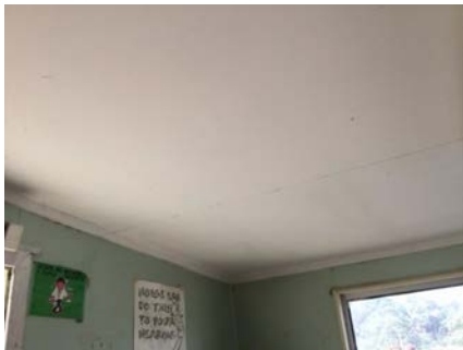
PHOTO NO.: J154900-001-PHOTO076 RESULT: ASBESTOS - NEGATIVE BUILDING/LEVEL: TRADES SHED - GROUND LEVEL ROOM/LOCATION: MEALS ROOM - THROUGHOUT FEATURE/MATERIAL: CEILING - FIBRE CEMENT SHEETING SAMPLE NO.: J154900-001-041
