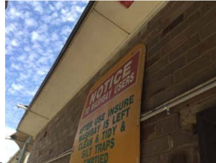
PHOTO NO.: J154900-001-PHOTO084 RESULT: ASBESTOS - POSITIVE BUILDING/LEVEL: STORAGE SHED - GROUND LEVEL ROOM/LOCATION: EXTERIOR - VARIOUS THROUGHOUT FEATURE/MATERIAL: EAVES - FIBRE CEMENT SHEETING SAMPLE NO.: PREVIOUSLY SAMPLED REGIONAL ENVIROSCIENCE B17336-S19
