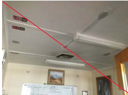
PHOTO NO.: J154900-001-PHOTO012 RESULT: ASBESTOS - POSITIVE BUILDING/LEVEL: ADMINISTRATION BUILDING - GROUND LEVEL ROOM/LOCATION: SOUTHERN OFFICE - BULK WASTE COORDINATOR OFFICE - VARIOUS THROUGHOUT FEATURE/MATERIAL: CEILING - FIBRE CEMENT SHEETING SAMPLE NO.: PREVIOUSLY SAMPLED REGIONAL ENVIROSCIENCE B17336-S10
