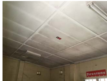
PHOTO NO.: J154900-001-PHOTO086 RESULT: ASBESTOS - POSITIVE BUILDING/LEVEL: STORAGE SHED - GROUND LEVEL ROOM/LOCATION: EAST STORE ROOM - THROUGHOUT FEATURE/MATERIAL: CEILING - FIBRE CEMENT SHEETING SAMPLE NO.: PREVIOUSLY SAMPLED REGIONAL ENVIROSCIENCE B17336-S19
