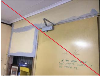
PHOTO NO.: J154900-001-PHOTO021 RESULT: ASBESTOS - POSITIVE BUILDING/LEVEL: ADMINISTRATION BUILDING - GROUND LEVEL ROOM/LOCATION: WASTE SERVICES OFFICE - KEY RETURN AREA - SOUTH FEATURE/MATERIAL: WALL - FIBRE CEMENT SHEETING SAMPLE NO.: J154900-001-026
