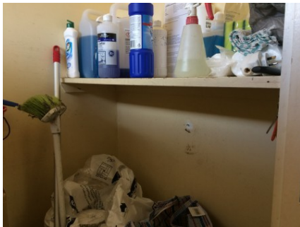
PHOTO NO.: J154900-001-PHOTO139 RESULT: ASBESTOS - POSITIVE BUILDING/LEVEL: AMENITIES BUILDING - GROUND LEVEL ROOM/LOCATION: CLEANER ROOM (WITHIN MALE TOILET) - WEST FEATURE/MATERIAL: WALL - FIBRE CEMENT SHEETING SAMPLE NO.: J154900-001-020
