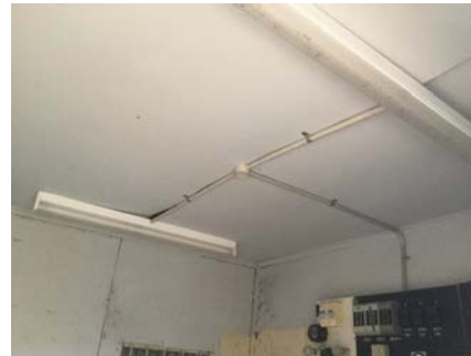
PHOTO NO.: J154900-001-PHOTO079 RESULT: BUILDING/LEVEL: TRADES SHED - GROUND LEVEL ROOM/LOCATION: OFFICE/STORE - NORTHWEST - VARIOUS THROUGHOUT FEATURE/MATERIAL: NON-HAZARDOUS FEATURE - NON-HAZARDOUS MATERIAL SAMPLE NO.: -
