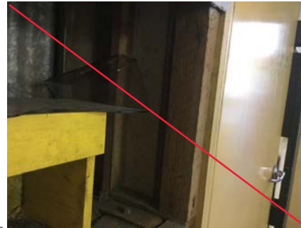
PHOTO NO.: J154900-001-PHOTO024 RESULT: ASBESTOS - PRESUMED POSITIVE BUILDING/LEVEL: ADMINISTRATION BUILDING - GROUND LEVEL ROOM/LOCATION: WASTE SERVICES OFFICE - KEY RETURN AREA - SOUTH FEATURE/MATERIAL: WALL - FIBRE CEMENT SHEETING SAMPLE NO.: SIMILAR TO: J154900-001-026
