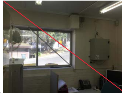
PHOTO NO.: J154900-001-PHOTO015 RESULT: ASBESTOS - POSITIVE BUILDING/LEVEL: ADMINISTRATION BUILDING - GROUND LEVEL ROOM/LOCATION: WASTE SERVICES OFFICE - HUMAN RESOURCES ROOM - WEST FEATURE/MATERIAL: WALL LINING - FIBRE CEMENT SHEETING SAMPLE NO.: J154900-001-024
