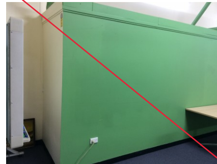
PHOTO NO.: J154900-001-PHOTO152 RESULT: ASBESTOS - POSITIVE BUILDING/LEVEL: AMENITIES BUILDING - LEVEL ONE ROOM/LOCATION: CONFERENCE ROOM - EAST FEATURE/MATERIAL: WALL - FIBRE CEMENT SHEETING SAMPLE NO.: J154900-001-012
