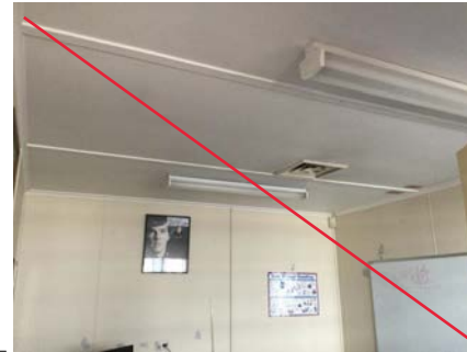
PHOTO NO.: J154900-001-PHOTO009 RESULT: ASBESTOS - POSITIVE BUILDING/LEVEL: ADMINISTRATION BUILDING - GROUND LEVEL ROOM/LOCATION: SOUTHERN OFFICE - WASTE KERBSIDE/ADMIN OFFICE - VARIOUS THROUGHOUT FEATURE/MATERIAL: CEILING - FIBRE CEMENT SHEETING SAMPLE NO.: PREVIOUSLY SAMPLED REGIONAL ENVIROSCIENCE B17336-S10
