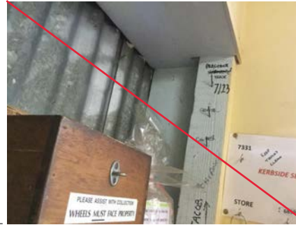
PHOTO NO.: J154900-001-PHOTO025 RESULT: ASBESTOS - PRESUMED POSITIVE BUILDING/LEVEL: ADMINISTRATION BUILDING - GROUND LEVEL ROOM/LOCATION: WASTE SERVICES OFFICE - KEY RETURN AREA - SOUTH FEATURE/MATERIAL: WALL - FIBRE CEMENT SHEETING SAMPLE NO.: SIMILAR TO: J154900-001-026
