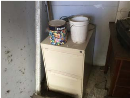
PHOTO NO.: J154900-001-PHOTO073 RESULT: ASBESTOS - NEGATIVE BUILDING/LEVEL: TRADES SHED - GROUND LEVEL ROOM/LOCATION: OFFICE/STORE - NORTHWEST - SOUTHEAST FEATURE/MATERIAL: LOWER WALL LINING - FIBRE CEMENT SHEETING SAMPLE NO.: J154900-001-039
