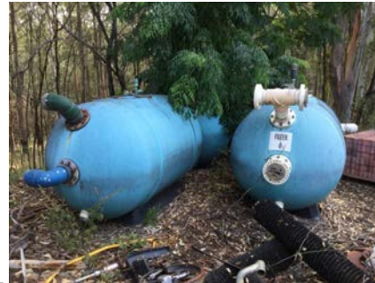
PHOTO NO.: J154900-001-PHOTO118 RESULT: ASBESTOS - NEGATIVE BUILDING/LEVEL: WORKSHOP - GROUND LEVEL ROOM/LOCATION: EXTERIOR - SOUTHWEST FEATURE/MATERIAL: STORAGE TANK - GASKET SAMPLE NO.: J154900-001-047
