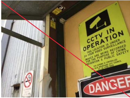
PHOTO NO.: J154900-001-PHOTO083 RESULT: ASBESTOS - POSITIVE BUILDING/LEVEL: ADMINISTRATION BUILDING - GROUND LEVEL ROOM/LOCATION: EXTERIOR - SOUTHEAST FEATURE/MATERIAL: INFILL PANELS - FIBRE CEMENT SHEETING SAMPLE NO.: PREVIOUSLY SAMPLED REGIONAL ENVIROSCIENCE B17336-S07
