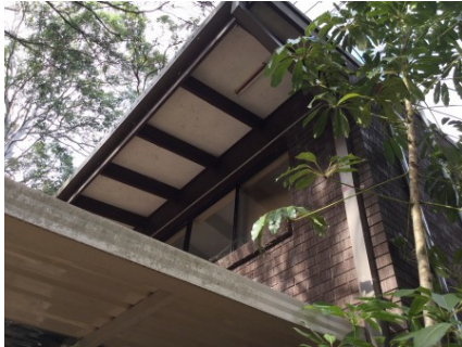
PHOTO NO.: J154900-001-PHOTO158 RESULT: ASBESTOS - PREVIOUSLY SAMPLED POSITIVE BUILDING/LEVEL: AMENITIES BUILDING - ALL LEVELS ROOM/LOCATION: EXTERIOR - EAST & WEST FEATURE/MATERIAL: AWNING - FIBRE CEMENT SHEETING SAMPLE NO.: PREVIOUSLY SAMPLED REGIONAL ENVIROSCIENCE B17336-S12
