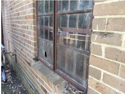
PHOTO NO.: J154900-001-PHOTO094 RESULT: ASBESTOS - NEGATIVE BUILDING/LEVEL: STORAGE SHED - GROUND LEVEL ROOM/LOCATION: EXTERIOR - SOUTH FEATURE/MATERIAL: WINDOW FRAMES - PUTTY SAMPLE NO.: J154900-001-042
