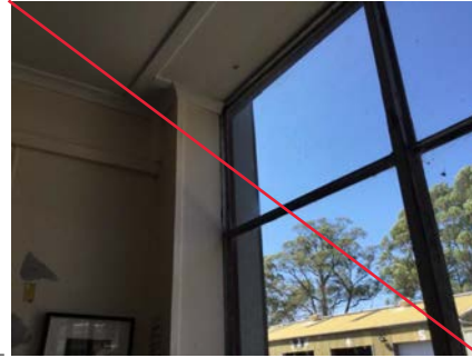
PHOTO NO.: J154900-001-PHOTO033 RESULT: ASBESTOS - POSITIVE BUILDING/LEVEL: ADMINISTRATION BUILDING - GROUND LEVEL ROOM/LOCATION: HALLWAY - SOUTHERN OFFICE - VARIOUS THROUGHOUT FEATURE/MATERIAL: WALL - FIBRE CEMENT SHEETING SAMPLE NO.: PREVIOUSLY SAMPLED REGIONAL ENVIROSCIENCE B17336-S09
