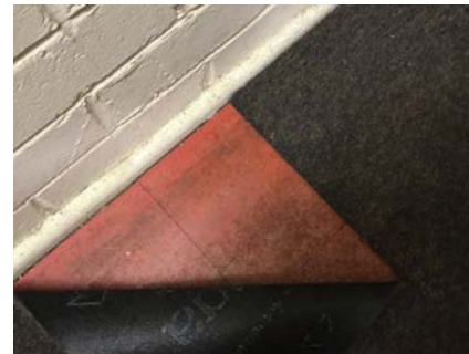
PHOTO NO.: J154900-001-PHOTO028 RESULT: ASBESTOS - PRESUMED NEGATIVE BUILDING/LEVEL: ADMINISTRATION BUILDING - GROUND LEVEL ROOM/LOCATION: WASTE SERVICES OFFICE - TRUCKS COORDINATOR ROOM - THROUGHOUT FEATURE/MATERIAL: FLOOR COVERING - VINYL TILES & ADHESIVE SAMPLE NO.: SIMILAR TO: J154900-001-023
