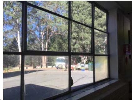
PHOTO NO.: J154900-001-PHOTO017 RESULT: ASBESTOS - NEGATIVE BUILDING/LEVEL: ADMINISTRATION BUILDING - GROUND LEVEL ROOM/LOCATION: WASTE SERVICES OFFICE - HALLWAY - SOUTH FEATURE/MATERIAL: WINDOW FRAMES - PUTTY SAMPLE NO.: J154900-001-025
