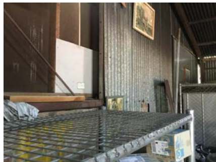
PHOTO NO.: J154900-001-PHOTO036 RESULT: ASBESTOS - NEGATIVE BUILDING/LEVEL: ADMINISTRATION BUILDING - GROUND LEVEL ROOM/LOCATION: WASTE BINS SHED - WEST FEATURE/MATERIAL: SWITCHBOARD BACKING PANEL - FIBRE CEMENT SHEETING SAMPLE NO.: J154900-001-028
