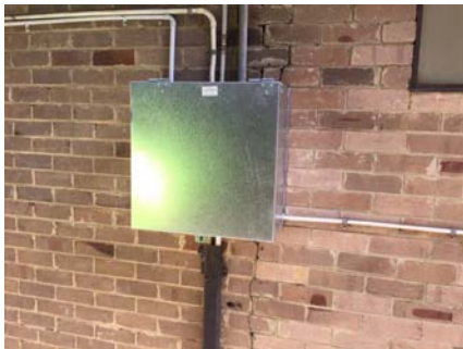
PHOTO NO.: J154900-001-PHOTO089 RESULT: ASBESTOS - PRESUMED POSITIVE BUILDING/LEVEL: STORAGE SHED - GROUND LEVEL ROOM/LOCATION: EXTERIOR - NORTH FEATURE/MATERIAL: ELECTRICAL - SWITCH BOARD - COMPRESSED BITUMINOUS ELECTRICAL PANEL SAMPLE NO.: SIMILAR TO:
