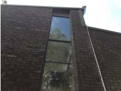
PHOTO NO.: J154900-001-PHOTO114 RESULT: ASBESTOS - POSITIVE BUILDING/LEVEL: AMENITIES BUILDING - GROUND LEVEL ROOM/LOCATION: EXTERIOR - NORTH & SOUTH FEATURE/MATERIAL: INFILL PANELS - FIBRE CEMENT SHEETING SAMPLE NO.: PREVIOUSLY SAMPLED REGIONAL ENVIROSCIENCE B17336-S13
