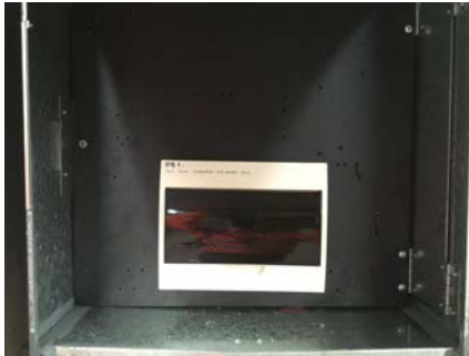
PHOTO NO.: J154900-001-PHOTO047 RESULT: ASBESTOS - NEGATIVE BUILDING/LEVEL: ADMINISTRATION BUILDING - GROUND LEVEL ROOM/LOCATION: RMT SHED - SOUTHWEST FEATURE/MATERIAL: ELECTRICAL - SWITCH BOARD - DUST SAMPLE NO.: J154900-001-032
