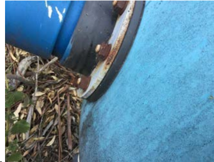
PHOTO NO.: J154900-001-PHOTO120 RESULT: ASBESTOS - NEGATIVE BUILDING/LEVEL: WORKSHOP - GROUND LEVEL ROOM/LOCATION: EXTERIOR - SOUTHWEST FEATURE/MATERIAL: STORAGE TANK - GASKET SAMPLE NO.: J154900-001-047
