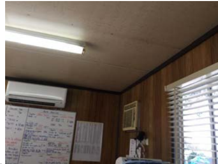
PHOTO NO.: J154900-001-PHOTO101 RESULT: BUILDING/LEVEL: WORKSHOP - GROUND LEVEL ROOM/LOCATION: OFFICE (ADJACENT TEA ROOM) - VARIOUS THROUGHOUT FEATURE/MATERIAL: NON-HAZARDOUS FEATURE - NON-HAZARDOUS MATERIAL SAMPLE NO.: -
