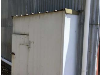
PHOTO NO.: J154900-001-PHOTO068 RESULT: ASBESTOS - NEGATIVE BUILDING/LEVEL: TRADES SHED - GROUND LEVEL ROOM/LOCATION: PUMP SHED - SOUTHEAST - THROUGHOUT FEATURE/MATERIAL: WALL - FIBRE CEMENT SHEETING SAMPLE NO.: J154900-001-036
