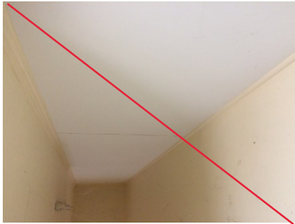
PHOTO NO.: J154900-001-PHOTO147 RESULT: ASBESTOS - PRESUMED POSITIVE BUILDING/LEVEL: AMENITIES BUILDING - LEVEL ONE ROOM/LOCATION: REAR STAIRWELL - TO CONFERENCE ROOM - THROUGHOUT FEATURE/MATERIAL: CEILING - FIBRE CEMENT SHEETING SAMPLE NO.: SIMILAR TO: J154900-001-006
