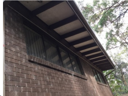
PHOTO NO.: J154900-001-PHOTO159 RESULT: ASBESTOS - PREVIOUSLY SAMPLED POSITIVE BUILDING/LEVEL: AMENITIES BUILDING - ALL LEVELS ROOM/LOCATION: EXTERIOR - EAST & WEST FEATURE/MATERIAL: AWNING - FIBRE CEMENT SHEETING SAMPLE NO.: PREVIOUSLY SAMPLED REGIONAL ENVIROSCIENCE B17336-S12
