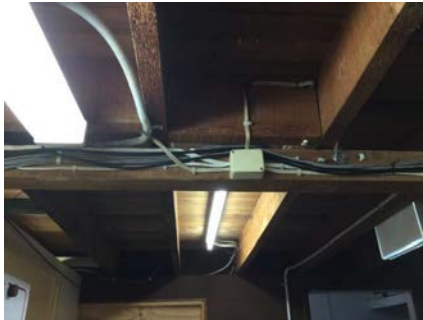
PHOTO NO.: J154900-001-PHOTO046 RESULT: BUILDING/LEVEL: ADMINISTRATION BUILDING - GROUND LEVEL ROOM/LOCATION: SIGN- IN OFFICE/PPE STORE - VARIOUS THROUGHOUT FEATURE/MATERIAL: NON-HAZARDOUS FEATURE - NON-HAZARDOUS MATERIAL SAMPLE NO.: -
