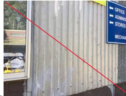
PHOTO NO.: J154900-001-PHOTO038 RESULT: ASBESTOS - POSITIVE BUILDING/LEVEL: ADMINISTRATION BUILDING - GROUND LEVEL ROOM/LOCATION: EXTERIOR - SOUTHWEST FEATURE/MATERIAL: WALL LINING - FIBRE CEMENT SHEETING SAMPLE NO.: J154900-001-029
