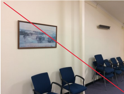
PHOTO NO.: J154900-001-PHOTO153 RESULT: ASBESTOS - POSITIVE BUILDING/LEVEL: AMENITIES BUILDING - LEVEL ONE ROOM/LOCATION: CONFERENCE ROOM - SOUTH FEATURE/MATERIAL: WALL - FIBRE CEMENT SHEETING SAMPLE NO.: J154900-001-013
