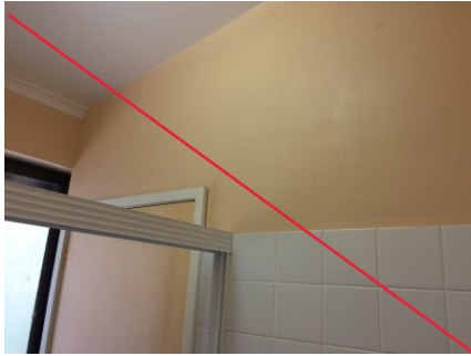
PHOTO NO.: J154900-001-PHOTO142 RESULT: ASBESTOS - PRESUMED POSITIVE BUILDING/LEVEL: AMENITIES BUILDING - LEVEL ONE ROOM/LOCATION: FEMALE SHOWER - THROUGHOUT FEATURE/MATERIAL: CEILING - FIBRE CEMENT SHEETING SAMPLE NO.: SIMILAR TO: J154900-001-006
