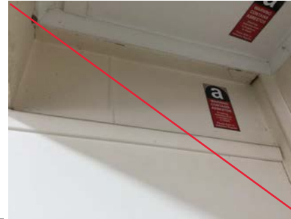
PHOTO NO.: J154900-001-PHOTO030 RESULT: ASBESTOS - POSITIVE BUILDING/LEVEL: ADMINISTRATION BUILDING - GROUND LEVEL ROOM/LOCATION: WASTE SERVICES OFFICE - KITCHENETTE - WEST FEATURE/MATERIAL: WALL - FIBRE CEMENT SHEETING SAMPLE NO.: PREVIOUSLY SAMPLED REGIONAL ENVIROSCIENCE B17336-S09
