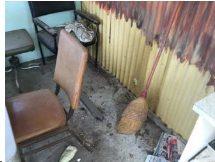
PHOTO NO.: J154900-001-PHOTO077 RESULT: BUILDING/LEVEL: TRADES SHED - GROUND LEVEL ROOM/LOCATION: MEALS ROOM - VARIOUS THROUGHOUT FEATURE/MATERIAL: NON-HAZARDOUS FEATURE - NON-HAZARDOUS MATERIAL SAMPLE NO.: -
