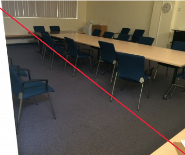
PHOTO NO.: J154900-001-PHOTO160 RESULT: ASBESTOS - POSITIVE BUILDING/LEVEL: AMENITIES BUILDING - LEVEL ONE ROOM/LOCATION: CONFERENCE ROOM - THROUGHOUT FEATURE/MATERIAL: FLOOR COVERING - VINYL TILES & ADHESIVE SAMPLE NO.: PREVIOUSLY SAMPLED REGIONAL ENVIROSCIENCE B17336-S14
