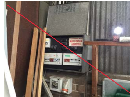
PHOTO NO.: J154900-001-PHOTO041 RESULT: ASBESTOS - POSITIVE BUILDING/LEVEL: ADMINISTRATION BUILDING - GROUND LEVEL ROOM/LOCATION: STORE SHED - NORTHEAST FEATURE/MATERIAL: ELECTRICAL - SWITCH BOARD - COMPRESSED BITUMINOUS ELECTRICAL PANEL SAMPLE NO.: SIMILAR TO: J154900-001-038
