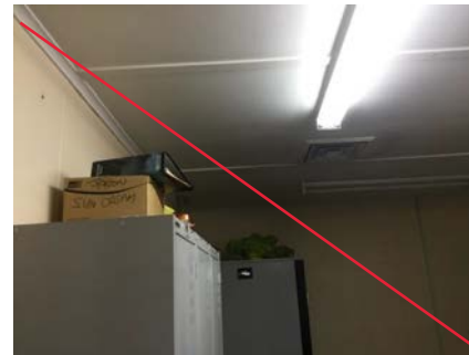
PHOTO NO.: J154900-001-PHOTO011 RESULT: ASBESTOS - POSITIVE BUILDING/LEVEL: ADMINISTRATION BUILDING - GROUND LEVEL ROOM/LOCATION: SOUTHERN OFFICE - PRINTER ROOM - VARIOUS THROUGHOUT FEATURE/MATERIAL: CEILING - FIBRE CEMENT SHEETING SAMPLE NO.: PREVIOUSLY SAMPLED REGIONAL ENVIROSCIENCE B17336-S10
