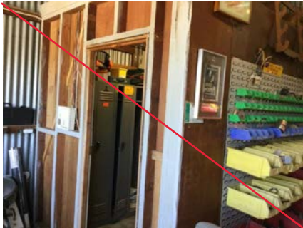
PHOTO NO.: J154900-001-PHOTO060 RESULT: ASBESTOS - POSITIVE BUILDING/LEVEL: GARDENERS SHED - GROUND LEVEL ROOM/LOCATION: LOCKER ROOM (LOWER LEVEL) - SOUTH FEATURE/MATERIAL: DEBRIS - FIBRE CEMENT DEBRIS SAMPLE NO.: PREVIOUSLY SAMPLED REGIONAL ENVIROSCIENCE B17336-S26
