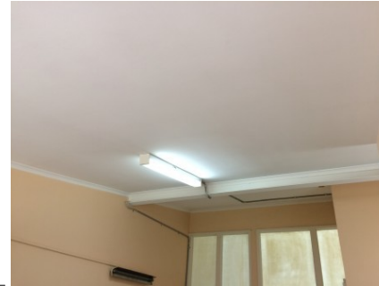
PHOTO NO.: J154900-001-PHOTO155 RESULT: ASBESTOS - PRESUMED POSITIVE BUILDING/LEVEL: AMENITIES BUILDING - LEVEL ONE ROOM/LOCATION: FEMALE TOILET - THROUGHOUT FEATURE/MATERIAL: CEILING - FIBRE CEMENT SHEETING SAMPLE NO.: SIMILAR TO: J154900-001-006
