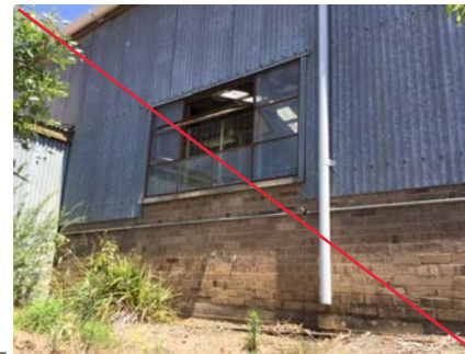
PHOTO NO.: J154900-001-PHOTO056 RESULT: ASBESTOS - NEGATIVE BUILDING/LEVEL: ADMINISTRATION BUILDING - GROUND LEVEL ROOM/LOCATION: EXTERIOR - VARIOUS THROUGHOUT FEATURE/MATERIAL: WINDOW FRAMES - PUTTY SAMPLE NO.: J154900-001-033
