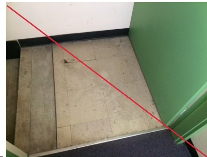
PHOTO NO.: J154900-001-PHOTO157 RESULT: ASBESTOS - POSITIVE BUILDING/LEVEL: AMENITIES BUILDING - LEVEL ONE ROOM/LOCATION: REAR STAIRWELL - TO CONFERENCE ROOM - ENTRY AREA FEATURE/MATERIAL: FLOOR COVERING - VINYL TILES & ADHESIVE SAMPLE NO.: PREVIOUSLY SAMPLED REGIONAL ENVIROSCIENCE B17336-S14
