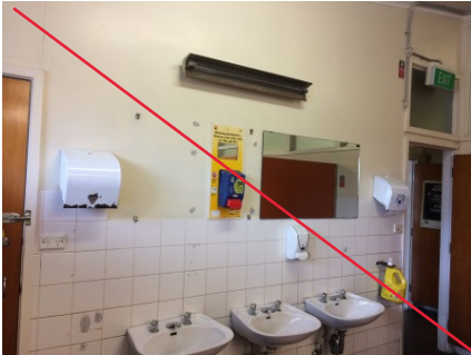
PHOTO NO.: J154900-001-PHOTO134 RESULT: ASBESTOS - POSITIVE BUILDING/LEVEL: AMENITIES BUILDING - GROUND LEVEL ROOM/LOCATION: MALE TOILET - SOUTH FEATURE/MATERIAL: WALL - FIBRE CEMENT SHEETING SAMPLE NO.: J154900-001-019
