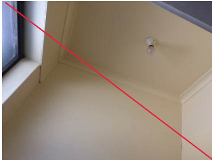
PHOTO NO.: J154900-001-PHOTO137 RESULT: ASBESTOS - PRESUMED POSITIVE BUILDING/LEVEL: AMENITIES BUILDING - GROUND LEVEL ROOM/LOCATION: CLEANER ROOM (WITHIN MALE TOILET) - THROUGHOUT FEATURE/MATERIAL: CEILING - FIBRE CEMENT SHEETING SAMPLE NO.: SIMILAR TO: J154900-001-001
