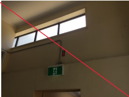
PHOTO NO.: J154900-001-PHOTO149 RESULT: ASBESTOS - POSITIVE BUILDING/LEVEL: AMENITIES BUILDING - LEVEL ONE ROOM/LOCATION: CENTRAL FOYER - TO CONFERENCE/FEMALE TOILET/SHOWER/ CHANGE ROOMS - EAST FEATURE/MATERIAL: WALL - FIBRE CEMENT SHEETING SAMPLE NO.: J154900-001-011
