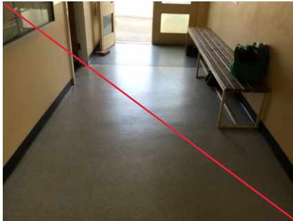
PHOTO NO.: J154900-001-PHOTO166 RESULT: ASBESTOS - PRESUMED POSITIVE BUILDING/LEVEL: AMENITIES BUILDING - GROUND LEVEL ROOM/LOCATION: FOYER - VARIOUS THROUGHOUT FEATURE/MATERIAL: WALL - FIBRE CEMENT SHEETING SAMPLE NO.: SIMILAR TO: J154900-001-020
