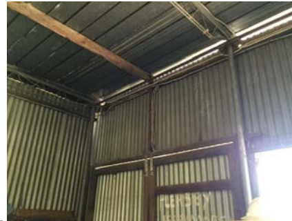
PHOTO NO.: J154900-001-PHOTO059 RESULT: BUILDING/LEVEL: GARDENERS SHED - GROUND LEVEL ROOM/LOCATION: ALL AREAS - VARIOUS THROUGHOUT FEATURE/MATERIAL: NON-HAZARDOUS FEATURE - NON-HAZARDOUS MATERIAL SAMPLE NO.: -
