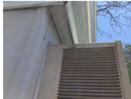
PHOTO NO.: J154900-001-PHOTO067 RESULT: ASBESTOS - NEGATIVE BUILDING/LEVEL: TRADES SHED - GROUND LEVEL ROOM/LOCATION: MEALS ROOM - THROUGHOUT FEATURE/MATERIAL: WALL - FIBRE CEMENT SHEETING SAMPLE NO.: J154900-001-035
