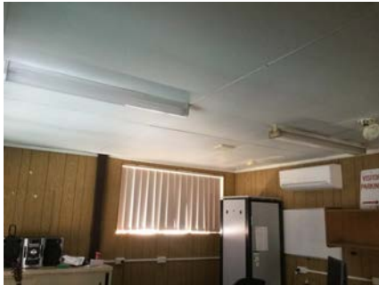
PHOTO NO.: J154900-001-PHOTO043 RESULT: BUILDING/LEVEL: ADMINISTRATION BUILDING - MEZZANINE LEVEL ROOM/LOCATION: MANAGER'S OFFICE - VARIOUS THROUGHOUT FEATURE/MATERIAL: NON-HAZARDOUS FEATURE - NON-HAZARDOUS MATERIAL SAMPLE NO.: -
