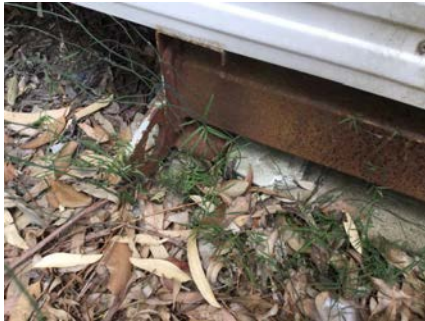
PHOTO NO.: J154900-001-PHOTO103 RESULT: ASBESTOS - NEGATIVE BUILDING/LEVEL: WORKSHOP - GROUND LEVEL ROOM/LOCATION: EXTERIOR - SOUTH FEATURE/MATERIAL: PACKER - FIBRE CEMENT SHEETING SAMPLE NO.: PREVIOUSLY SAMPLED REGIONAL ENVIROSCIENCE B17336-S25
