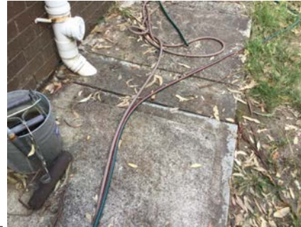
PHOTO NO.: J154900-001-PHOTO111 RESULT: ASBESTOS - NEGATIVE BUILDING/LEVEL: AMENITIES BUILDING - GROUND LEVEL ROOM/LOCATION: EXTERIOR - VARIOUS THROUGHOUT FEATURE/MATERIAL: EXPANSION JOINT - MASTIC SEALANT SAMPLE NO.: J154900-001-045
