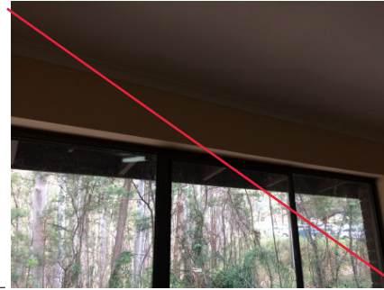
PHOTO NO.: J154900-001-PHOTO143 RESULT: ASBESTOS - PRESUMED POSITIVE BUILDING/LEVEL: AMENITIES BUILDING - LEVEL ONE ROOM/LOCATION: FEMALE SHOWER - WEST FEATURE/MATERIAL: INFILL PANELS - FIBRE CEMENT SHEETING SAMPLE NO.: SIMILAR TO: J154900-001-007
