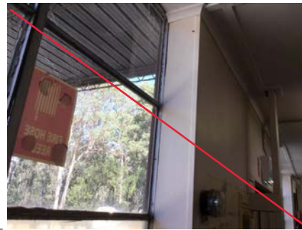
PHOTO NO.: J154900-001-PHOTO034 RESULT: ASBESTOS - POSITIVE BUILDING/LEVEL: ADMINISTRATION BUILDING - GROUND LEVEL ROOM/LOCATION: HALLWAY - SOUTHERN OFFICE - VARIOUS THROUGHOUT FEATURE/MATERIAL: WALL - FIBRE CEMENT SHEETING SAMPLE NO.: PREVIOUSLY SAMPLED REGIONAL ENVIROSCIENCE B17336-S09
