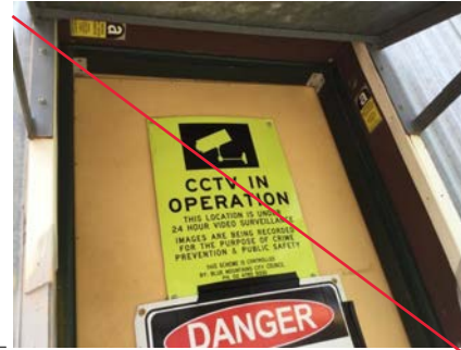
PHOTO NO.: J154900-001-PHOTO082 RESULT: ASBESTOS - POSITIVE BUILDING/LEVEL: ADMINISTRATION BUILDING - GROUND LEVEL ROOM/LOCATION: EXTERIOR - SOUTHEAST FEATURE/MATERIAL: INFILL PANELS - FIBRE CEMENT SHEETING SAMPLE NO.: PREVIOUSLY SAMPLED REGIONAL ENVIROSCIENCE B17336-S07
