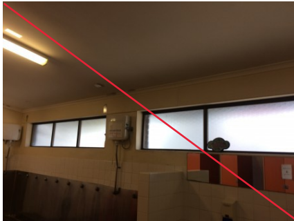
PHOTO NO.: J154900-001-PHOTO164 RESULT: ASBESTOS - PRESUMED POSITIVE BUILDING/LEVEL: AMENITIES BUILDING - GROUND LEVEL ROOM/LOCATION: LOCKER ROOM - THROUGHOUT FEATURE/MATERIAL: CEILING - FIBRE CEMENT SHEETING SAMPLE NO.: SIMILAR TO: J154900-001-001
