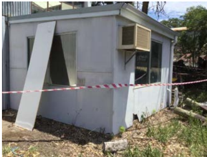
PHOTO NO.: J154900-001-PHOTO066 RESULT: ASBESTOS - NEGATIVE BUILDING/LEVEL: TRADES SHED - GROUND LEVEL ROOM/LOCATION: MEALS ROOM - THROUGHOUT FEATURE/MATERIAL: WALL - FIBRE CEMENT SHEETING SAMPLE NO.: J154900-001-035
