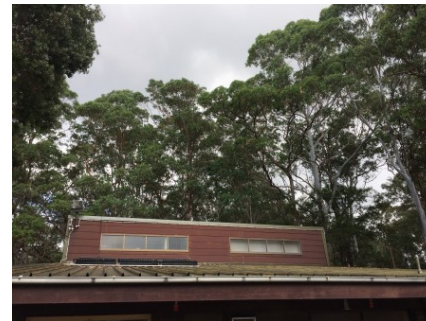
PHOTO NO.: J154900-001-PHOTO130 RESULT: ASBESTOS - POSITIVE BUILDING/LEVEL: AMENITIES BUILDING - LEVEL ONE ROOM/LOCATION: EXTERIOR - EAST FEATURE/MATERIAL: WALL CLADDING - FIBRE CEMENT SHEETING SAMPLE NO.: PREVIOUSLY SAMPLED REGIONAL ENVIROSCIENCE B17336-S14
