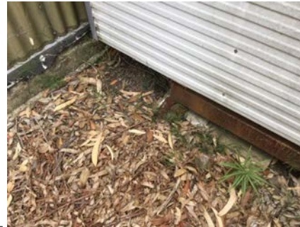
PHOTO NO.: J154900-001-PHOTO102 RESULT: ASBESTOS - NEGATIVE BUILDING/LEVEL: WORKSHOP - GROUND LEVEL ROOM/LOCATION: EXTERIOR - SOUTH FEATURE/MATERIAL: PACKER - FIBRE CEMENT SHEETING SAMPLE NO.: PREVIOUSLY SAMPLED REGIONAL ENVIROSCIENCE B17336-S25
