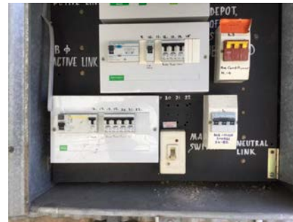
PHOTO NO.: J154900-001-PHOTO037 RESULT: ASBESTOS - PRESUMED NEGATIVE BUILDING/LEVEL: ADMINISTRATION BUILDING - GROUND LEVEL ROOM/LOCATION: EXTERIOR - SOUTH FEATURE/MATERIAL: ELECTRICAL - SWITCH BOARD - COMPRESSED BITUMINOUS ELECTRICAL PANEL SAMPLE NO.: NOT SAMPLED NEW APPEARANCE
