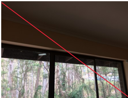
PHOTO NO.: J154900-001-PHOTO146 RESULT: ASBESTOS - POSITIVE BUILDING/LEVEL: AMENITIES BUILDING - LEVEL ONE ROOM/LOCATION: FEMALE CHANGE ROOM - WEST FEATURE/MATERIAL: INFILL PANELS - FIBRE CEMENT SHEETING SAMPLE NO.: J154900-001-007
