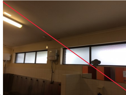
PHOTO NO.: J154900-001-PHOTO135 RESULT: ASBESTOS - PRESUMED POSITIVE BUILDING/LEVEL: AMENITIES BUILDING - GROUND LEVEL ROOM/LOCATION: MALE TOILET - THROUGHOUT FEATURE/MATERIAL: CEILING - FIBRE CEMENT SHEETING SAMPLE NO.: SIMILAR TO: J154900-001-001
