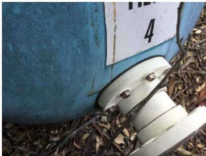
PHOTO NO.: J154900-001-PHOTO119 RESULT: ASBESTOS - NEGATIVE BUILDING/LEVEL: WORKSHOP - GROUND LEVEL ROOM/LOCATION: EXTERIOR - SOUTHWEST FEATURE/MATERIAL: STORAGE TANK - GASKET SAMPLE NO.: J154900-001-047
