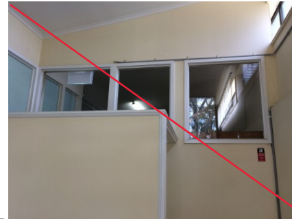
PHOTO NO.: J154900-001-PHOTO150 RESULT: ASBESTOS - PRESUMED POSITIVE BUILDING/LEVEL: AMENITIES BUILDING - LEVEL ONE ROOM/LOCATION: CENTRAL FOYER - TO CONFERENCE/FEMALE TOILET/SHOWER/ CHANGE ROOMS - THROUGHOUT FEATURE/MATERIAL: CEILING - FIBRE CEMENT SHEETING SAMPLE NO.: SIMILAR TO: J154900-001-006
