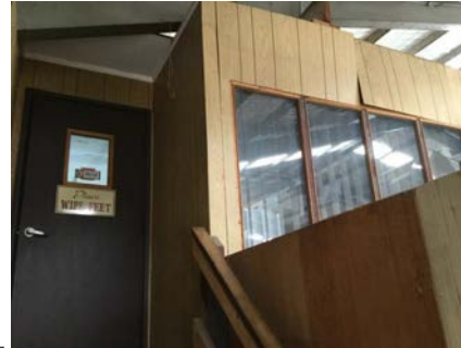
PHOTO NO.: J154900-001-PHOTO042 RESULT: BUILDING/LEVEL: ADMINISTRATION BUILDING - MEZZANINE LEVEL ROOM/LOCATION: MANAGER'S OFFICE - VARIOUS THROUGHOUT FEATURE/MATERIAL: NON-HAZARDOUS FEATURE - NON-HAZARDOUS MATERIAL SAMPLE NO.: -
