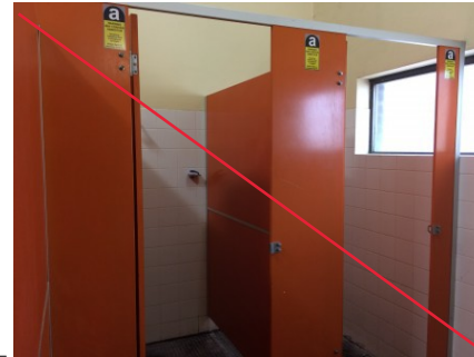
PHOTO NO.: J154900-001-PHOTO132 RESULT: ASBESTOS - POSITIVE BUILDING/LEVEL: AMENITIES BUILDING - GROUND LEVEL ROOM/LOCATION: LOCKER ROOM - NORTH FEATURE/MATERIAL: TOILET CUBICLE - COMPRESSED CEMENT SHEETING SAMPLE NO.: PREVIOUSLY SAMPLED REGIONAL ENVIROSCIENCE B17336-S15
