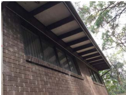
PHOTO NO.: J154900-001-PHOTO127 RESULT: ASBESTOS - POSITIVE BUILDING/LEVEL: AMENITIES BUILDING - ALL LEVELS ROOM/LOCATION: EXTERIOR - EAST & WEST FEATURE/MATERIAL: INFILL PANELS - FIBRE CEMENT SHEETING SAMPLE NO.: J154900-001-049
