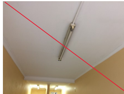
PHOTO NO.: J154900-001-PHOTO140 RESULT: ASBESTOS - POSITIVE BUILDING/LEVEL: AMENITIES BUILDING - GROUND LEVEL ROOM/LOCATION: FOYER - THROUGHOUT FEATURE/MATERIAL: CEILING - FIBRE CEMENT SHEETING SAMPLE NO.: J154900-001-020
