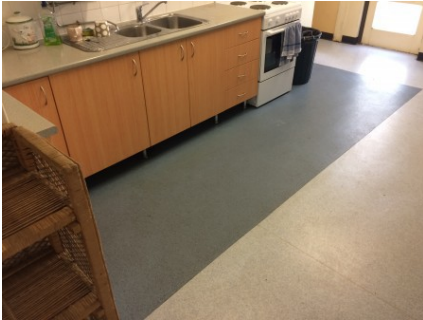
PHOTO NO.: J154900-001-PHOTO161 RESULT: ASBESTOS - NEGATIVE BUILDING/LEVEL: AMENITIES BUILDING - LOWER GROUND LEVEL ROOM/LOCATION: LUNCH ROOM - VARIOUS THROUGHOUT FEATURE/MATERIAL: FLOOR COVERING - SHEET VINYL & ADHESIVE SAMPLE NO.: PREVIOUSLY SAMPLED REGIONAL ENVIROSCIENCE B17336-S32
