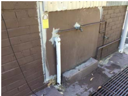
PHOTO NO.: J154900-001-PHOTO039 RESULT: ASBESTOS - NEGATIVE BUILDING/LEVEL: ADMINISTRATION BUILDING - GROUND LEVEL ROOM/LOCATION: EXTERIOR - SOUTHWEST FEATURE/MATERIAL: WALL LINING - FIBRE CEMENT SHEETING SAMPLE NO.: J154900-001-030
