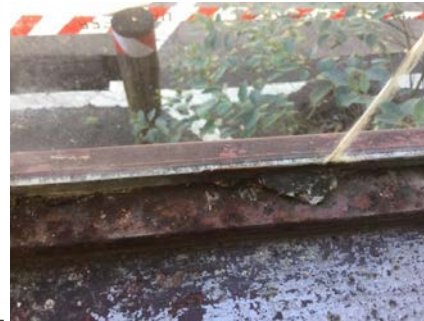
PHOTO NO.: J154900-001-PHOTO018 RESULT: ASBESTOS - NEGATIVE BUILDING/LEVEL: ADMINISTRATION BUILDING - GROUND LEVEL ROOM/LOCATION: WASTE SERVICES OFFICE - HALLWAY - SOUTH FEATURE/MATERIAL: WINDOW FRAMES - PUTTY SAMPLE NO.: J154900-001-025
