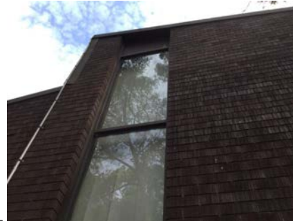
PHOTO NO.: J154900-001-PHOTO129 RESULT: ASBESTOS - POSITIVE BUILDING/LEVEL: AMENITIES BUILDING - GROUND LEVEL ROOM/LOCATION: EXTERIOR - NORTH & SOUTH FEATURE/MATERIAL: INFILL PANELS - FIBRE CEMENT SHEETING SAMPLE NO.: PREVIOUSLY SAMPLED REGIONAL ENVIROSCIENCE B17336-S13
