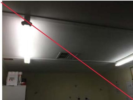
PHOTO NO.: J154900-001-PHOTO013 RESULT: ASBESTOS - POSITIVE BUILDING/LEVEL: ADMINISTRATION BUILDING - GROUND LEVEL ROOM/LOCATION: SOUTHERN OFFICE - TRUCKS COORDINATOR OFFICE - VARIOUS THROUGHOUT FEATURE/MATERIAL: CEILING - FIBRE CEMENT SHEETING SAMPLE NO.: PREVIOUSLY SAMPLED REGIONAL ENVIROSCIENCE B17336-S10
