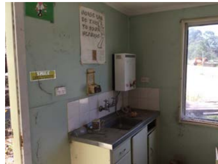
PHOTO NO.: J154900-001-PHOTO075 RESULT: ASBESTOS - NEGATIVE BUILDING/LEVEL: TRADES SHED - GROUND LEVEL ROOM/LOCATION: MEALS ROOM - THROUGHOUT FEATURE/MATERIAL: WALL - FIBRE CEMENT SHEETING SAMPLE NO.: J154900-001-040
