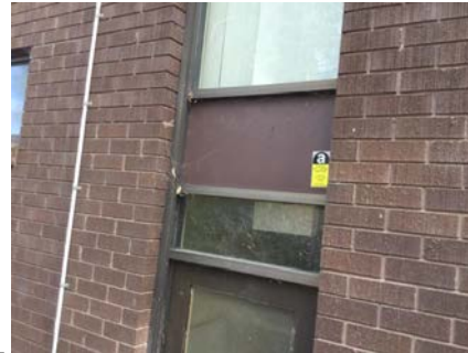
PHOTO NO.: J154900-001-PHOTO128 RESULT: ASBESTOS - POSITIVE BUILDING/LEVEL: AMENITIES BUILDING - GROUND LEVEL ROOM/LOCATION: EXTERIOR - NORTH & SOUTH FEATURE/MATERIAL: INFILL PANELS - FIBRE CEMENT SHEETING SAMPLE NO.: PREVIOUSLY SAMPLED REGIONAL ENVIROSCIENCE B17336-S13
