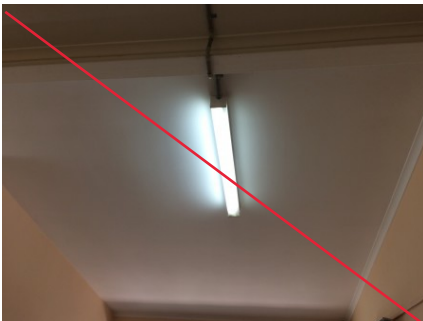
PHOTO NO.: J154900-001-PHOTO156 RESULT: ASBESTOS - POSITIVE BUILDING/LEVEL: AMENITIES BUILDING - LEVEL ONE ROOM/LOCATION: HAND WASH AREA (WITHIN FEMALE CHANGE ROOM) - THROUGHOUT FEATURE/MATERIAL: CEILING - FIBRE CEMENT SHEETING SAMPLE NO.: J154900-001-006
