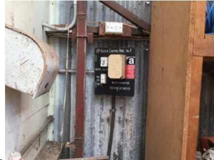
PHOTO NO.: J154900-001-PHOTO070 RESULT: ASBESTOS - PRESUMED POSITIVE BUILDING/LEVEL: TRADES SHED - GROUND LEVEL ROOM/LOCATION: MAIN SHED - WEST FEATURE/MATERIAL: ELECTRICAL - SWITCH BOARD - COMPRESSED BITUMINOUS ELECTRICAL PANEL SAMPLE NO.: SIMILAR TO: J154900-001-038
