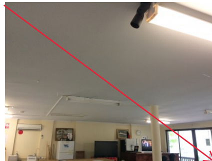
PHOTO NO.: J154900-001-PHOTO133 RESULT: ASBESTOS - POSITIVE BUILDING/LEVEL: AMENITIES BUILDING - LOWER GROUND LEVEL ROOM/LOCATION: LUNCH ROOM - THROUGHOUT FEATURE/MATERIAL: CEILING - FIBRE CEMENT SHEETING SAMPLE NO.: J154900-001-015
