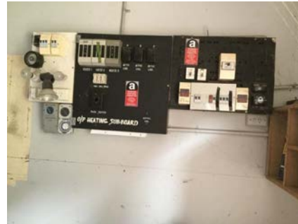
PHOTO NO.: J154900-001-PHOTO071 RESULT: ASBESTOS - PRESUMED POSITIVE BUILDING/LEVEL: TRADES SHED - GROUND LEVEL ROOM/LOCATION: OFFICE/STORE - NORTHWEST - WEST FEATURE/MATERIAL: ELECTRICAL - SWITCH BOARD - COMPRESSED BITUMINOUS ELECTRICAL PANEL SAMPLE NO.: SIMILAR TO: J154900-001-038
