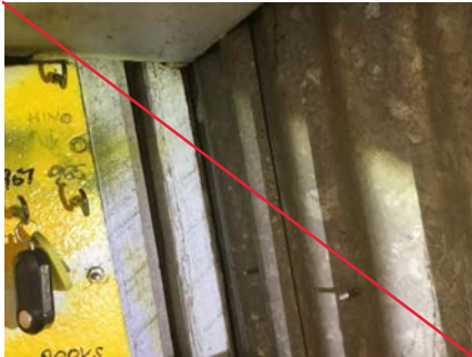
PHOTO NO.: J154900-001-PHOTO026 RESULT: ASBESTOS - PRESUMED POSITIVE BUILDING/LEVEL: ADMINISTRATION BUILDING - GROUND LEVEL ROOM/LOCATION: WASTE SERVICES OFFICE - KEY RETURN AREA - SOUTH FEATURE/MATERIAL: WALL - FIBRE CEMENT SHEETING SAMPLE NO.: SIMILAR TO: J154900-001-026
