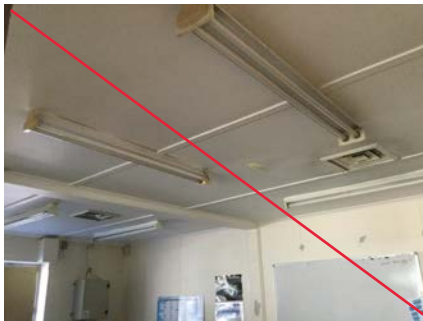
PHOTO NO.: J154900-001-PHOTO010 RESULT: ASBESTOS - POSITIVE BUILDING/LEVEL: ADMINISTRATION BUILDING - GROUND LEVEL ROOM/LOCATION: SOUTHERN OFFICE - HUMAN RESOURCES OFFICE - VARIOUS THROUGHOUT FEATURE/MATERIAL: CEILING - FIBRE CEMENT SHEETING SAMPLE NO.: PREVIOUSLY SAMPLED REGIONAL ENVIROSCIENCE B17336-S10
