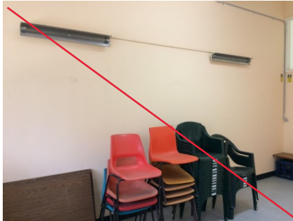
PHOTO NO.: J154900-001-PHOTO144 RESULT: ASBESTOS - POSITIVE BUILDING/LEVEL: AMENITIES BUILDING - LEVEL ONE ROOM/LOCATION: FEMALE CHANGE ROOM - NORTH FEATURE/MATERIAL: WALL - FIBRE CEMENT SHEETING SAMPLE NO.: J154900-001-005
