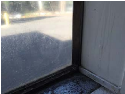
PHOTO NO.: J154900-001-PHOTO016 RESULT: ASBESTOS - NEGATIVE BUILDING/LEVEL: ADMINISTRATION BUILDING - GROUND LEVEL ROOM/LOCATION: WASTE SERVICES OFFICE - HALLWAY - SOUTH FEATURE/MATERIAL: WINDOW FRAMES - PUTTY SAMPLE NO.: J154900-001-025
