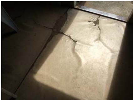
PHOTO NO.: J154900-001-PHOTO098 RESULT: ASBESTOS - NEGATIVE BUILDING/LEVEL: WORKSHOP - GROUND LEVEL ROOM/LOCATION: TEA ROOM - THROUGHOUT FEATURE/MATERIAL: FLOOR COVERING - SHEET VINYL SAMPLE NO.: PREVIOUSLY SAMPLED REGIONAL ENVIROSCIENCE B17336-S24
