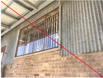
PHOTO NO.: J154900-001-PHOTO057 RESULT: ASBESTOS - NEGATIVE BUILDING/LEVEL: ADMINISTRATION BUILDING - GROUND LEVEL ROOM/LOCATION: EXTERIOR - VARIOUS THROUGHOUT FEATURE/MATERIAL: WINDOW FRAMES - PUTTY SAMPLE NO.: J154900-001-033
