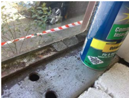
PHOTO NO.: J154900-001-PHOTO019 RESULT: ASBESTOS - NEGATIVE BUILDING/LEVEL: ADMINISTRATION BUILDING - GROUND LEVEL ROOM/LOCATION: WASTE SERVICES OFFICE - HALLWAY - SOUTH FEATURE/MATERIAL: WINDOW FRAMES - PUTTY SAMPLE NO.: J154900-001-025
