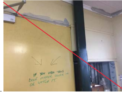
PHOTO NO.: J154900-001-PHOTO022 RESULT: ASBESTOS - POSITIVE BUILDING/LEVEL: ADMINISTRATION BUILDING - GROUND LEVEL ROOM/LOCATION: WASTE SERVICES OFFICE - KEY RETURN AREA - SOUTH FEATURE/MATERIAL: WALL - FIBRE CEMENT SHEETING SAMPLE NO.: J154900-001-026
