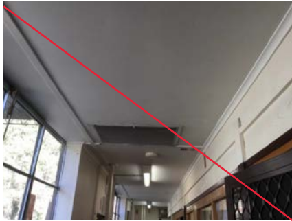
PHOTO NO.: J154900-001-PHOTO006 RESULT: ASBESTOS - POSITIVE BUILDING/LEVEL: ADMINISTRATION BUILDING - GROUND LEVEL ROOM/LOCATION: HALLWAY - SOUTHERN OFFICE - THROUGHOUT FEATURE/MATERIAL: CEILING - FIBRE CEMENT SHEETING SAMPLE NO.: PREVIOUSLY SAMPLED REGIONAL ENVIROSCIENCE B17336-S10
