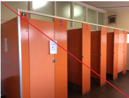
PHOTO NO.: J154900-001-PHOTO131 RESULT: ASBESTOS - POSITIVE BUILDING/LEVEL: AMENITIES BUILDING - GROUND LEVEL ROOM/LOCATION: MALE TOILET - WEST FEATURE/MATERIAL: TOILET CUBICLE - COMPRESSED CEMENT SHEETING SAMPLE NO.: PREVIOUSLY SAMPLED REGIONAL ENVIROSCIENCE B17336-S15
