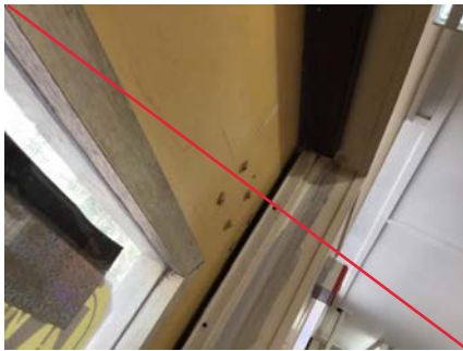
PHOTO NO.: J154900-001-PHOTO035 RESULT: ASBESTOS - POSITIVE BUILDING/LEVEL: ADMINISTRATION BUILDING - GROUND LEVEL ROOM/LOCATION: HALLWAY - SOUTHERN OFFICE - VARIOUS THROUGHOUT FEATURE/MATERIAL: WALL - FIBRE CEMENT SHEETING SAMPLE NO.: PREVIOUSLY SAMPLED REGIONAL ENVIROSCIENCE B17336-S09
