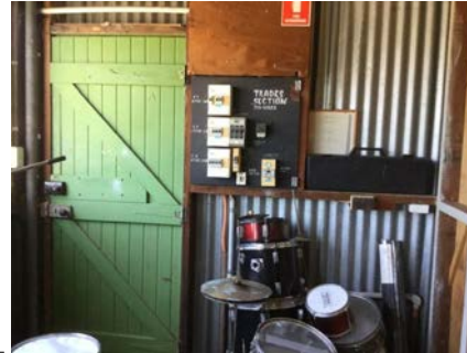
PHOTO NO.: J154900-001-PHOTO062 RESULT: ASBESTOS - NEGATIVE BUILDING/LEVEL: GARDENERS SHED - GROUND LEVEL ROOM/LOCATION: LUNCH AREA - SOUTHEAST FEATURE/MATERIAL: ELECTRICAL - SWITCH BOARD - COMPRESSED BITUMINOUS ELECTRICAL PANEL SAMPLE NO.: J154900-001-034
