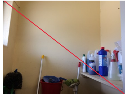
PHOTO NO.: J154900-001-PHOTO138 RESULT: ASBESTOS - POSITIVE BUILDING/LEVEL: AMENITIES BUILDING - GROUND LEVEL ROOM/LOCATION: CLEANER ROOM (WITHIN MALE TOILET) - WEST FEATURE/MATERIAL: WALL - FIBRE CEMENT SHEETING SAMPLE NO.: J154900-001-020
