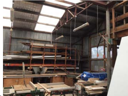
PHOTO NO.: J154900-001-PHOTO081 RESULT: BUILDING/LEVEL: TRADES SHED - GROUND LEVEL ROOM/LOCATION: MAIN SHED - VARIOUS THROUGHOUT FEATURE/MATERIAL: NON-HAZARDOUS FEATURE - NON-HAZARDOUS MATERIAL SAMPLE NO.: -
