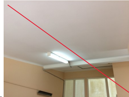
PHOTO NO.: J154900-001-PHOTO145 RESULT: ASBESTOS - PRESUMED POSITIVE BUILDING/LEVEL: AMENITIES BUILDING - LEVEL ONE ROOM/LOCATION: FEMALE CHANGE ROOM - THROUGHOUT FEATURE/MATERIAL: CEILING - FIBRE CEMENT SHEETING SAMPLE NO.: SIMILAR TO: J154900-001-006
