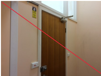
PHOTO NO.: J154900-001-PHOTO151 RESULT: ASBESTOS - POSITIVE BUILDING/LEVEL: AMENITIES BUILDING - LEVEL ONE ROOM/LOCATION: ENTRY - FEMALE TOILET/SHOWER/CHANGE ROOM - EAST FEATURE/MATERIAL: WALL - FIBRE CEMENT SHEETING SAMPLE NO.: J154900-001-008
