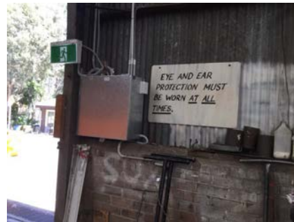
PHOTO NO.: J154900-001-PHOTO048 RESULT: ASBESTOS - NEGATIVE BUILDING/LEVEL: ADMINISTRATION BUILDING - GROUND LEVEL ROOM/LOCATION: RMT SHED - SOUTHWEST FEATURE/MATERIAL: ELECTRICAL - SWITCH BOARD - DUST SAMPLE NO.: J154900-001-032
