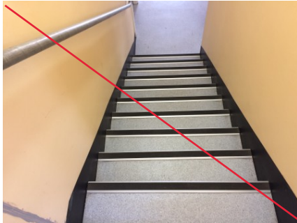
PHOTO NO.: J154900-001-PHOTO162 RESULT: ASBESTOS - NEGATIVE BUILDING/LEVEL: AMENITIES BUILDING - GROUND LEVEL ROOM/LOCATION: STAIRWELL TO LUNCH ROOM - VARIOUS THROUGHOUT FEATURE/MATERIAL: SKIRTING - SHEET VINYL & ADHESIVE SAMPLE NO.: PREVIOUSLY SAMPLED REGIONAL ENVIROSCIENCE B17336-S33
