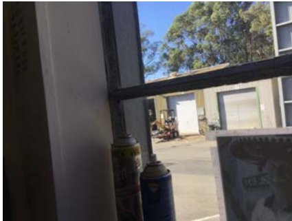
PHOTO NO.: J154900-001-PHOTO020 RESULT: ASBESTOS - NEGATIVE BUILDING/LEVEL: ADMINISTRATION BUILDING - GROUND LEVEL ROOM/LOCATION: WASTE SERVICES OFFICE - HALLWAY - SOUTH FEATURE/MATERIAL: WINDOW FRAMES - PUTTY SAMPLE NO.: J154900-001-025
