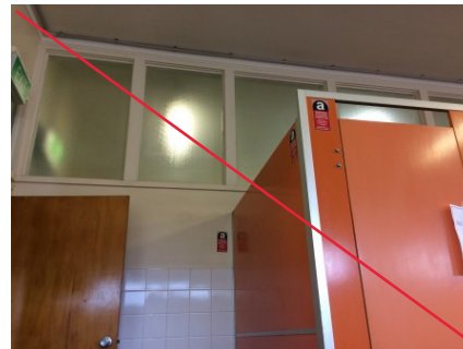
PHOTO NO.: J154900-001-PHOTO136 RESULT: ASBESTOS - POSITIVE BUILDING/LEVEL: AMENITIES BUILDING - GROUND LEVEL ROOM/LOCATION: MALE TOILET - WEST FEATURE/MATERIAL: WALL - FIBRE CEMENT SHEETING SAMPLE NO.: J154900-001-018
