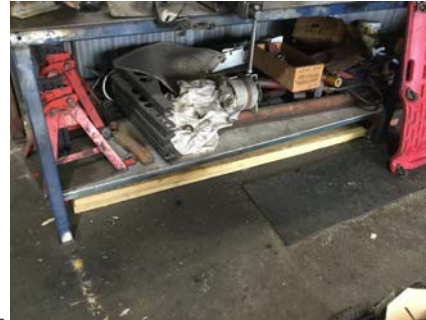
PHOTO NO.: J154900-001-PHOTO106 RESULT: ASBESTOS - NEGATIVE BUILDING/LEVEL: WORKSHOP - GROUND LEVEL ROOM/LOCATION: MAIN WORKSHOP - SOUTH FEATURE/MATERIAL: BENCH TOP - FIBRE CEMENT SHEETING SAMPLE NO.: J154900-001-043
