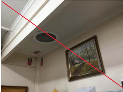
PHOTO NO.: J154900-001-PHOTO029 RESULT: ASBESTOS - PREVIOUSLY SAMPLED POSITIVE BUILDING/LEVEL: ADMINISTRATION BUILDING - GROUND LEVEL ROOM/LOCATION: WASTE SERVICES OFFICE - KITCHENETTE - THROUGHOUT FEATURE/MATERIAL: CEILING - FIBRE CEMENT SHEETING SAMPLE NO.: PREVIOUSLY SAMPLED REGIONAL ENVIROSCIENCE B17336-S10
