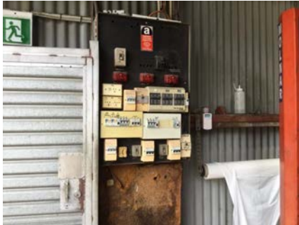
PHOTO NO.: J154900-001-PHOTO105 RESULT: ASBESTOS - PRESUMED POSITIVE BUILDING/LEVEL: WORKSHOP - GROUND LEVEL ROOM/LOCATION: MAIN WORKSHOP - NORTHEAST FEATURE/MATERIAL: ELECTRICAL - SWITCH BOARD - COMPRESSED BITUMINOUS ELECTRICAL PANEL SAMPLE NO.: SIMILAR TO: J154900-001-038
