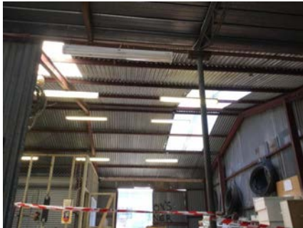
PHOTO NO.: J154900-001-PHOTO058 RESULT: BUILDING/LEVEL: GARDENERS SHED - GROUND LEVEL ROOM/LOCATION: ALL AREAS - VARIOUS THROUGHOUT FEATURE/MATERIAL: NON-HAZARDOUS FEATURE - NON-HAZARDOUS MATERIAL SAMPLE NO.: -
