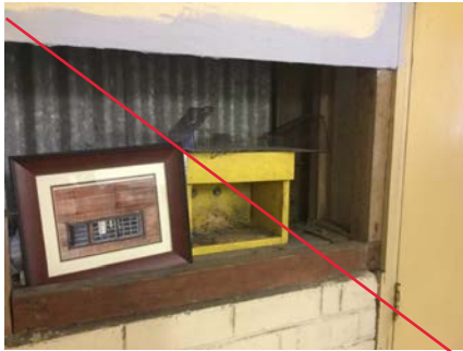
PHOTO NO.: J154900-001-PHOTO023 RESULT: ASBESTOS - PRESUMED POSITIVE BUILDING/LEVEL: ADMINISTRATION BUILDING - GROUND LEVEL ROOM/LOCATION: WASTE SERVICES OFFICE - KEY RETURN AREA - SOUTH FEATURE/MATERIAL: WALL - FIBRE CEMENT SHEETING SAMPLE NO.: SIMILAR TO: J154900-001-026
