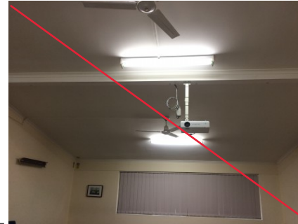
PHOTO NO.: J154900-001-PHOTO154 RESULT: ASBESTOS - PRESUMED POSITIVE BUILDING/LEVEL: AMENITIES BUILDING - LEVEL ONE ROOM/LOCATION: CONFERENCE ROOM - THROUGHOUT FEATURE/MATERIAL: CEILING - FIBRE CEMENT SHEETING SAMPLE NO.: SIMILAR TO: J154900-001-006
