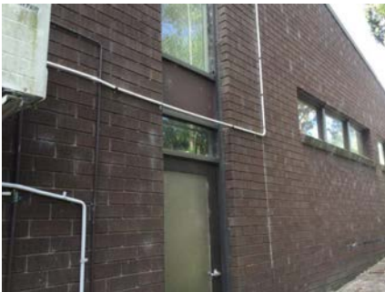
PHOTO NO.: J154900-001-PHOTO113 RESULT: ASBESTOS - POSITIVE BUILDING/LEVEL: AMENITIES BUILDING - GROUND LEVEL ROOM/LOCATION: EXTERIOR - NORTH & SOUTH FEATURE/MATERIAL: INFILL PANELS - FIBRE CEMENT SHEETING SAMPLE NO.: PREVIOUSLY SAMPLED REGIONAL ENVIROSCIENCE B17336-S13
