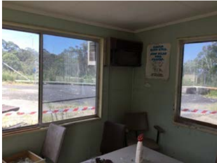
PHOTO NO.: J154900-001-PHOTO074 RESULT: ASBESTOS - NEGATIVE BUILDING/LEVEL: TRADES SHED - GROUND LEVEL ROOM/LOCATION: MEALS ROOM - THROUGHOUT FEATURE/MATERIAL: WALL - FIBRE CEMENT SHEETING SAMPLE NO.: J154900-001-040
