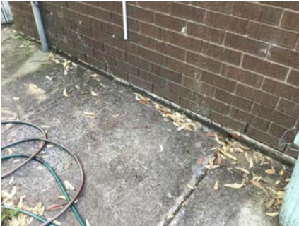
PHOTO NO.: J154900-001-PHOTO110 RESULT: ASBESTOS - NEGATIVE BUILDING/LEVEL: AMENITIES BUILDING - GROUND LEVEL ROOM/LOCATION: EXTERIOR - VARIOUS THROUGHOUT FEATURE/MATERIAL: EXPANSION JOINT - MASTIC SEALANT SAMPLE NO.: J154900-001-044
