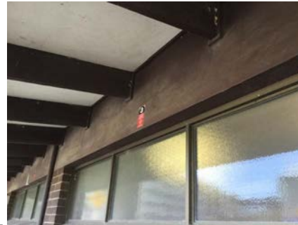
PHOTO NO.: J154900-001-PHOTO126 RESULT: ASBESTOS - POSITIVE BUILDING/LEVEL: AMENITIES BUILDING - ALL LEVELS ROOM/LOCATION: EXTERIOR - EAST & WEST FEATURE/MATERIAL: INFILL PANELS - FIBRE CEMENT SHEETING SAMPLE NO.: J154900-001-049
