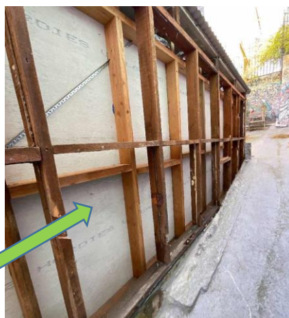
External, GF, Exterior, South West, Internal wall of lower ground floor - Fibre cement sheet, No Asbestos detected, 442261/AS02
