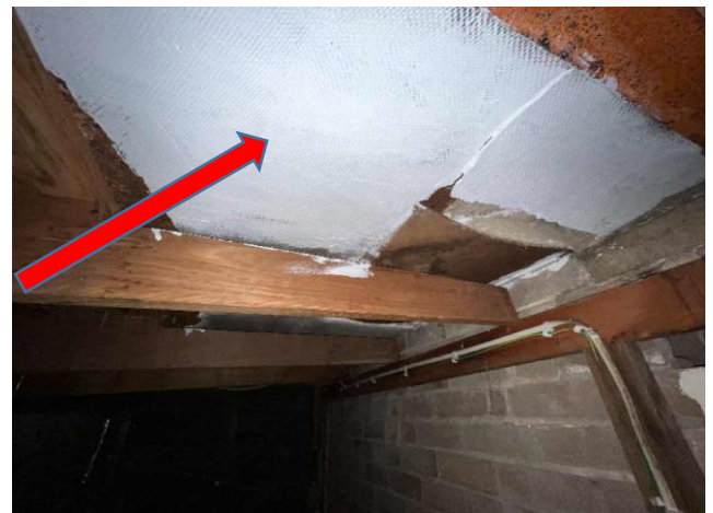
Internal, GF, Ceiling space, Formwork to underside of level 1 - Fibre cement sheet, Chrysotile asbestos detected, Previously sampled B17455S23
