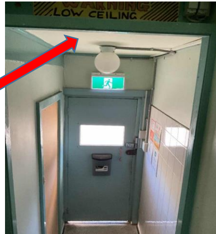
Internal, L1, Internal hallway, North East, Ceiling of entry to level 1 - Fibre cement sheet, Chrysotile and Amosite asbestos detected, Previously sampled B17455S27
