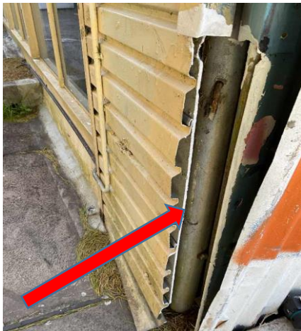
External, GF, Exterior, West, Wall - FC Cladding beneath metal cladding - Fibre cement sheet, Chrysotile asbestos detected, Previously sampled B17455S06
