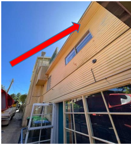
External, L1, Exterior, West, Eaves - Fibre cement sheet, Chrysotile asbestos detected, Similar to Previously sampled B17455S09
