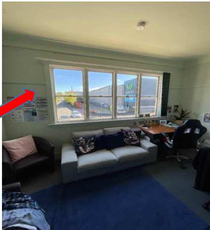
Internal, L1, North east office, North, Wall infills on left and right of window - Fibre cement sheet, Contains Chrysotile and Amosite Asbestos, 442261/AS01
