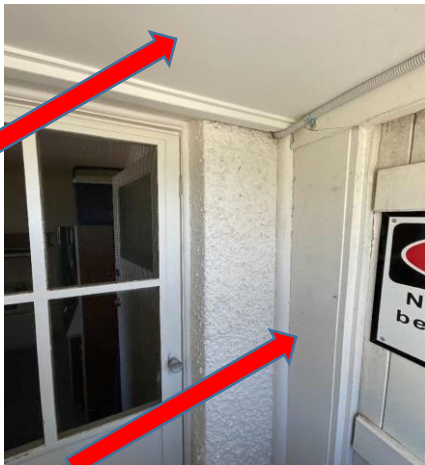
Internal, L1, External south east porch, South West, Ceiling and walls - Fibre cement sheet, Chrysotile, Amosite and Crocidolite asbestos detected, Previously sampled B17455S29
