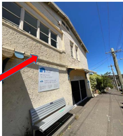
External, GF, Exterior, External yellow paint to all surfaces - Yellow - Topcoat, Lead based paint system (0.2%w/w), Previous sampled 17455-S02
