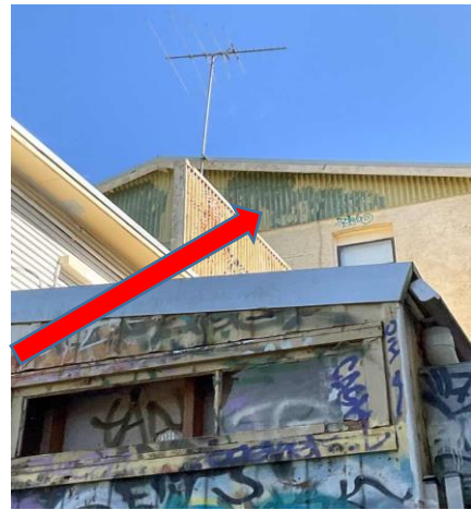
External, L1, Exterior, Northeast and southeast gable ends - Fibre cement sheet, Assumed positive for asbestos, Assumed positive
