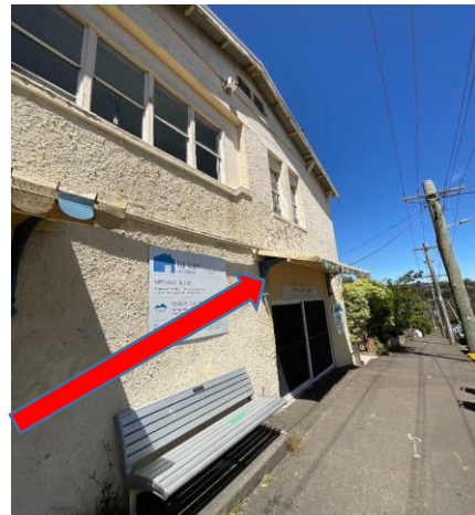
External, GF, Exterior, North East, Wrought iron brackets - Blue - Topcoat, Lead based paint system (9.5%w/w), Previously sampled 17455-S03
