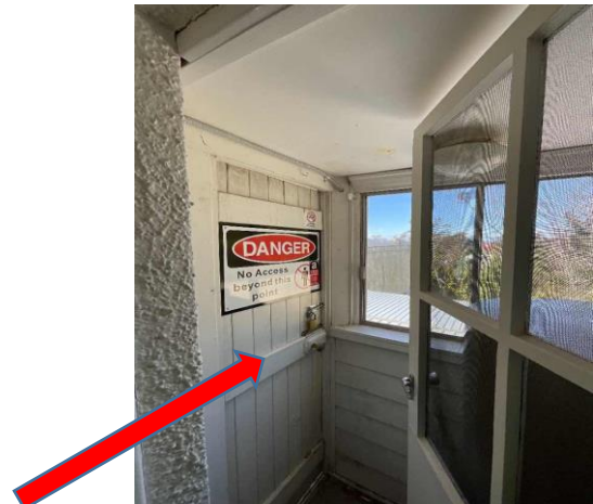
Internal, L1, External south east porch, Ceiling, walls, timber trim and doors - Cream - Topcoat, Lead based paint system (0.2%w/w), Previously sampled 17455-S25
