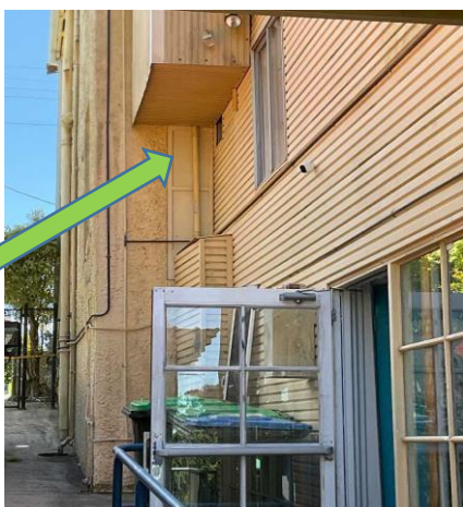
External, L1, Exterior, South West, Corner infill - Fibre cement sheet, No asbestos detected, Previously sampled B17455S05
