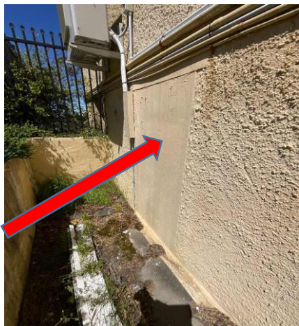
External, GF, Exterior, East, Door infill - Fibre cement sheet, Chrysotile asbestos detected, Similar to previously sampled B17455S10
