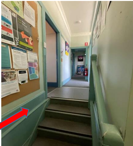
Internal, L1, Interior, On timber trim throughout level 1 - Blue & light blue - Topcoat, Lead based paint system (0.3%w/w), Previously sampled 17455-S31
