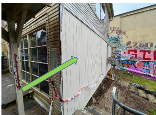
External, GF, Exterior, South and east elevation - Fibre cement sheet, No asbestos assumed, -
