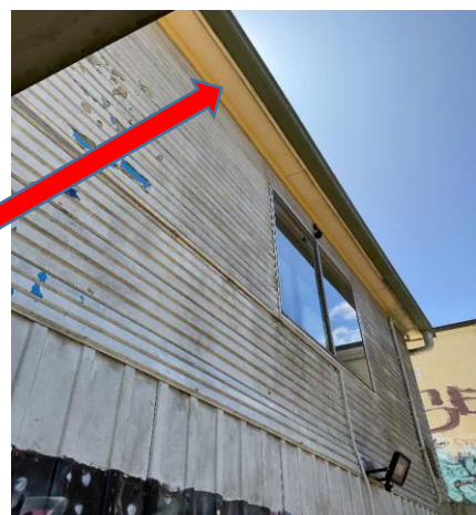
External, L1, Exterior, South, Eaves - Fibre cement sheet, Chrysotile asbestos detected, Previously sampled B17455S09
