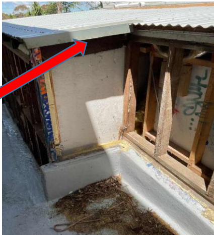
External, GF, Exterior, South and East elevation wall cavities - Fibre cement, Presumed asbestos containing, Similar to 442261/AS01
