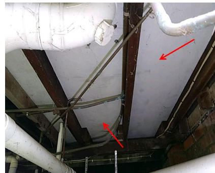
Photo No: 210823-121504 Result: Asbestos - Positive Location-Level: Exterior - Ground Floor Room-Location: NE elevation of the building - flooring Feature-Material: Moulded FC Item No - Risk Rating: 27 - Low
