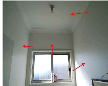
Photo No: 210811-100703 Result: Asbestos - Negative Location-Level: Interior - Ground Floor Room-Location: Toilet - internal walls and ceiling Feature-Material: FC sheeting
