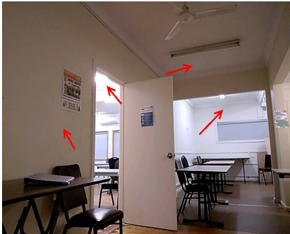
Photo No: 210811-095456 Result: Asbestos - Negative Location-Level: Interior - Ground Floor Room-Location: Meeting room and studio - Internal walls, dividing wall and ceilings Feature-Material: Plaster-like material
