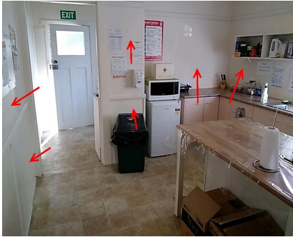
Photo No: 210811-103311 Result: Asbestos - Presumed Negative Location-Level: Interior - Ground Floor Room-Location: Kitchen Feature-Material: Plaster-like material
