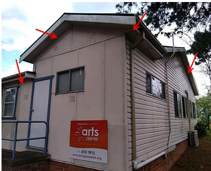
Photo No: 210823-120443 Result: Asbestos - Presumed Positive Location-Level: Exterior - Ground Floor Room-Location: Western and northern elevation of the building - eaves Feature-Material: FC sheeting Item No - Risk Rating: 23 - Low
