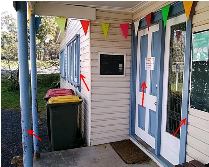
Photo No: 210811-111218 Result: Lead in Paint - Positive Location-Level: Exterior - Ground Floor Room-Location: All elevation of the building - door frames, windows frames, handrail and column Feature-Material: Lower colour paint system Item No - Risk Rating: 16 - N/A
