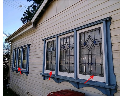
Photo No: 210811-111328 Result: Asbestos - Negative Location-Level: Exterior - Ground Floor Room-Location: Southern elevation of the building - windows frames sealants Feature-Material: Mastic-like material
