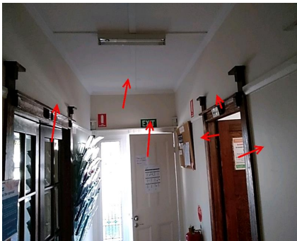
Photo No: 210811-104916 Result: Asbestos - Presumed Negative Location-Level: Interior - Ground Floor Room-Location: Entry lobby - internal, dividing walls and ceiling Feature-Material: Plaster-like material
