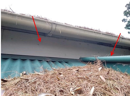
Photo No: 210823-120823 Result: Asbestos - Presumed Negative Location-Level: Exterior - Ground Floor Room-Location: Northern elevation of the building- infill panels above external walls Feature-Material: Similar to 03
