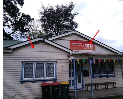
Photo No: 210823-123900 Result: Asbestos - Presumed Positive Location-Level: Exterior - Ground Floor Room-Location: Southern and northern elevation of the building - gable Feature-Material: FC sheeting Item No - Risk Rating: 22 - Low
