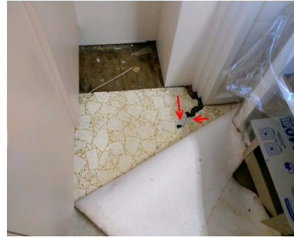
Photo No: 210915-090207 Result: Asbestos - Positive Location-Level: Interior - Ground Floor Room-Location: Kitchen - Floor covering Feature-Material: (a) vinyl sheeting and backing material. (b) adhesive Item No - Risk Rating: 29 - High
