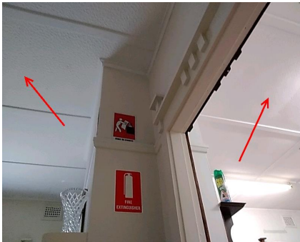
Photo No: 210811-104056 Result: Asbestos - Presumed Negative Location-Level: Interior - Ground Floor Room-Location: Kitchen and office - ceilings Feature-Material: Plaster-like material
