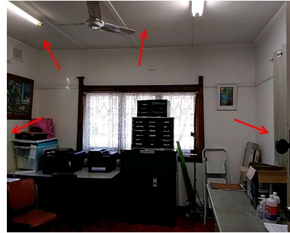
Photo No: 210811-103648 Result: Asbestos - Presumed Negative Location-Level: Interior - Ground Floor Room-Location: Office - internal walls and ceiling Feature-Material: Plaster-like material
