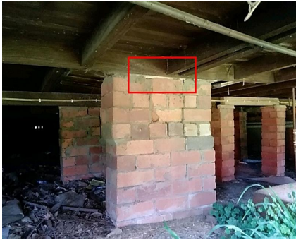
Photo No: 210811-111734 Result: Asbestos - Positive Location-Level: Exterior - Ground Floor Room-Location: All elevation of the building - packer to support beams Feature-Material: FC sheeting Item No - Risk Rating: 21 - Low
