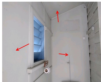
Photo No: 210811-111626 Result: Asbestos - Positive Location-Level: Exterior - Ground Floor Room-Location: External toilet - internal walls and ceiling Feature-Material: FC sheeting Item No - Risk Rating: 20 - Low
