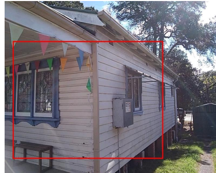
Photo No: 210811-111231 Result: Lead in Paint - Positive Location-Level: Exterior - Ground Floor Room-Location: All elevation of the building - external walls Feature-Material: Lower colour paint system Item No - Risk Rating: 17 - N/A
