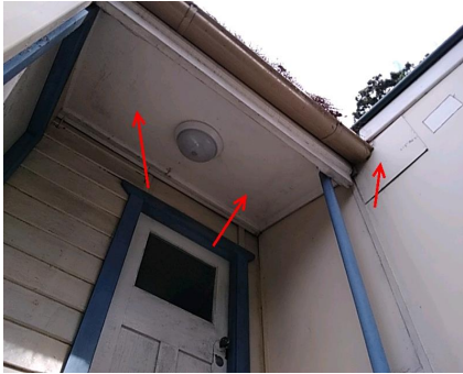
Photo No: 210823-124259 Result: Asbestos - Presumed Positive Location-Level: Exterior - Ground Floor Room-Location: Northern elevation of the building (next to rear entrance) - infill panel and eaves Feature-Material: FC sheeting Item No - Risk Rating: 28 - Low
