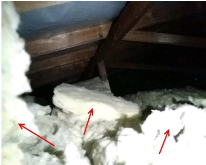
Photo No: 210811-095033 Result: SMF - Presumed Positive Location-Level: Interior - Roof Room-Location: Roof - insulation Feature-Material: Insulation Item No - Risk Rating: 1 - N/A
