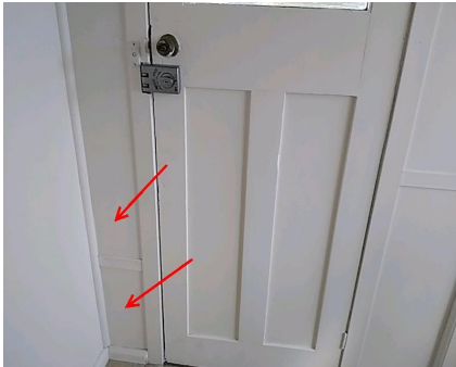
Photo No: 210811-101411 Result: Asbestos - Negative Location-Level: Interior - Ground Floor Room-Location: Northern exit - infill panels next to exit door Feature-Material: FC sheeting
