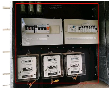
Photo No: 210823-120217 Result: Asbestos - Presumed Positive Location-Level: Exterior - Ground Floor Room-Location: SE elevation of the building - electrical distribution backing board Feature-Material: Bituminous-like material Item No - Risk Rating: 24 - Low
