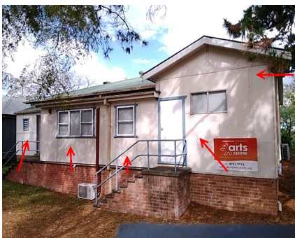
Photo No: 210823-124111 Result: Asbestos - Positive Location-Level: Exterior - Ground Floor Room-Location: Northern elevation of the building - external walls Feature-Material: FC sheeting Item No - Risk Rating: 19 - Low
