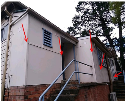
Photo No: 210823-121005 Result: Asbestos - Positive Location-Level: Exterior - Ground Floor Room-Location: Eastern, western and northern elevation of the building - walls corner cover strip Feature-Material: Moulded FC Item No - Risk Rating: 26 - Low
