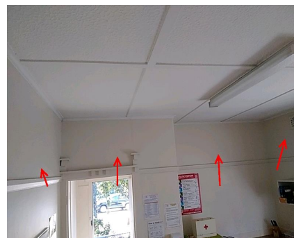
Photo No: 210811-102927 Result: Asbestos - Negative Location-Level: Interior - Ground Floor Room-Location: Kitchen - upper section of internal and dividing wall Feature-Material: FC sheeting
