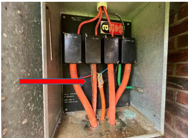
External, GF, Exterior, External cabinet - link panel 1 - Electrical backing board, Suspected Asbestos, Assumed positive
