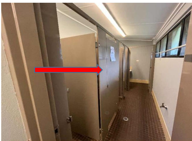
Internal, GF, Men's Bathroom, Toilet Partition Walls - Fibreboard, Chrysotile Asbestos, 37272-6
