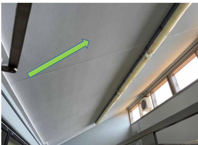
Internal, GF, Women's Bathroom, Ceiling Lining - Fibreboard, Assumed Negative, Similar to 37272-5
