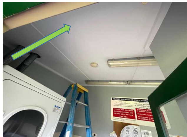
Internal, GF, Laundry, Laundry Ceiling Lining - Fibreboard, Assumed Negative, Similar to 37272-5
