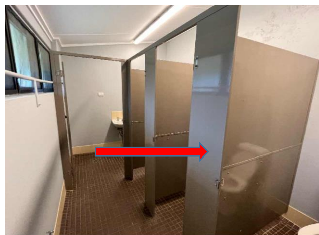
Internal, GF, Women's Bathroom, Toilet Partition Walls - Fibreboard, Assumed Positive, Similar to Sample 37272-6
