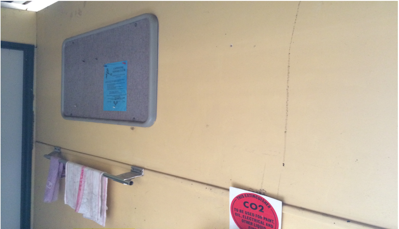
Photo 24: D00156 – Tennis Clubhouse – Explorers Road, Lapstone – Kitchenette – Wall cladding.
