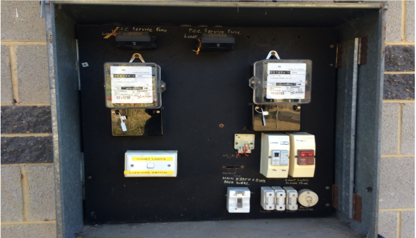
Photo 23: D00156 – Tennis Clubhouse – Explorers Road, Lapstone – Switchboard – Electrical backing board.
