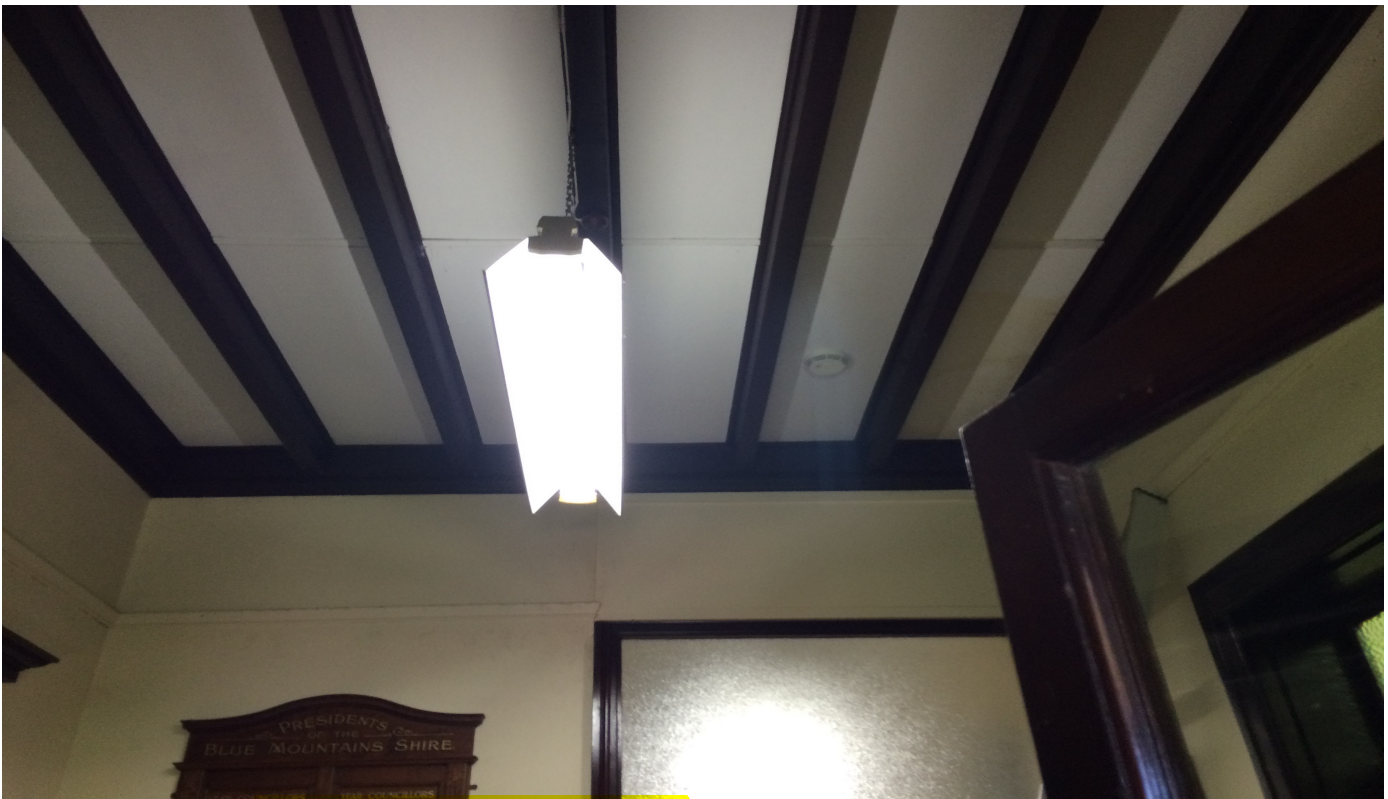
Photo 26: D00048 – Lawson Council Building and Library – 1 Loftus Street, Lawson – Upper level – Entry ceiling lining.
