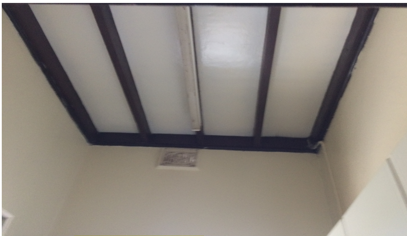
Photo 28: D00048 – Lawson Council Building and Library – 1 Loftus Street, Lawson – Upper level – Rear kitchenette – Ceiling lining.
