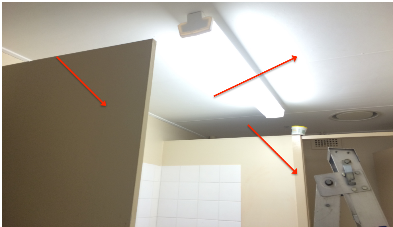
Photo 31: D00048 – Lawson Council Building and Library – 1 Loftus Street, Lawson – Lower level – Bathroom – Partition walls and ceiling lining.
