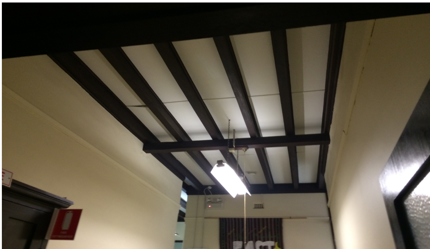
Photo 27: D00048 – Lawson Council Building and Library – 1 Loftus Street, Lawson – Example of Upper level – Ceiling throughout – Day care/ Hallway/ Offices/ Library.
