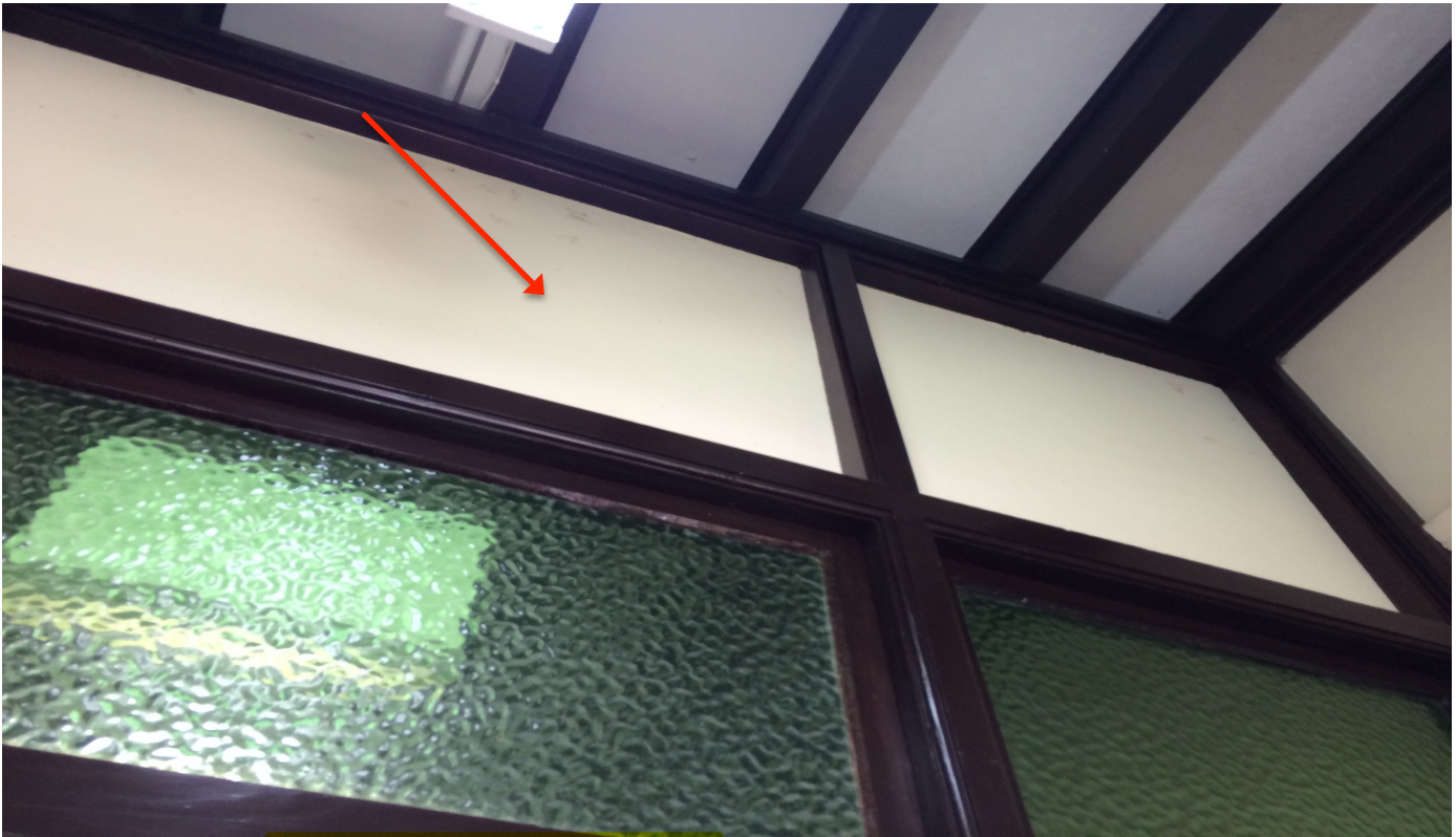
Photo 25: D00048 – Lawson Council Building and Library – 1 Loftus Street, Lawson – Upper level – Infill panels above entry windows.
