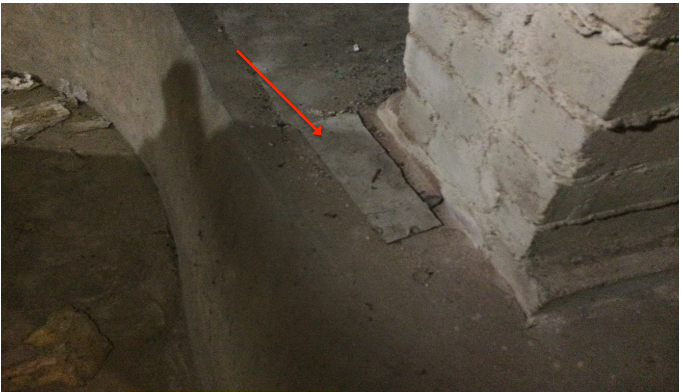
Photo 30: D00048 – Lawson Council Building and Library – 1 Loftus Street, Lawson – Lower level – Subfloor fragments.
