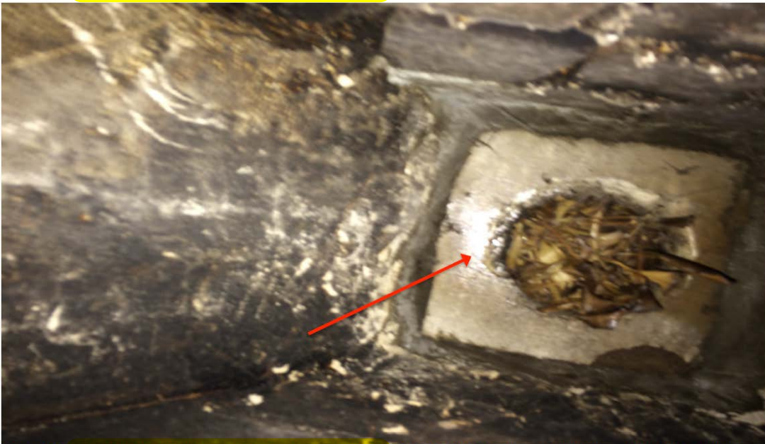
Photo 36: Heatherbrae House – 1 Benang Street, Lawson - Children's play area – Fireplace – Formwork around chimney.
