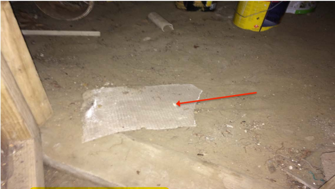
Photo 37: Heatherbrae House – 1 Benang Street, Lawson - Sub-floor – Redundant sheet.
