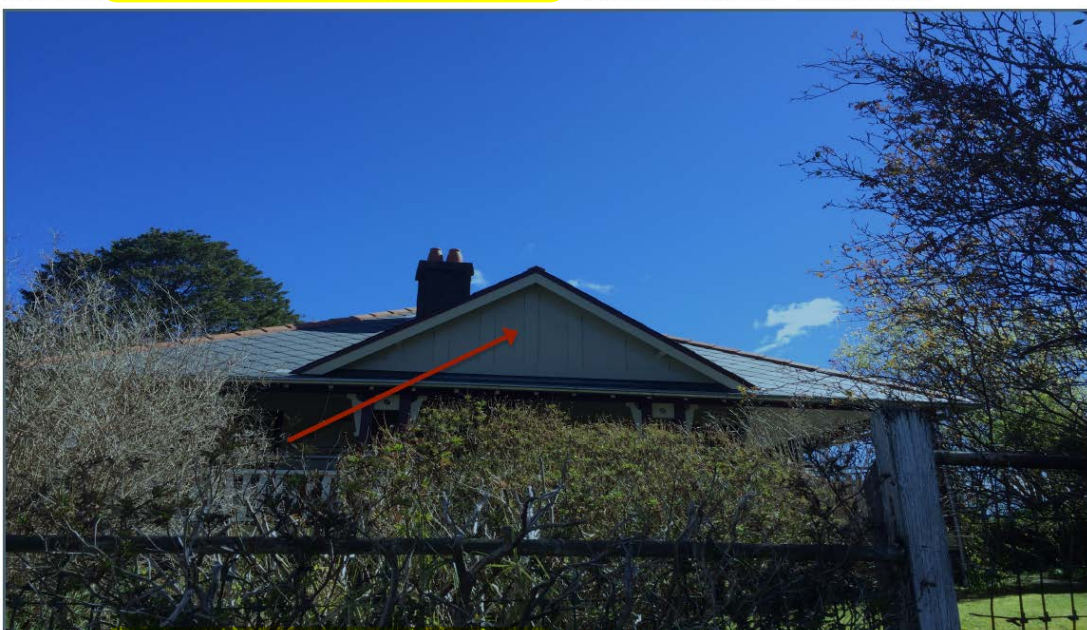
Photo 32: Heatherbrae House – 1 Benang Street, Lawson – Gable linings
