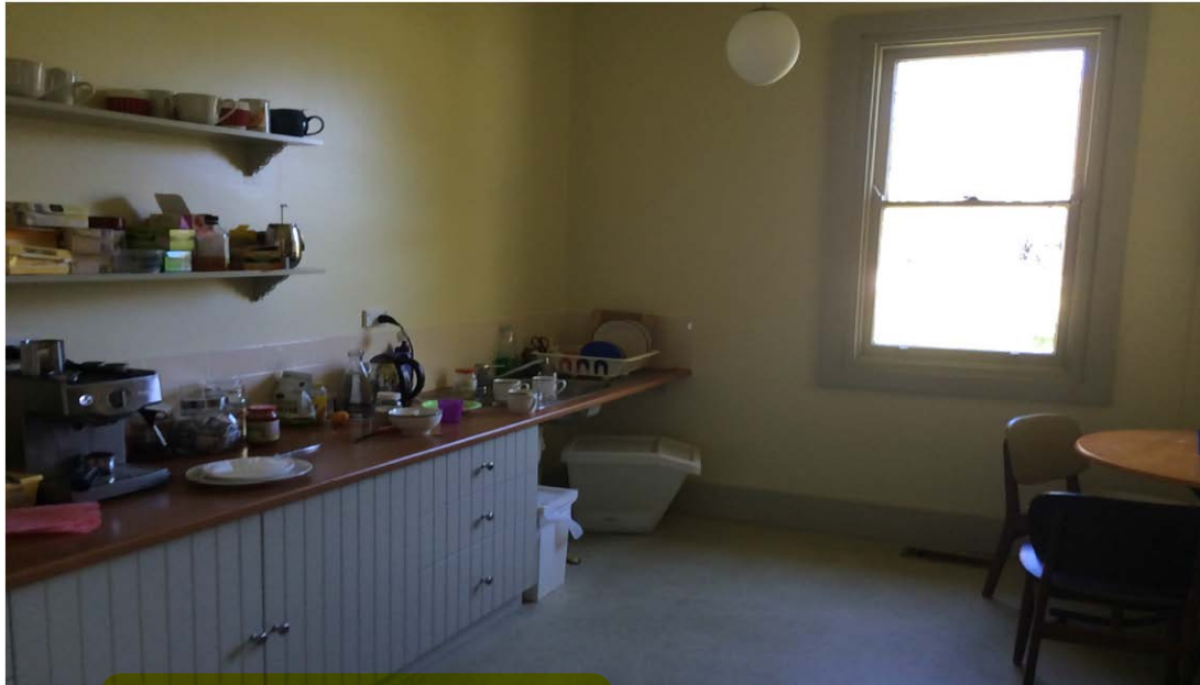
Photo 34: Heatherbrae House – 1 Benang Street, Lawson - Bathroom – Kitchen – Wall cladding.
