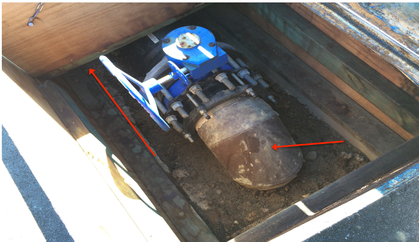
Photo 39: Lawson Swimming Pool – 2-16 St Bernards Drive, Lawson - Main inlet pipe. Continues underground after valve and polyurethane pipe – North of swimming pool.
