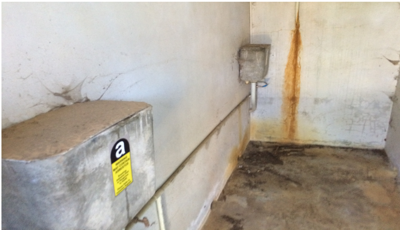
Photo 38: E00133 – Toilet Block - Lawson Swimming Pool – 2-16 St Bernards Drive, Lawson - Tank room – Cement tanks.
