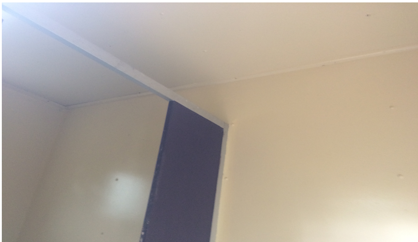
Photo 43: E00197 – Toilet Block - 12-14 The Avenue, Mount Wilson – Wall cladding and ceiling lining.
