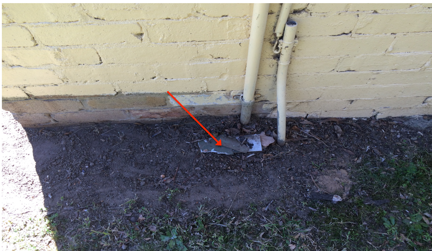
Photo 45: E00251 – Machinery Shed - 389-407 Great Western Highway, Springwood - Fragments under switchboard.
