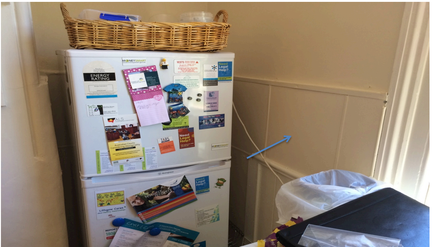
Photo 170: Asbestos cement sheet internal wall linings behind the fridge and on the northern perimeter wall in the Kitchen in the Katoomba Community Legal Centre.
