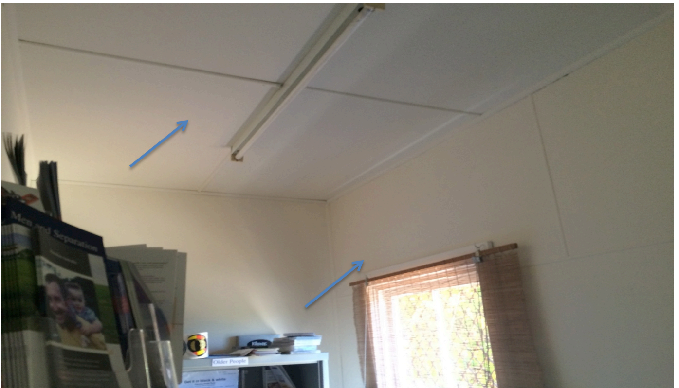
Photo 168: Asbestos cement sheet ceiling lining and internal walls of the north-eastern storeroom of the Katoomba Community Legal Centre.
