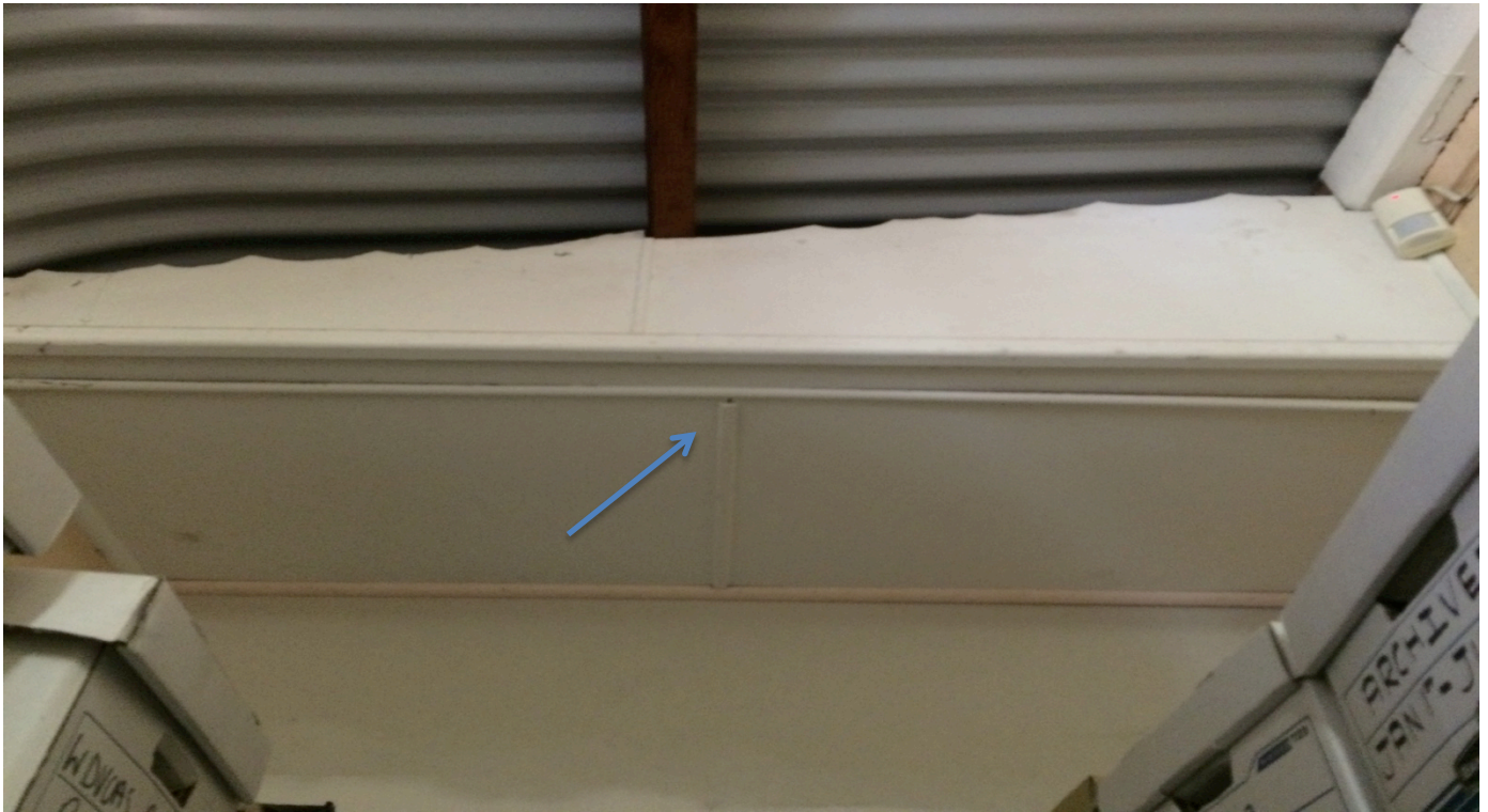
Photo 169: Asbestos cement sheet bulkhead lining Archive room in the Katoomba Community Legal Centre.
