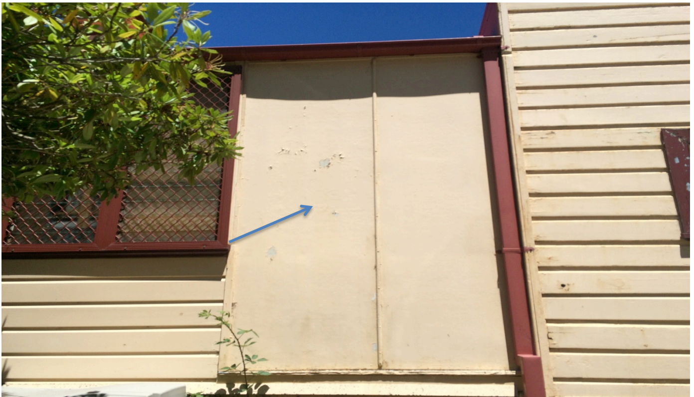
Photo 166: Asbestos cement sheet external wall panels on the northern perimeter of the Katoomba Community Legal Centre.
