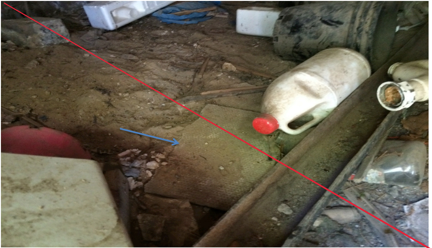
Photo 167: Asbestos cement sheet debris on the north-western area of the sub-floor of the Katoomba Community Legal Centre.
