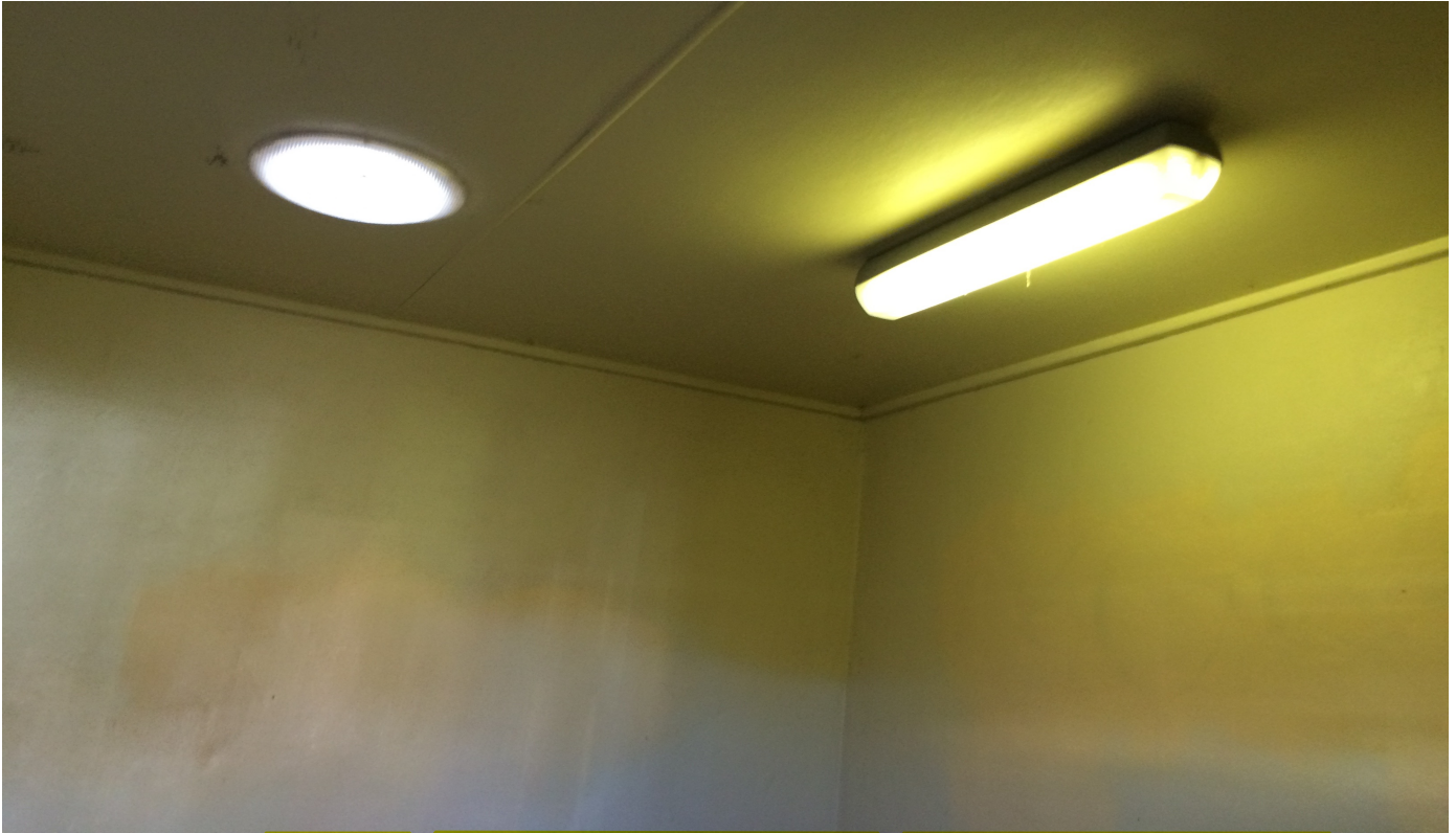
Photo 53: E00026 – Toilet Block - 19P Station Street, Wentworth Falls - Disabled bathroom – Ceiling lining.
