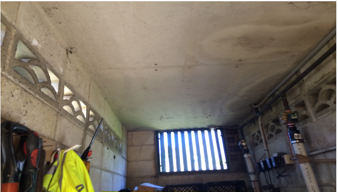
Photo 54: E00026 – Toilet Block - 19P Station Street, Wentworth Falls - Storage room.
