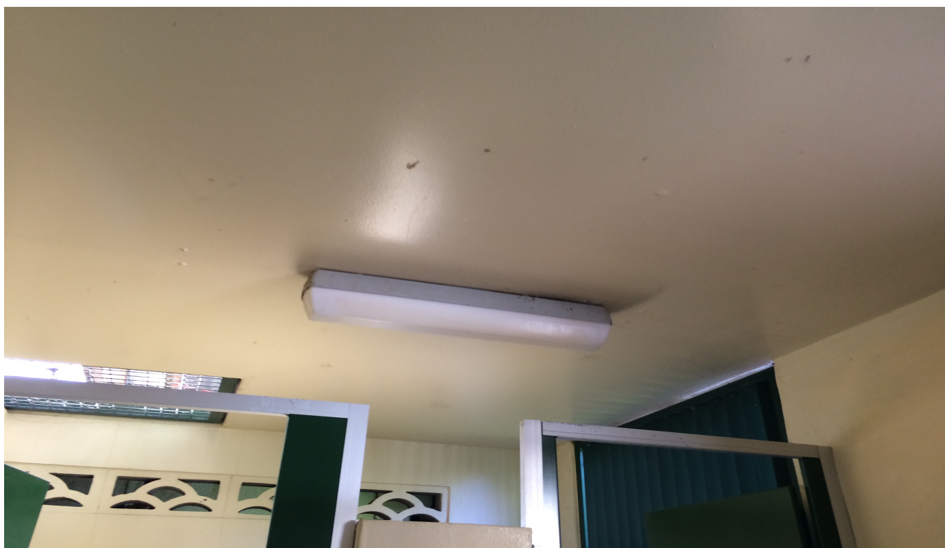
Photo 52: E00026 – Toilet Block - 19P Station Street, Wentworth Falls - Women's bathroom – Ceiling lining.
