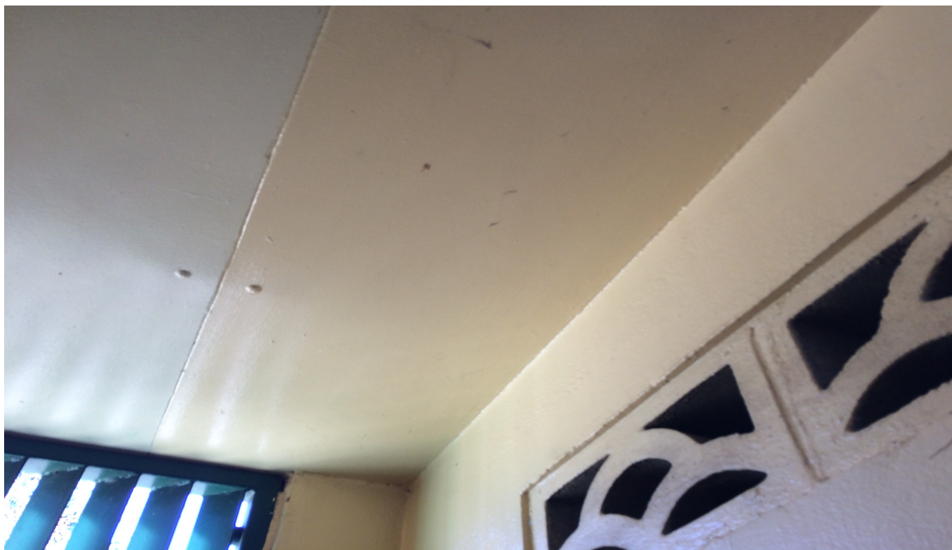
Photo 51: E00026 – Toilet Block - 19P Station Street, Wentworth Falls - Men's bathroom – Ceiling lining.
