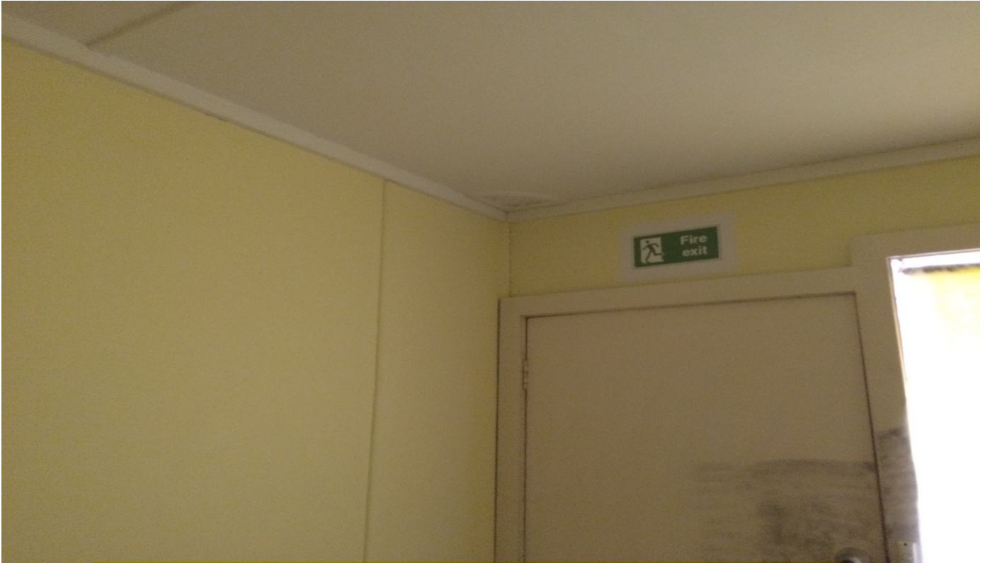
Photo 71: Cottage - 58-60 White Cross Road, Winmalee – Laundry – Wall cladding and ceiling lining.
