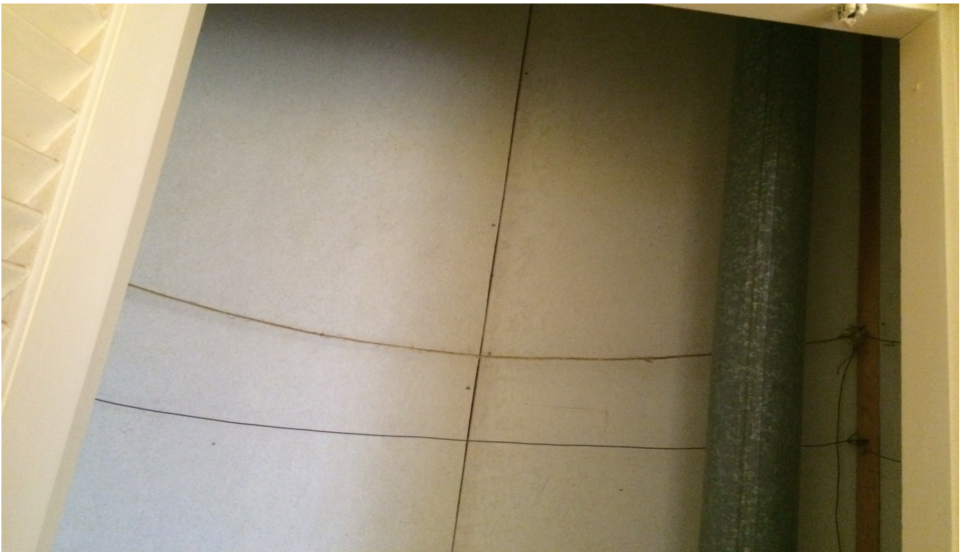
Photo 72: Cottage - 58-60 White Cross Road, Winmalee – Kitchen – Heater exhaust cupboard lining.
