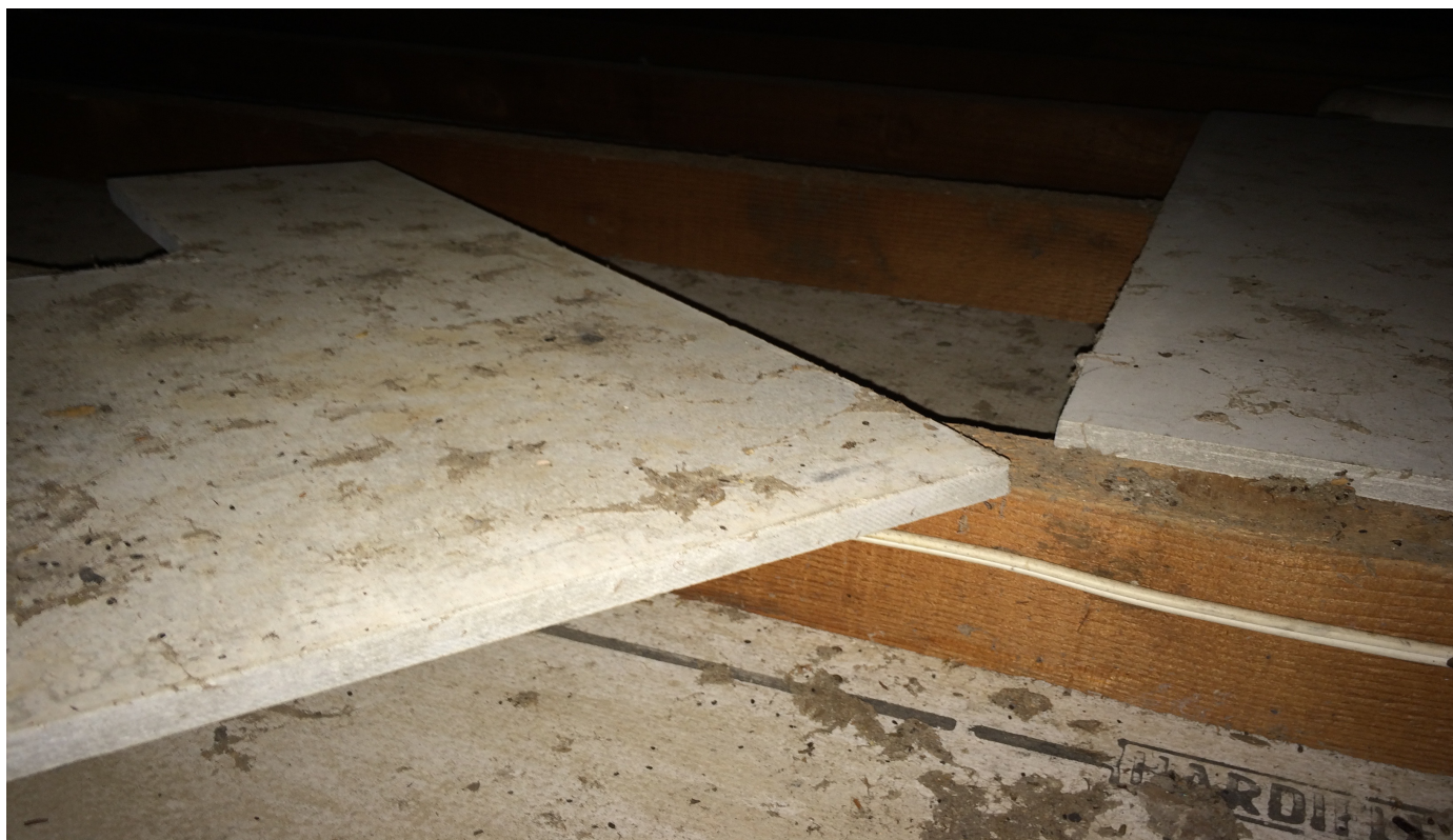
Photo 75: Cottage - 58-60 White Cross Road, Winmalee – Garage – Ceiling space – Cement slabs.
