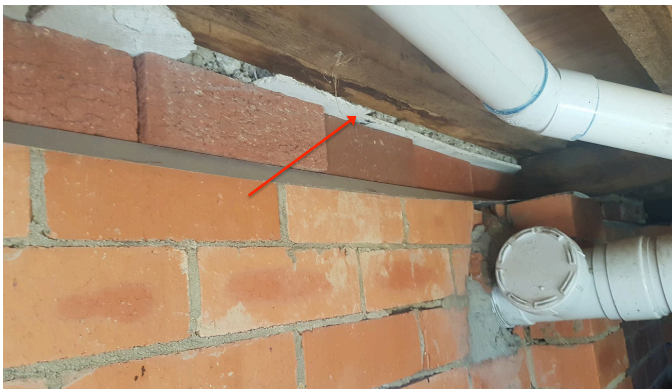
Photo 76: Cottage - 58-60 White Cross Road, Winmalee – Sub-floor – Form work above brickwork.
