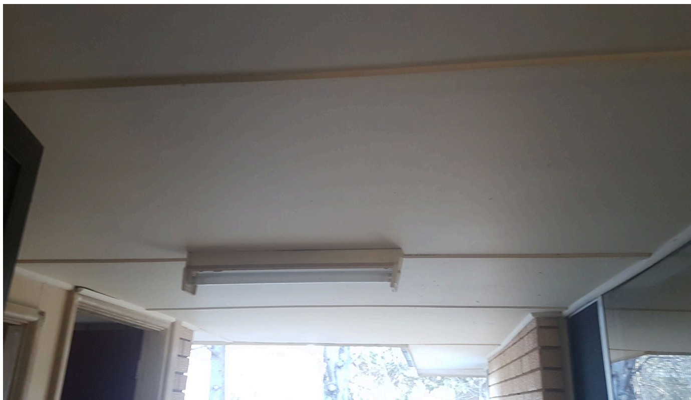
Photo 67: Cottage - 58-60 White Cross Road, Winmalee - Entry awning – Rear.
