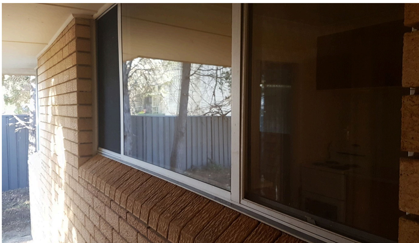
Photo 70: Cottage - 58-60 White Cross Road, Winmalee – Windows throughout.
