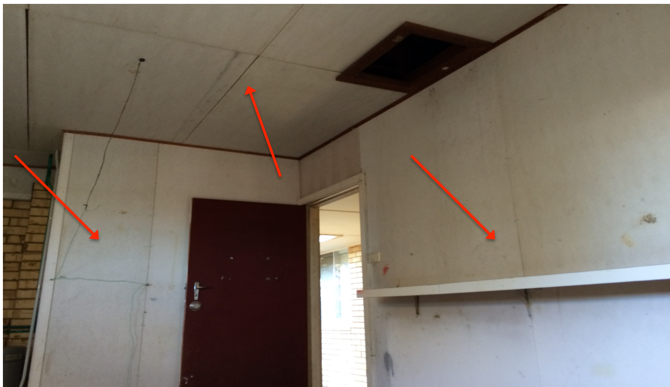
Photo 73: Cottage - 58-60 White Cross Road, Winmalee – Garage and adj. bathroom – Wall cladding and ceiling lining.
