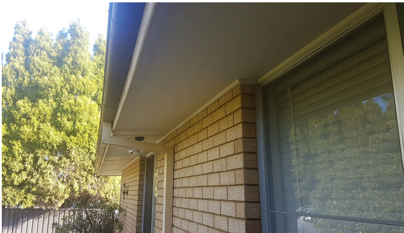
Photo 69: Cottage - 58-60 White Cross Road, Winmalee – Eave linings.
