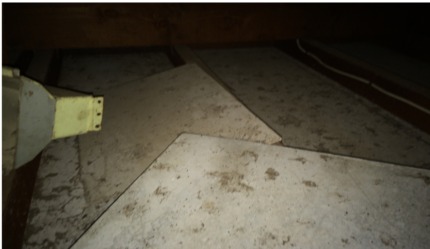
Photo 74: Cottage - 58-60 White Cross Road, Winmalee – Garage – Ceiling space - Redundant sheets.
