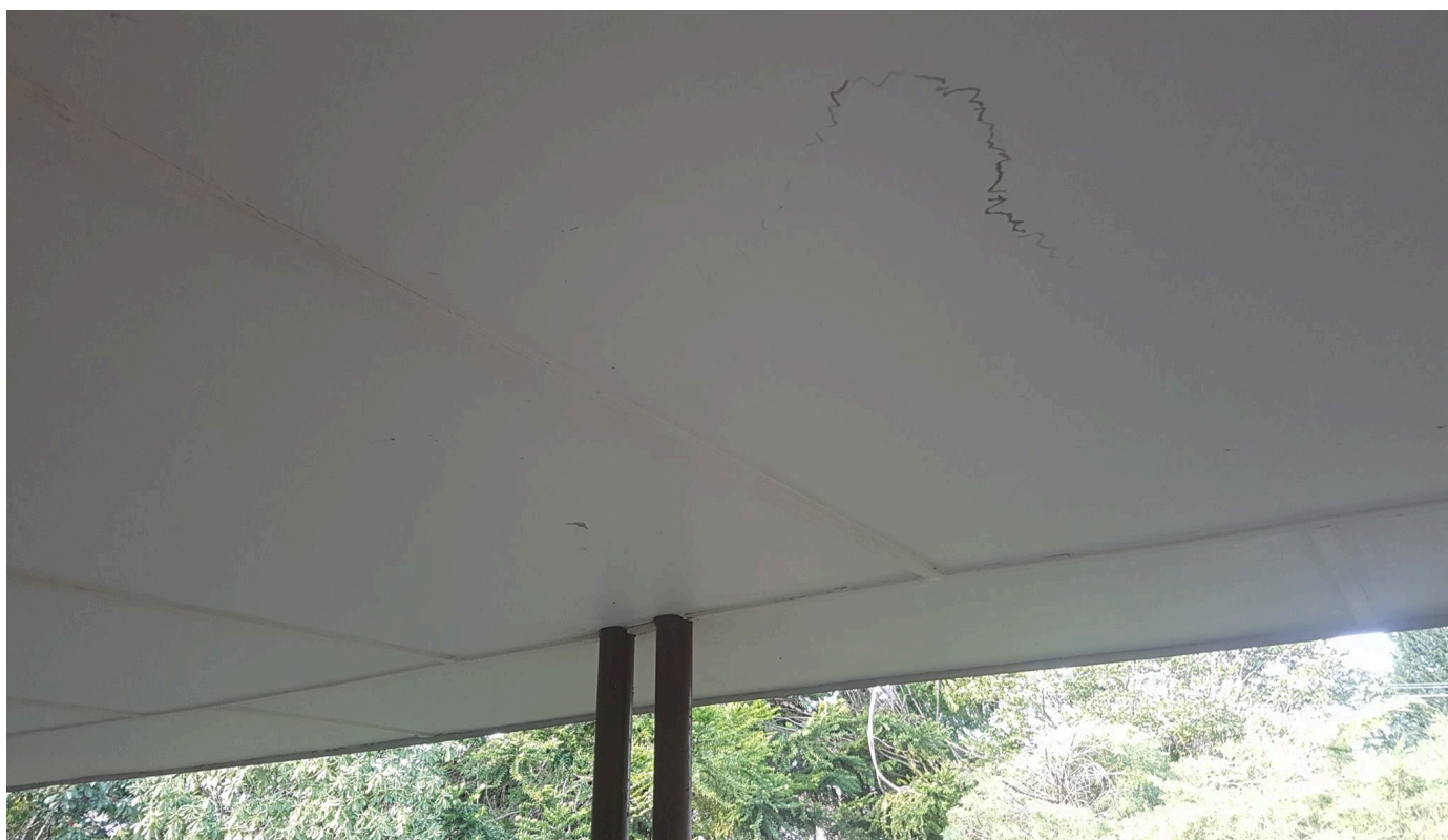
Photo 68: Cottage - 58-60 White Cross Road, Winmalee - Entry awning – Front.
