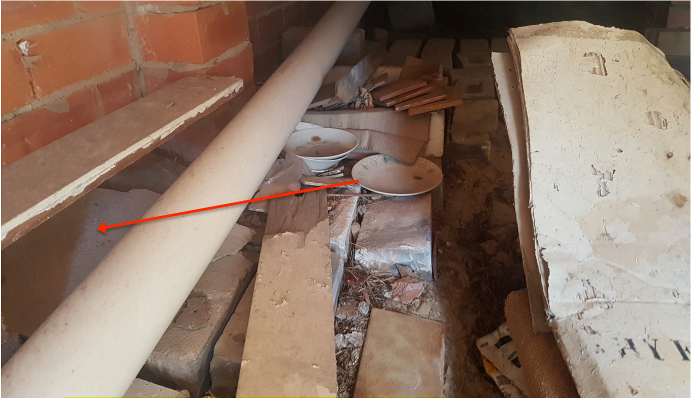
Photo 77: Cottage - 58-60 White Cross Road, Winmalee – Sub-floor –Fragments.
