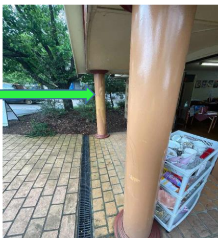
External, GF, Exterior, South, Entrance, Columns - Fibre cement pipe, No asbestos detected, 437014-AS04
