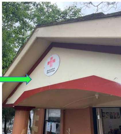
External, GF, Exterior, South, Entrance Gable End - Fibre Cement Sheet, Assumed Negative, 437014-AS03
