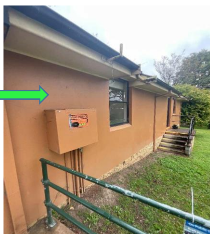
External, GF, Exterior, External walls - Orange - Topcoat, Lead Not Detected (<0.001%w/w), 437014-LP01
