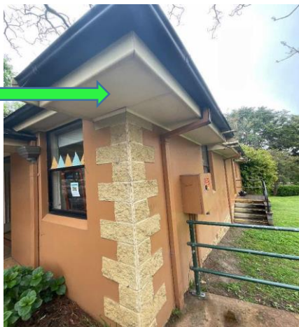
External, GF, Exterior, Eaves and fascia - Yellow - Topcoat, Lead Not Detected (0.003%w/w), 437014-LP02
