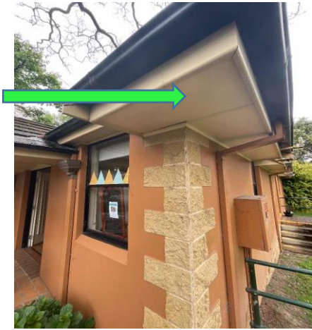
External, GF, Exterior, Perimeter Eave Linings - Fibre Cement Sheet, No Asbestos identified, 437014-AS02
