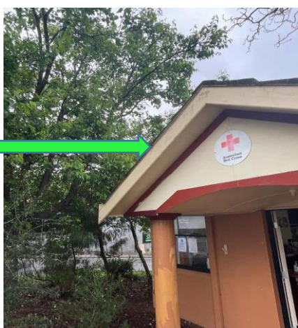
External, GF, Exterior, South, External Roof perimeter, Cloaked Verge Weather Strip - Fibre cement sheet, No Asbestos identified, 437014-
