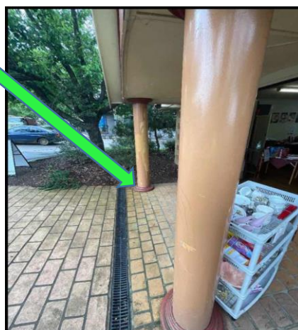
External, GF, Exterior, Entrance, top & bottom sheaths of column - Fibre cement, No Asbestos Detected, Similar to 437014-AS04
