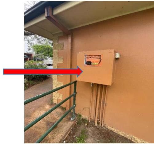
External, GF, Exterior Electrical Box, Backing board - Bituminous, Assumed Positive, No Sample taken Assumed Positive
