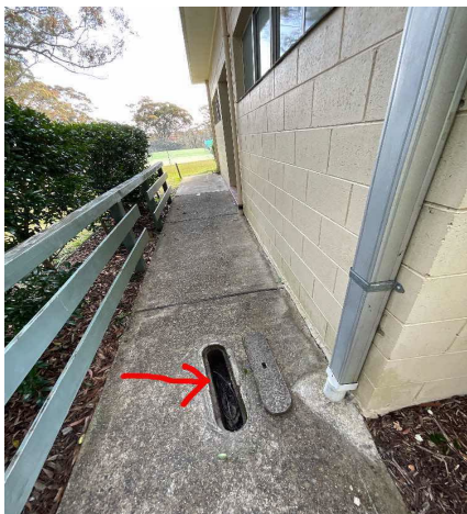
External, GF, Exterior, Sub-surface, Rear access pathway - Telecom pit, Chrysotile Asbestos, 431102/AS02
