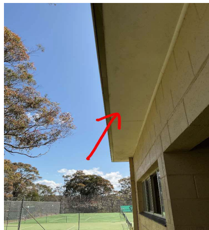
External, GF, Exterior, Eave Linings throughout - Fibreboard, Chrysotile, 28781-50-1
