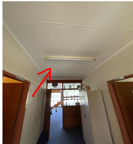
Internal, GF, Rear Entrance, Ceiling Lining - Fibreboard, Assumed Positive, Similar to 28781-50- 4 - Assumed Chrysotile
