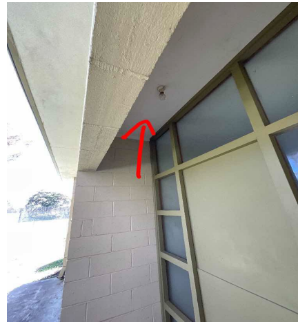
External, GF, Exterior, Rear Entrance Ceiling Lining - Fibreboard, Chrysotile, 28781-50-2
