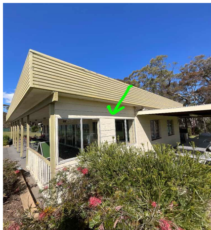
External, GF, Exterior, Canteen Area Partition Wall External Wall Cladding - Fibreboard, No Asbestos identified, 28781-50- 3
