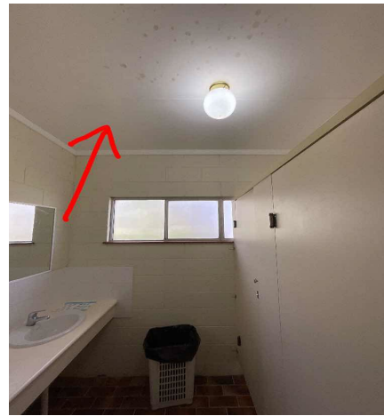
Internal, GF, Female Toilets, Ceiling Lining - Fibreboard, Assumed Positive, Similar to 28781-50-5 - Assumed Chrysotile
