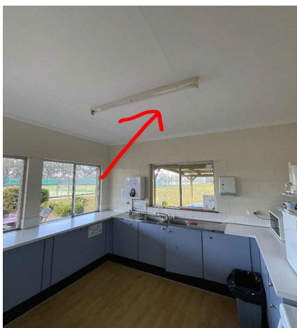
Internal, GF, Kitchen, Ceiling Lining - Fibreboard, Assumed Positive, Similar to 28781-50-4 - Assumed Chrysotile
