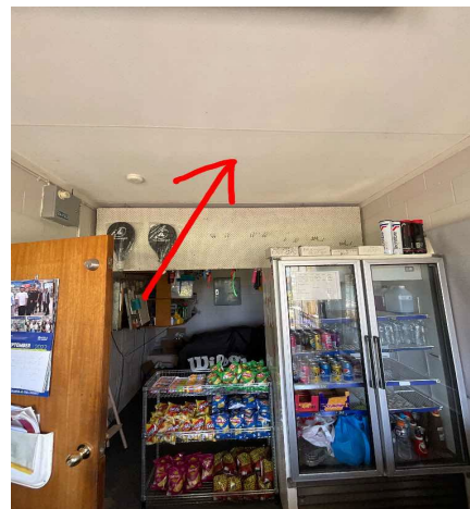
Internal, GF, Canteen/Storeroom, Ceiling Lining - Fibreboard, Assumed Positive, Similar to 28781-50-4 - Assumed Chrysotile
