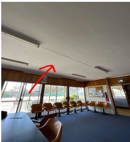
Internal, GF, Clubhouse, Ceiling Lining - Fibreboard, Chrysotile, 28781-50-4
