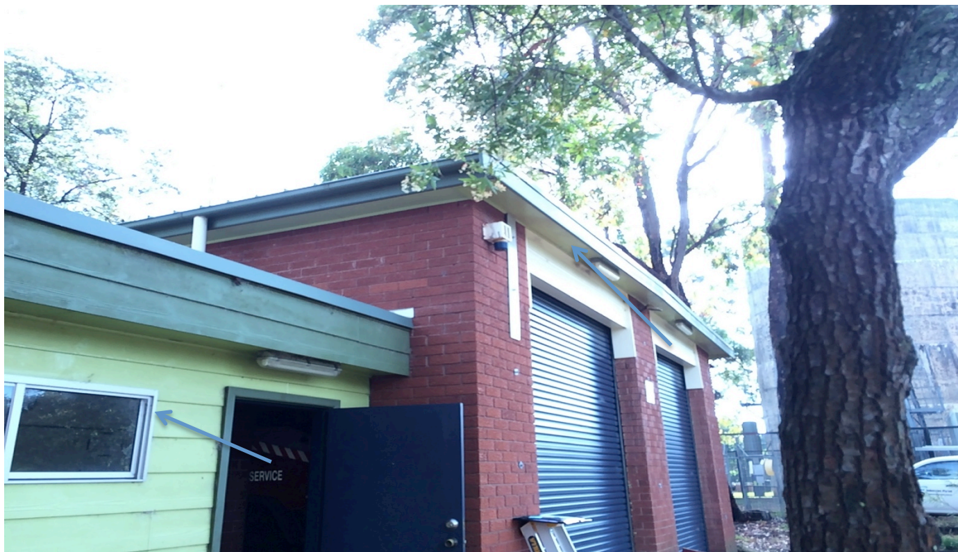
Photo 104: Fibreboard containing asbestos eave linings and external wall cladding of the Glenbrook Rural Fire Service Bushfire Station.
