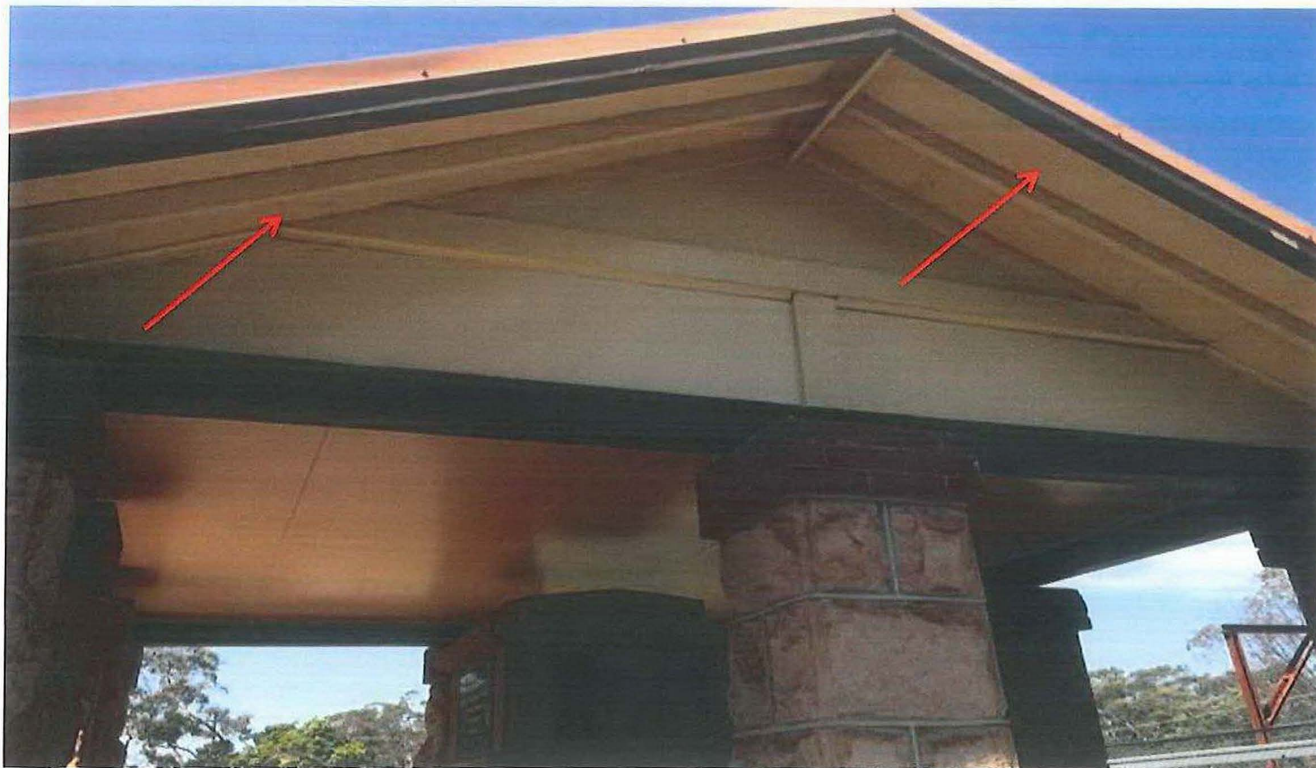
Photo 171: Asset E00189 – Woodford Memorial Shelter – Fibreboard containing asbestos eave linings.
