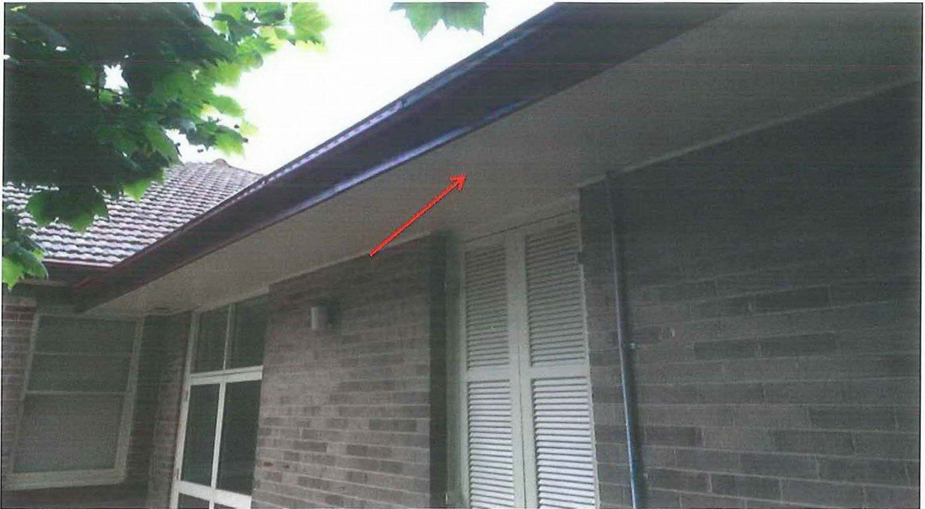
Photo 23: Asset D00081 - Blackheath Hall, Library and Neighbourhood Centre - fibreboard containing asbestos northern perimeter eaves of the KC Bates Hall.
