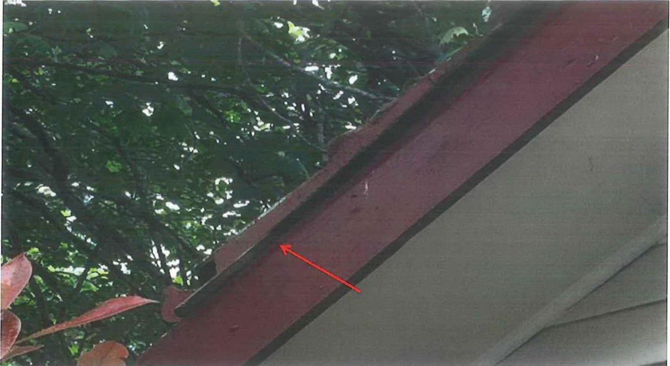
Photo 21: Asset D00081 – Blackheath Hall, Library and Neighbourhood Centre – fibreboard containing asbestos weather strips on the cloaked verges of the roof throughout.
