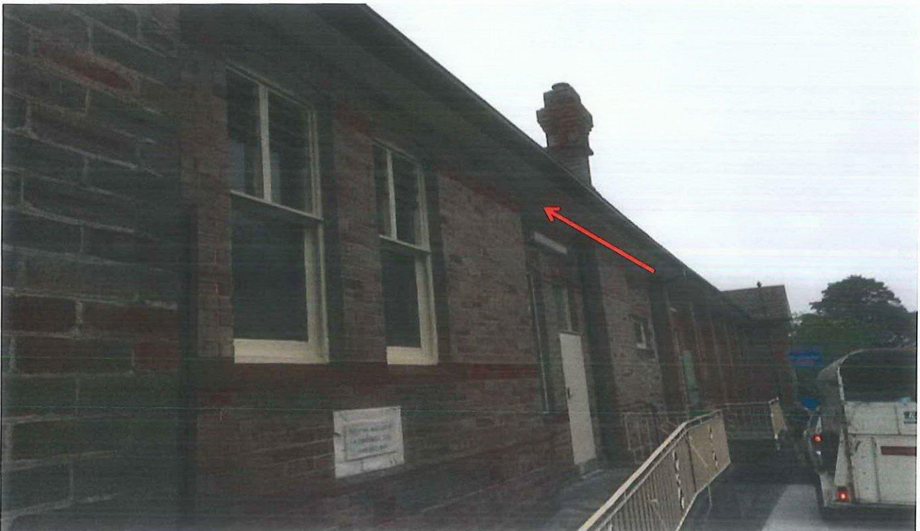
Photo 22: Asset D00081 – Blackheath Hall, Library and Neighbourhood Centre – asbestos cement sheet eave's throughout the Sandy Phillip's Hall.
