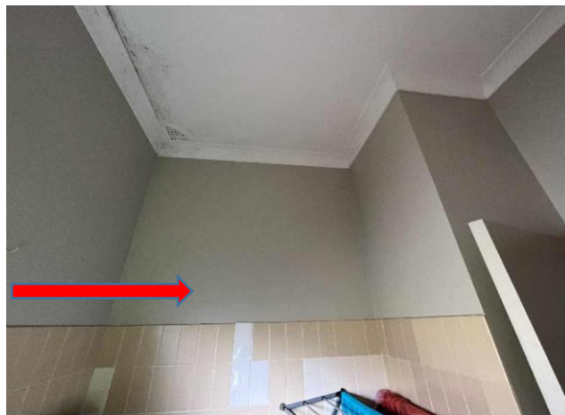
Internal, GF, Bathroom, Wall Cladding - Fibreboard, Chrysotile Asbestos, 28781-4-6
