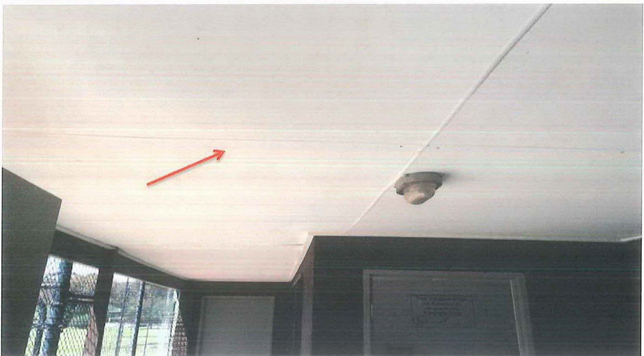
Photo 30: Asset D00149 – Lennox Park, Blaxland – Tennis Clubhouse – fibreboard containing asbestos awning lining.
