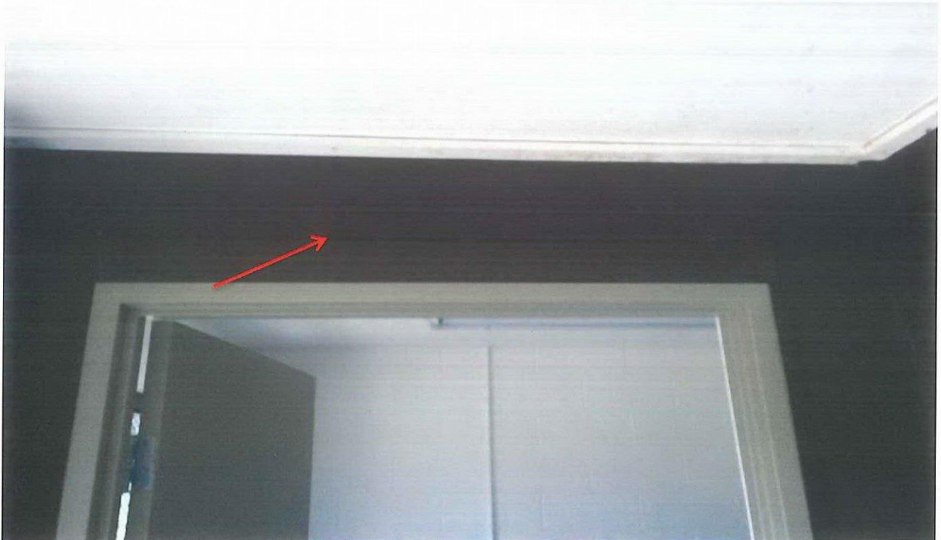
Photo 31: Asset D00149 – Lennox Park, Blaxland – Tennis Clubhouse – fibreglass assumed to contain asbestos above the entrance to the storeroom.
