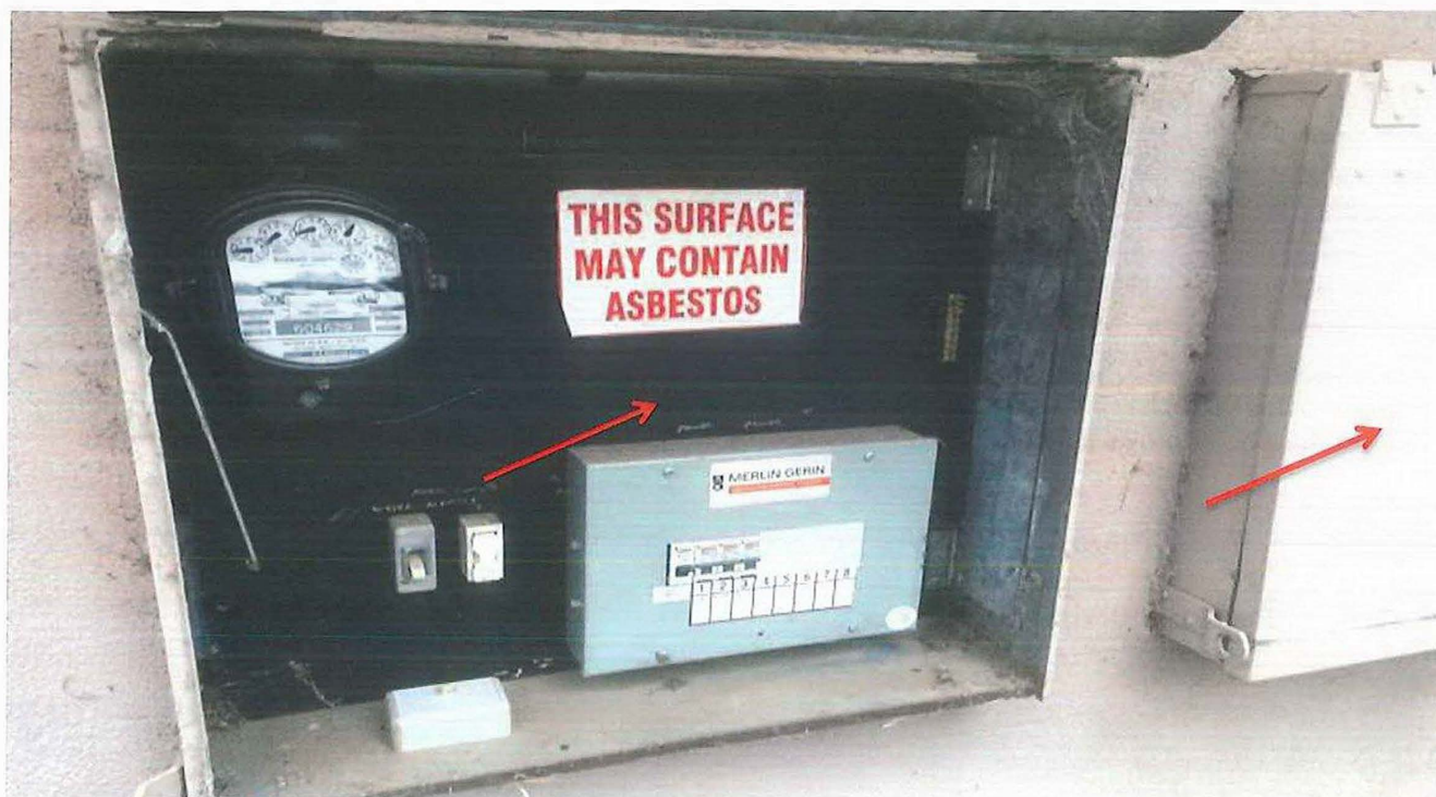
Photo 90: Asset D00097 - Lawson Pool - Canteen and Office - Office - eastern perimeter - electrical backing boards containing asbestos.
