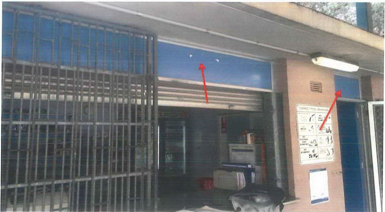
Photo 88: Asset D00097 – Lawson Pool – Canteen and Office – Canteen – asbestos cement sheet infill panels above windows and doorway.
