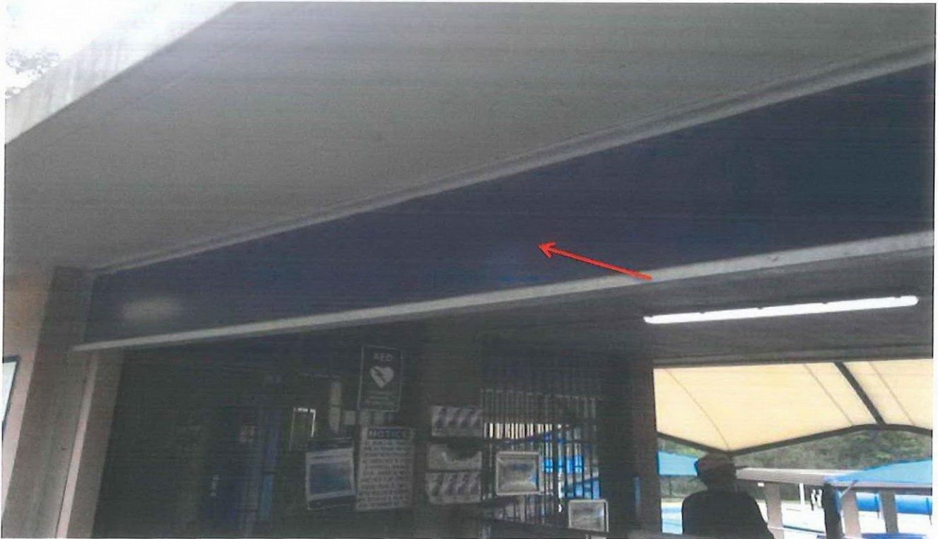
Photo 87: Asset D00097 – Lawson Pool – Canteen and Office – Entrance Area – asbestos cement sheet infill panel above gates.
