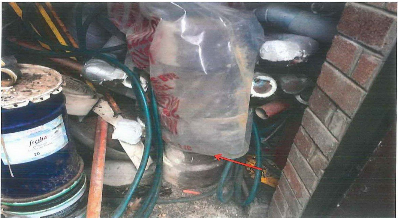
Photo 86: Asset E00515 – Lawson Pool – Change Rooms, Pump and Electrical Rooms and Chemical Stores – asbestos cement conduit with the HV Room.
