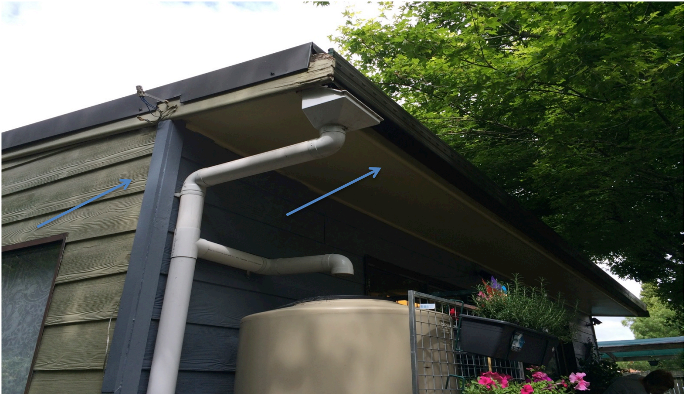
Photo 157: Fibreboard containing asbestos eave lining and external wall cladding of the Nursery area of 156 Megalong Street, Leura.
