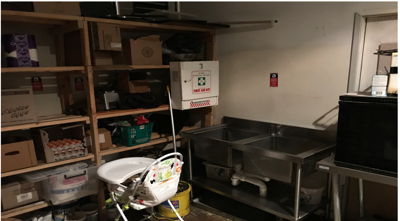
Photo 158: Asbestos cement sheet ceiling internal wall cladding of the café – storeroom of 156 Megalong Street, Leura.
