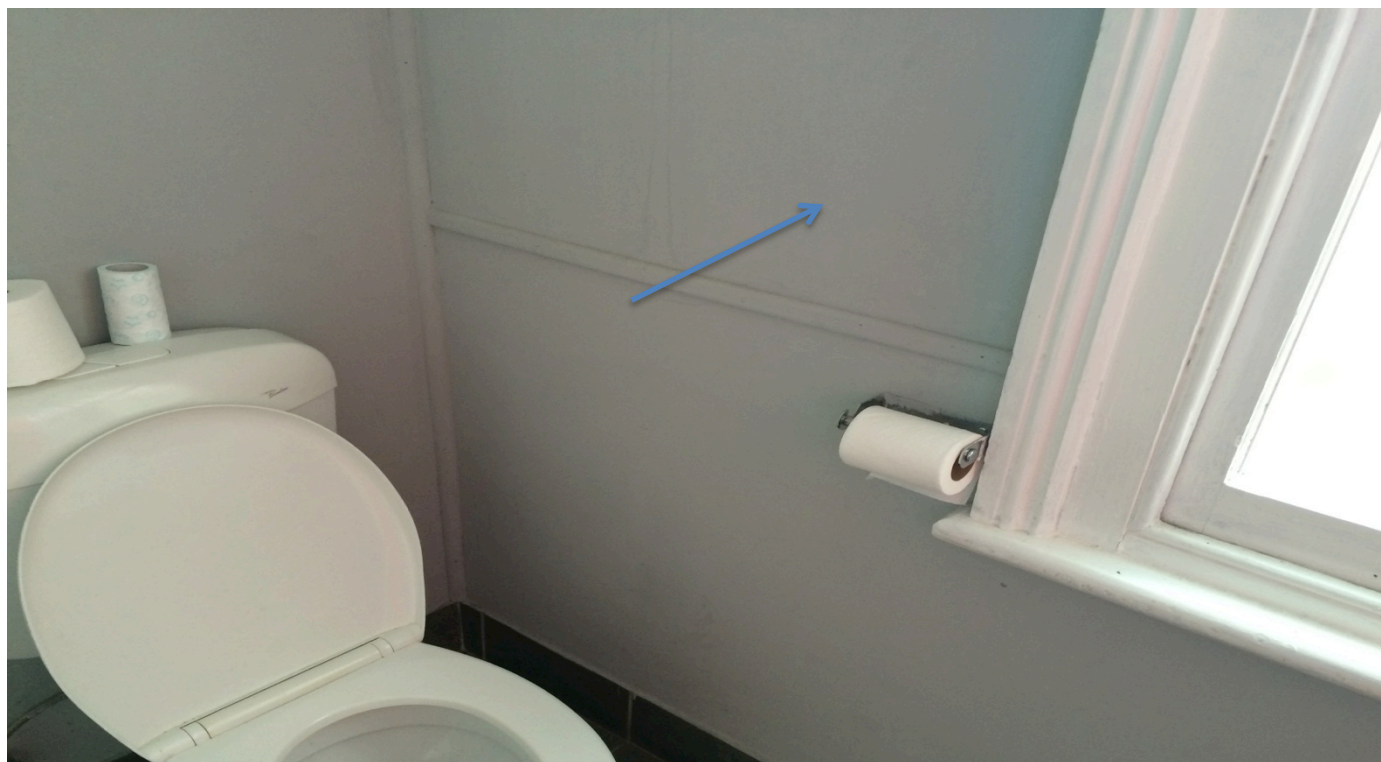
Photo 159: Asbestos cement sheet northern internal wall cladding of the Customer Toilet in the Cafe area of 156 Megalong Street, Leura.
