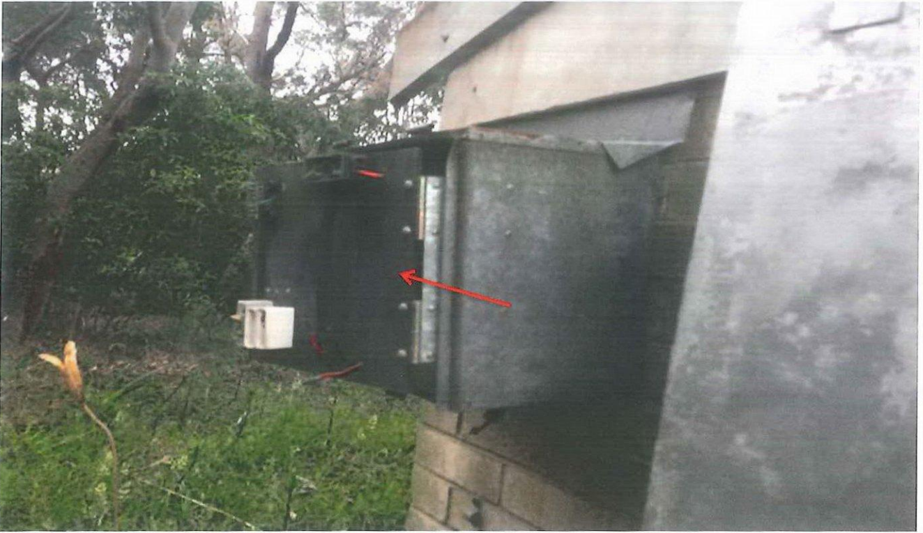
Photo 101: Asset E00017 – Former Lawson Golf Course – Machinery Shed – Western Perimeter – electrical backing board containing asbestos.
