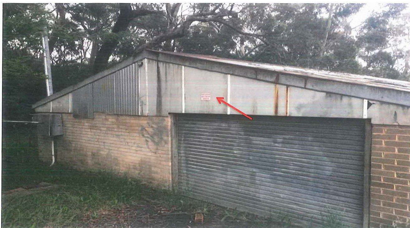
Photo 100: Asset E00017 – Former Lawson Golf Course – Machinery Shed – Western Perimeter – fibreboard containing asbestos gable end.
