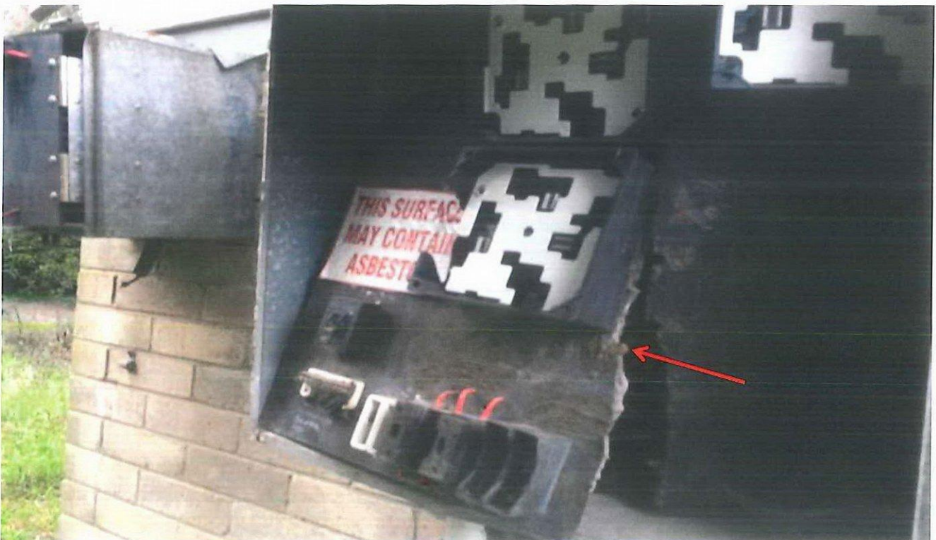
Photo 102: Asset E00017 – Former Lawson Golf Course – Machinery Shed – Western Perimeter – broken electrical backing board containing asbestos.
