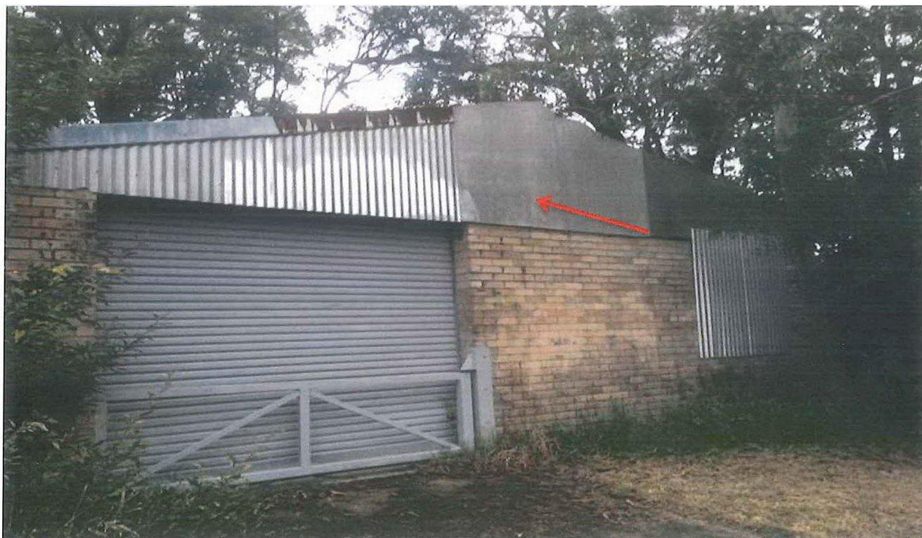
Photo 103: Asset E00017 – Former Lawson Golf Course – Machinery Shed – Eastern Perimeter – fibreglass containing asbestos sheeting is present behind the timber and tin gable end.
