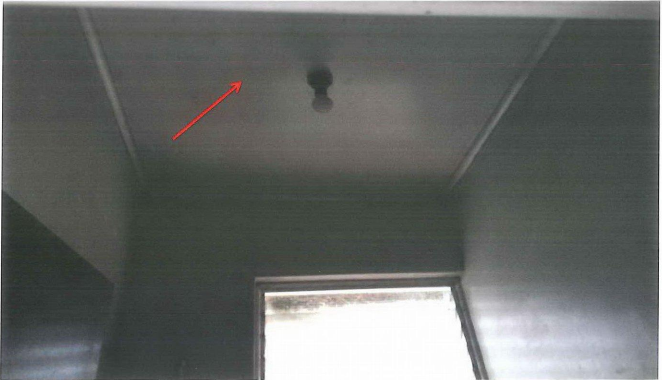
Photo 113: Asset D00151 – The Elise Langford Centre, Medlow Bath – asbestos cement sheet ceiling lining of toilet #1 (north).
