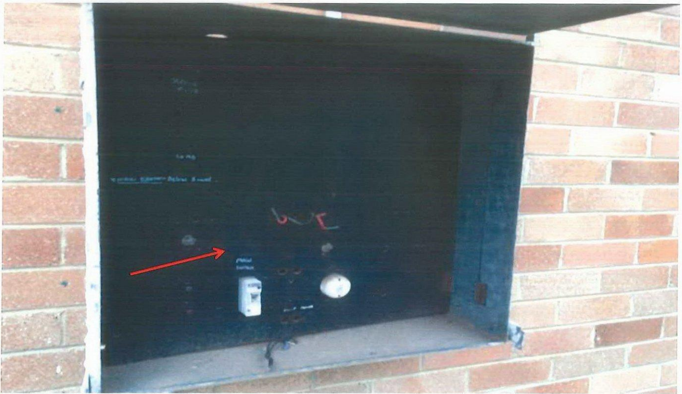
Photo 111: Asset D00151 – The Elise Langford Centre, Medlow Bath – electrical backing board containing asbestos on the western perimeter.
