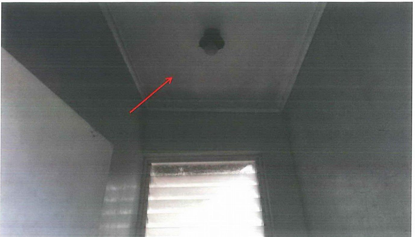
Photo 114: Asset D00151 – The Elise Langford Centre, Medlow Bath – asbestos cement sheet ceiling lining of toilet #2 (south).
