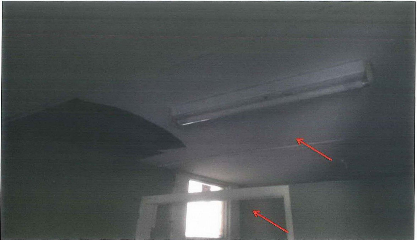
Photo 99: Asset D00040 – Former Lawson Golf Course – Clubhouse – Lower Level Change Rooms – Southern Toilet – asbestos cement sheet ceiling lining and upper internal wall cladding.
