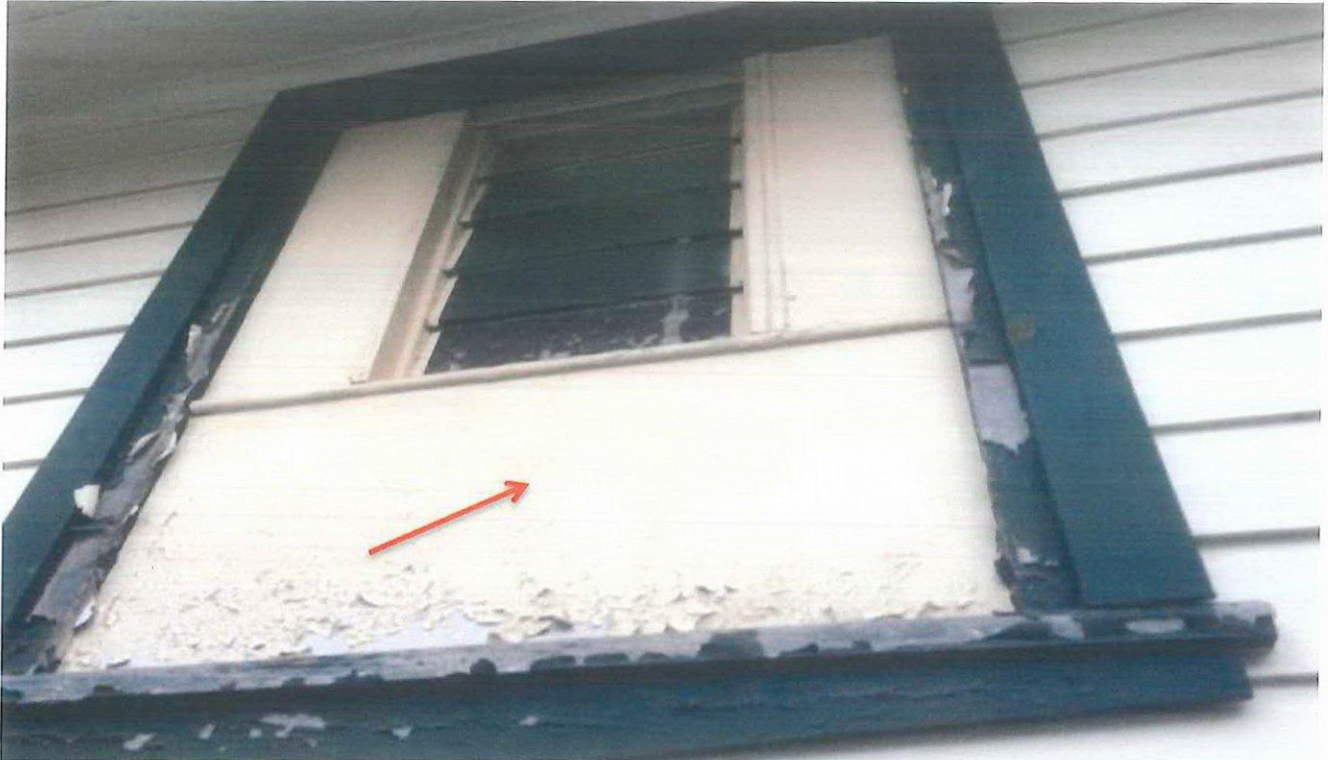
Photo 91: Asset D00040 – Former Lawson Golf Course – Clubhouse – Male Toilets – asbestos cement sheet infill panel around eastern window.
