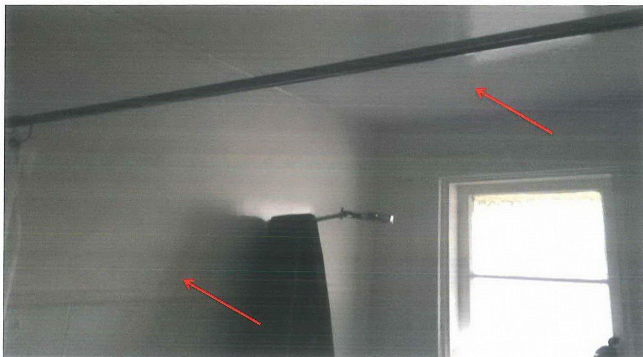
Photo 98: Asset D00040 – Former Lawson Golf Course – Clubhouse – Male Change Rooms – Shower Area – asbestos cement sheet ceiling lining and internal wall cladding.
