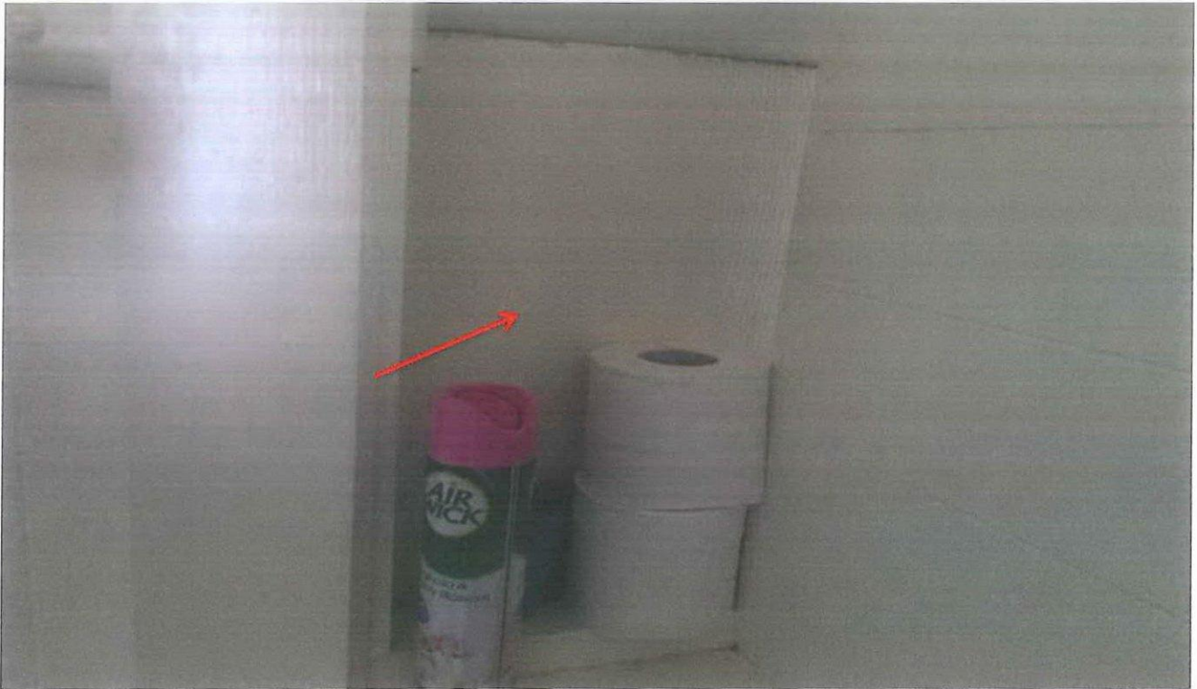
Photo 95: Asset D00040 – Former Lawson Golf Course – Clubhouse – Female Change Rooms – asbestos cement sheet infill panel in the western window.
