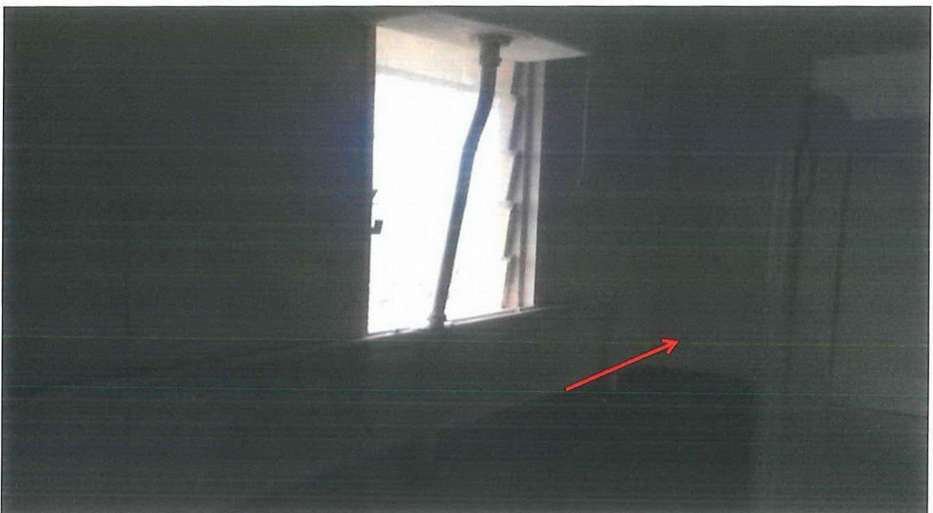
Photo 96: Asset D00040 – Former Lawson Golf Course – Clubhouse – Male Change Rooms – toilet area – asbestos cement sheet internal wall cladding.
