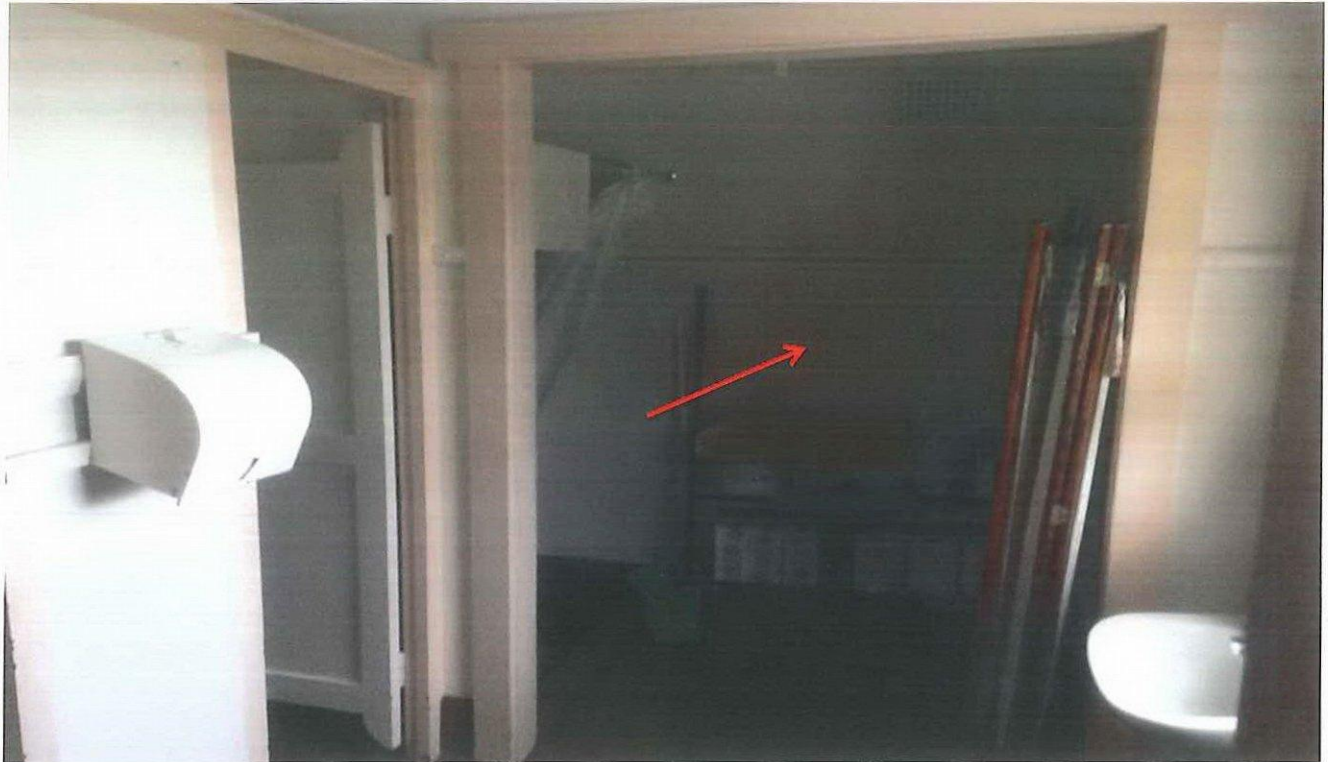
Photo 93: Asset D00040 – Former Lawson Golf Course – Clubhouse – Female Change Rooms – asbestos cement sheet lower internal wall cladding.
