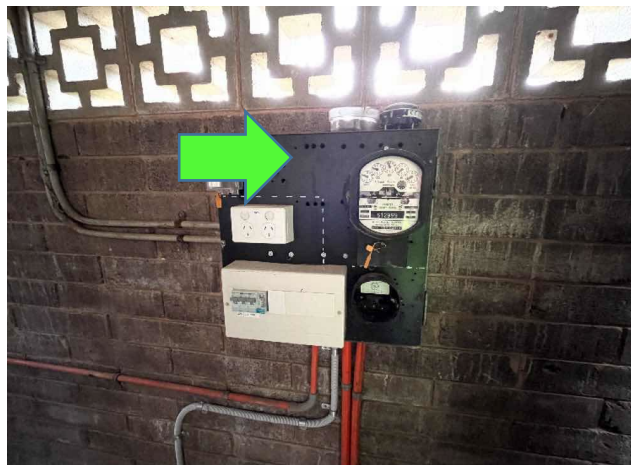
Internal, GF, Cistern Room, Internal southern wall - Electrical backing board, None Suspected, N/A
