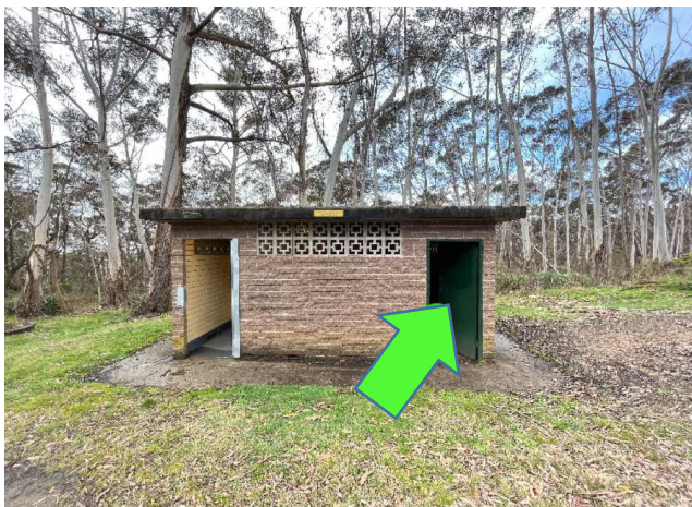
Internal, GF, Cistern Room, Door and door frame - Green paint, 433800/LP01
