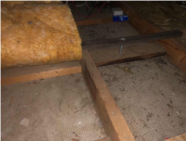
197612A2.1 Flat cement sheets Internal GF Roof Space Panels forming ceiling to kitchen and bathroom below
