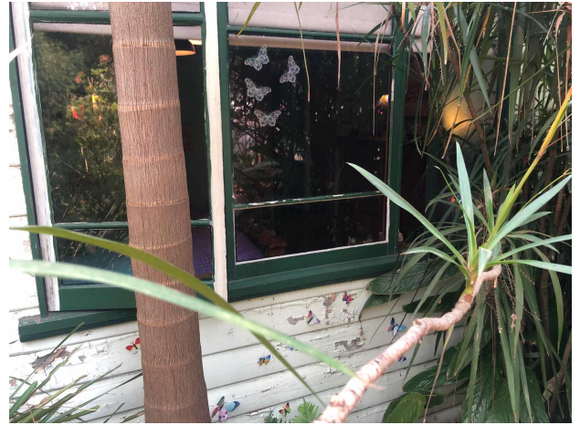
197612A7 Putty External GF All Elevations Window frames
