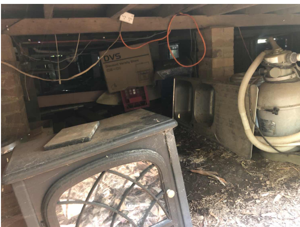
197612La1 Internal Sub-Floor Undercroft Undercroft
