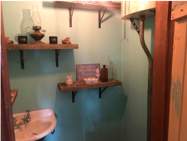
197612A4.1 Flat cement sheets External GF Toilet Wall panels behind plasterboard
