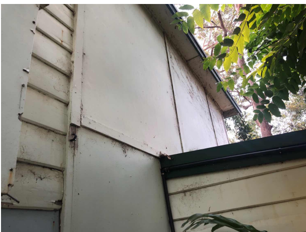
197612A5.4 Flat cement sheets External GF South Elevation Wall panels
