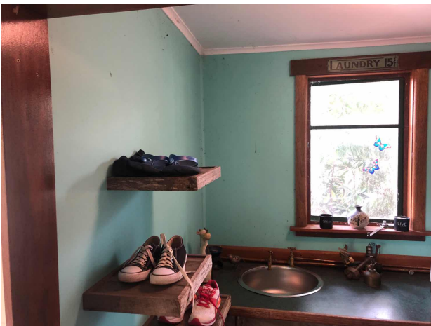
197612A4 Flat cement sheets External GF Laundry Wall panels behind plasterboard
