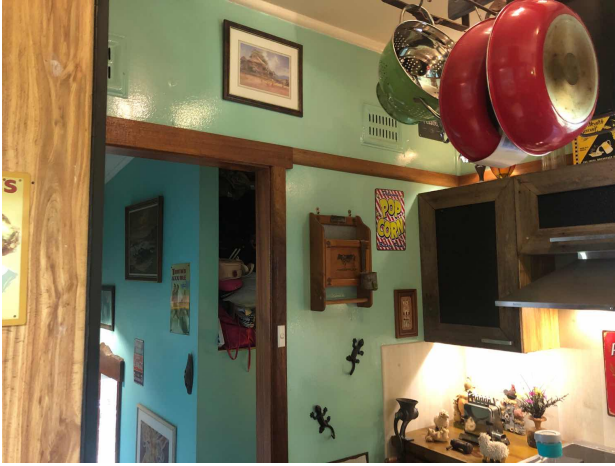
197612A1 Flat cement sheets Internal GF Kitchen Wall panels
