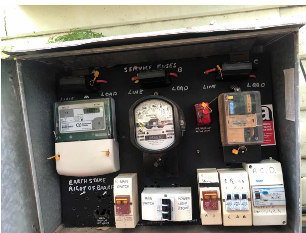
197612A6 Compressed bitumen External GF South Elevation Electrical mounting board
