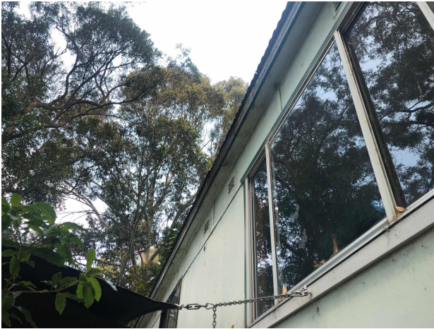
197612A5 Flat cement sheets External GF East Elevation Eaves
