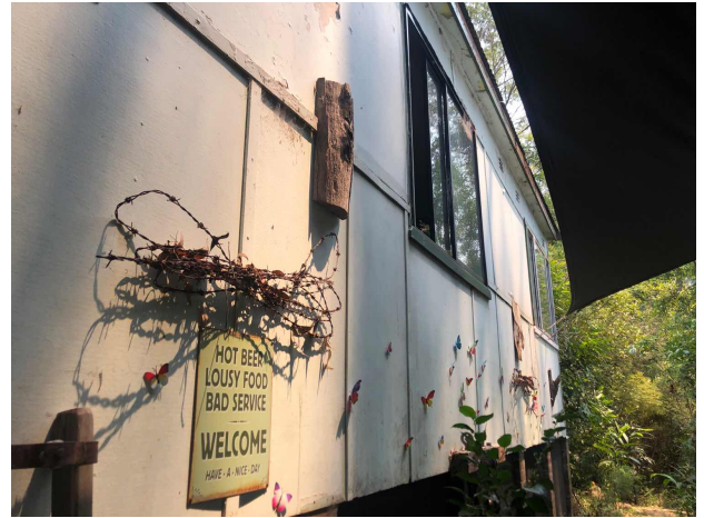
197612A5.1 Flat cement sheets External GF East Elevation Wall panels
