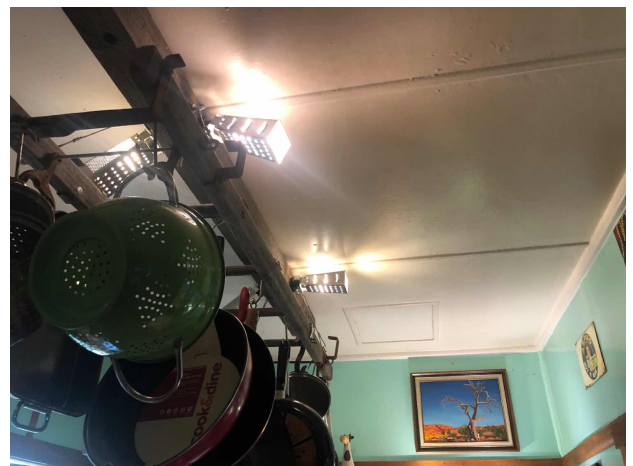
197612A2 Flat cement sheets Internal GF Kitchen Ceiling panels
