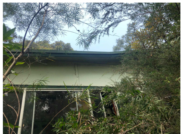
197612A5.3 Flat cement sheets External GF North Elevation Eaves
