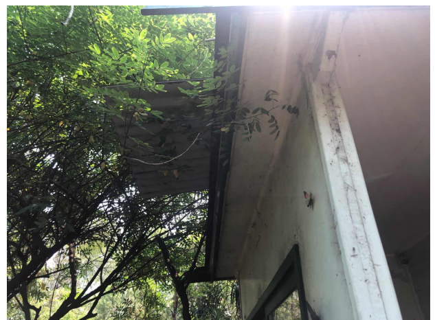
197612A5.7 Flat cement sheets External GF West Elevation Eaves
