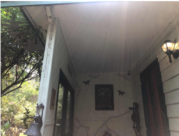
197612A5.6 Flat cement sheets External GF West Elevation Wall and ceiling panels to front porch
