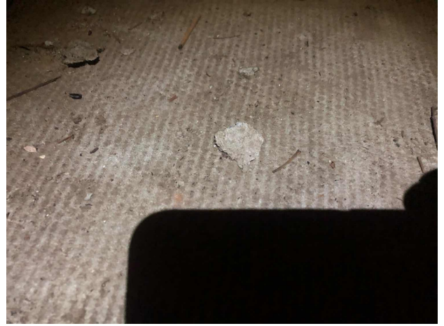
197612A3 Cement debris Internal GF Roof Space Adjacent manhole
