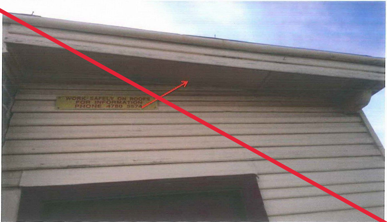
Photo 1: Asset D00153 – Jubilee Park, Blackheath – Tennis Clubhouse – western perimeter – fibreboard eave lining containing asbestos.
