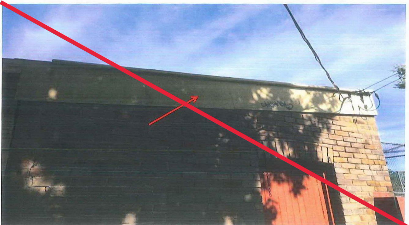
Photo 2: Asset D00153 – Jubilee Park, Blackheath – Tennis Clubhouse – eastern/western perimeter's – asbestos cement sheet flashing.
