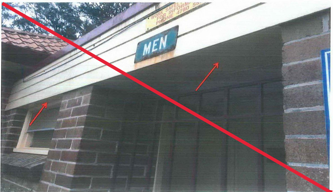
Photo 10: Asset E00544 – Blackheath Pool – Amenities Block – asbestos cement sheet eave linings and panels above the windows of the Male Changerooms and Toilets.
