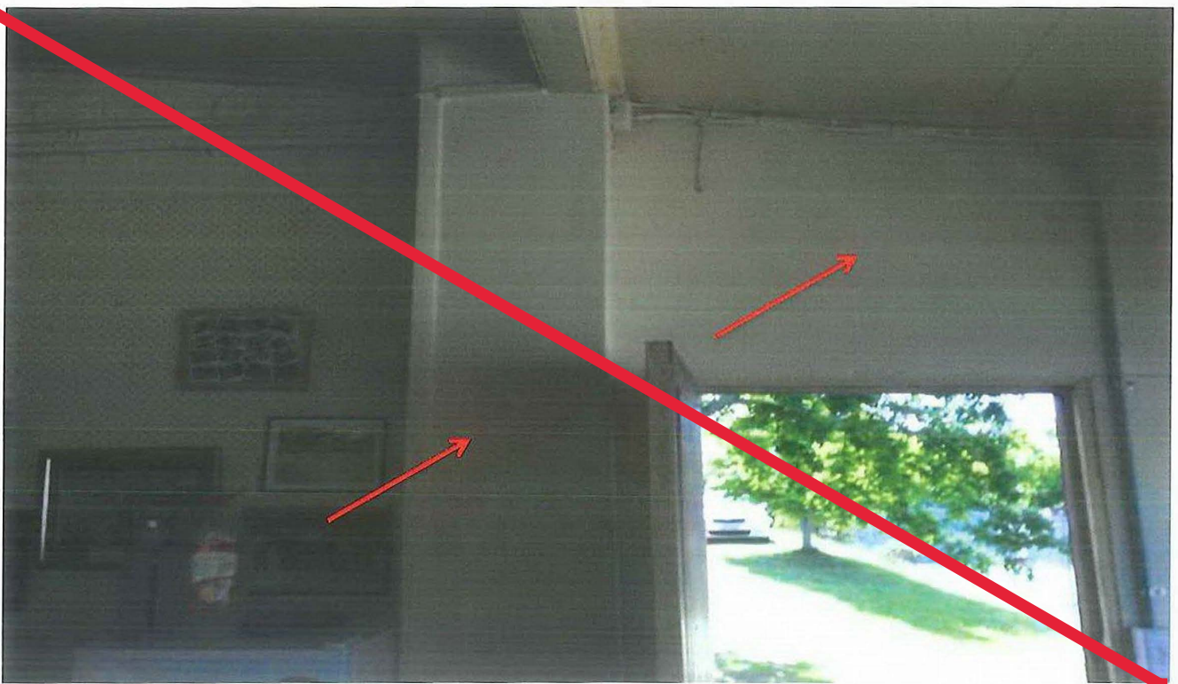
Photo 8: Asset D00153 – Jubilee Park, Blackheath – Tennis Clubhouse – kitchen and eastern entrance doorway – fibreboard containing asbestos riser covering and internal wall.
