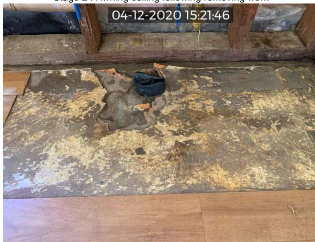
Stage 4 : Potential asbestos final below modern vinyl and tiles throughout
