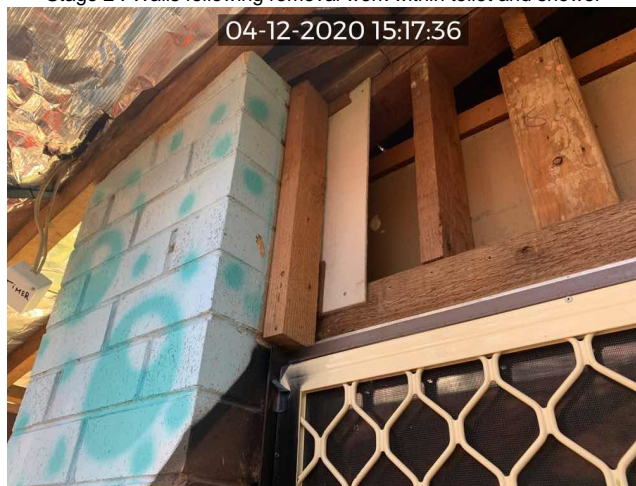
Stage 4 : Trapped asbestos cement still remains to the north-west corner eaves
