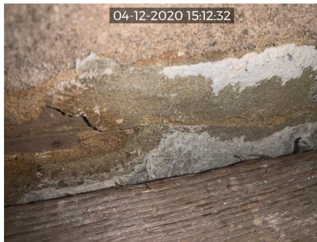
Stage 2 : Asbestos cement to back side of bathroom plinth
