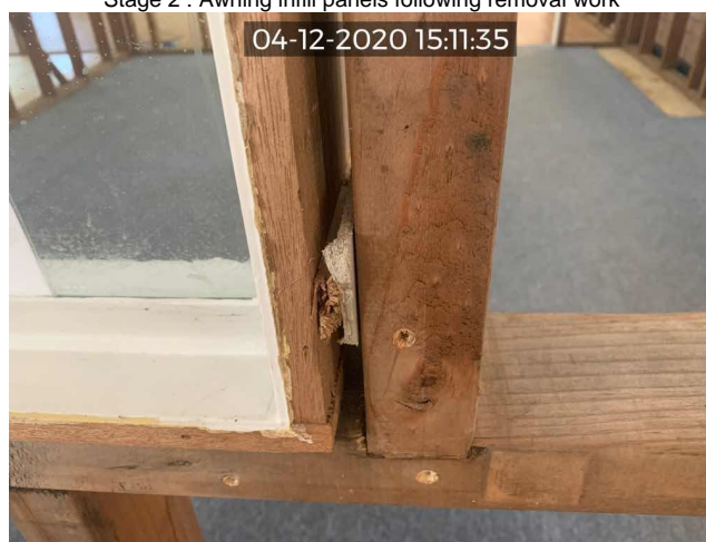
Stage 2 : Example of Packers between all windows
