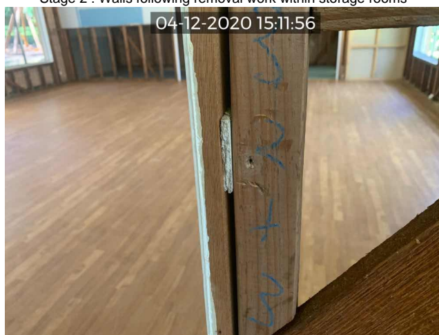
Stage 2 : Example of Packers to all doors
