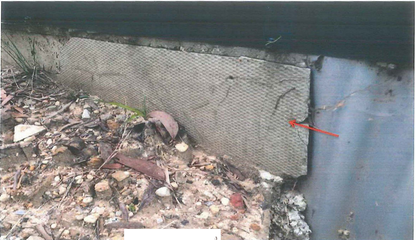
Photo 85: Asset D00099 – Trotting Pavilion – Katoomba Men's Shed– Garage Area asbestos cement sheeting on the eastern perimeter of the concrete slab.
