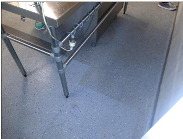
Plate 5: Kitchen floor, next to floating bench
