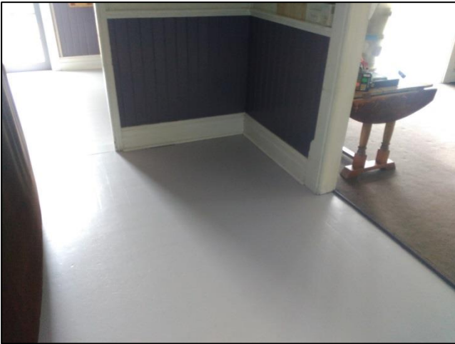
Plate 1: Reception room floor beneath replaced panel
