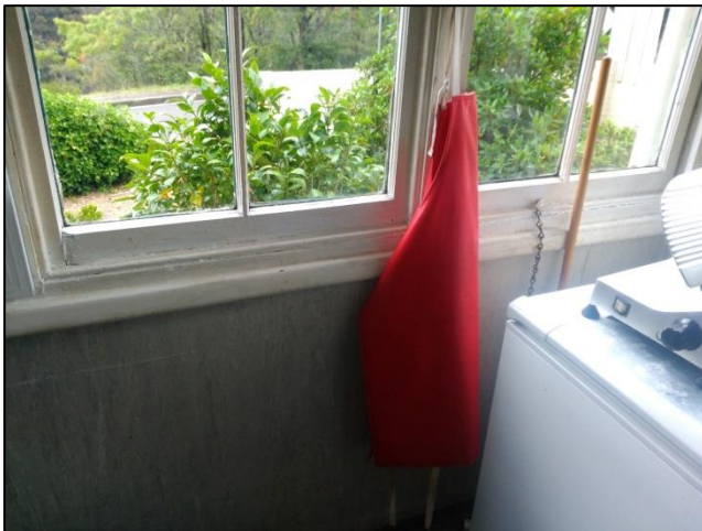
Plate 6: Windowsill, west end of kitchen
