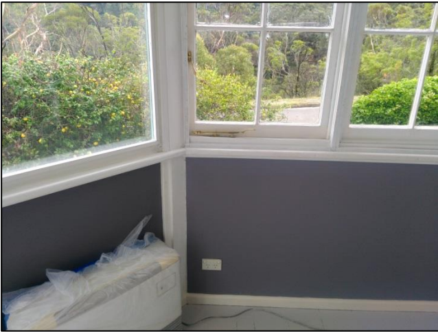
Plate 3: Windowsill, south corner of dining room
