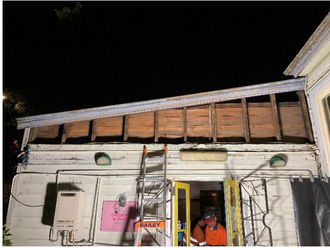
Photograph 7: Work area following removal works.
