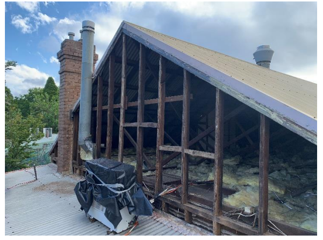
Photograph 8: Work area following removal works.
