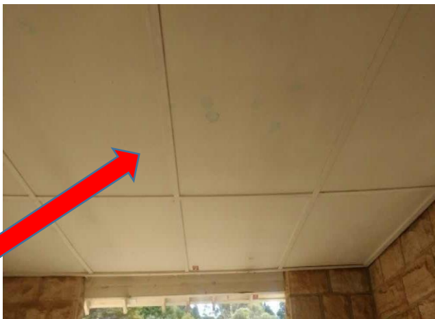
External, GF, Exterior, Ceiling Lining - Fibre cement sheet, Chrysotile Asbestos, Previously sampled 21880-106
