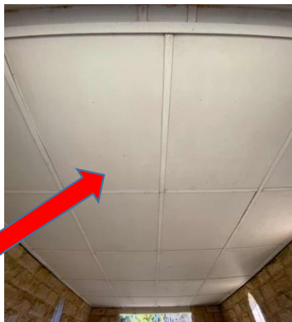
External, GF, Exterior, Ceiling Lining - Fibre cement sheet, Chrysotile Asbestos, Previously sampled 21880-106
