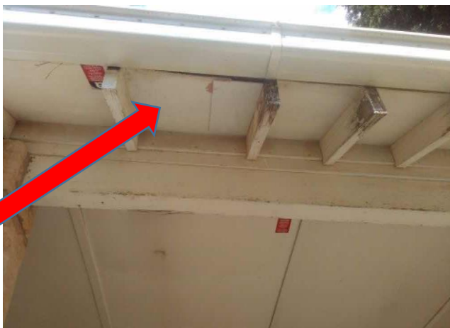
External, GF, Exterior, Western Perimeter Eave Linings - Fibre cement sheet, Chrysotile Asbestos, Previously sampled 21810-106
