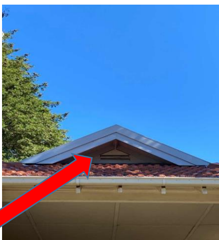
External, GF, Exterior, Western/Eastern Gable Ends - Fibre cement sheet, Assumed Positive chrysotile asbestos, Similar to 21812-106
