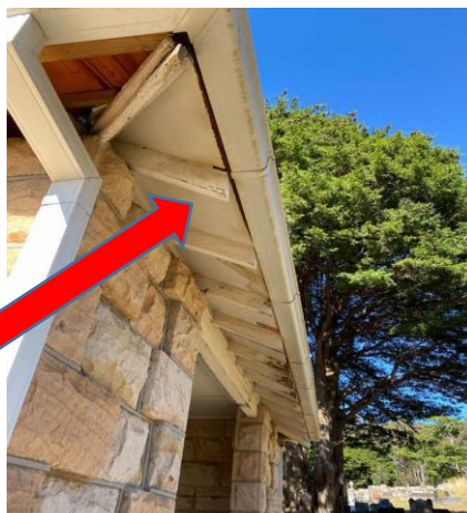
External, GF, Exterior, Western Perimeter Eave Linings - Fibre cement sheet, Chrysotile Asbestos, Previously sampled 21810-106
